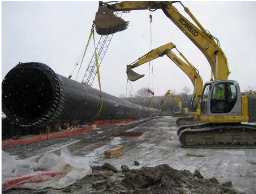
View of HDPE being placed in the trench.
