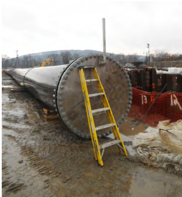
View of air vent on blind flange.
