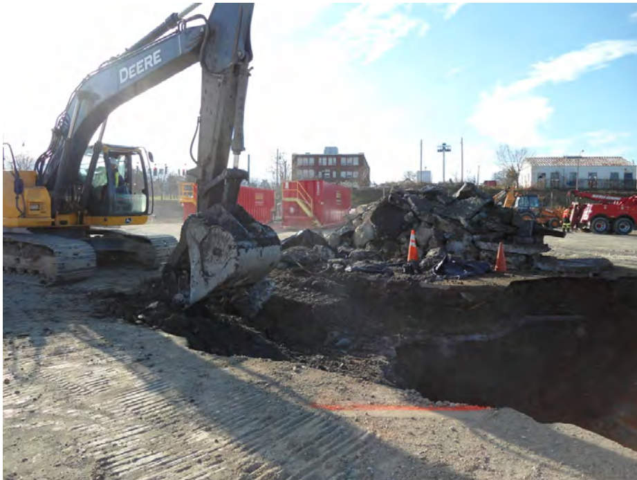
Excavation over the No. 4 Gas Holder foundation facing southwest.
