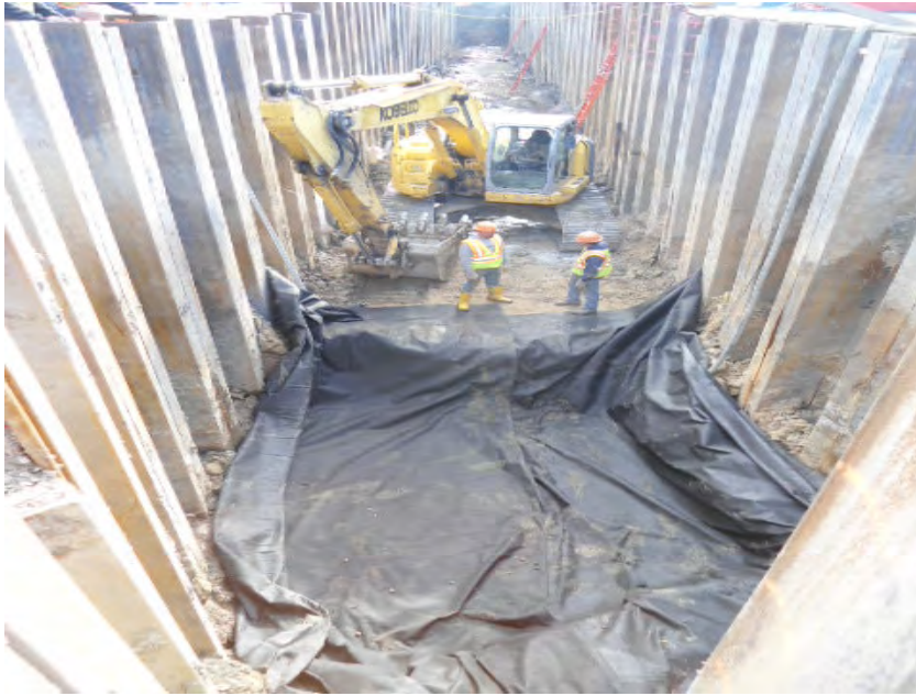
Tioga and AECOM placing geo-textile fabric over MH1-C excavation. Photo taken from north end of site facing south.
