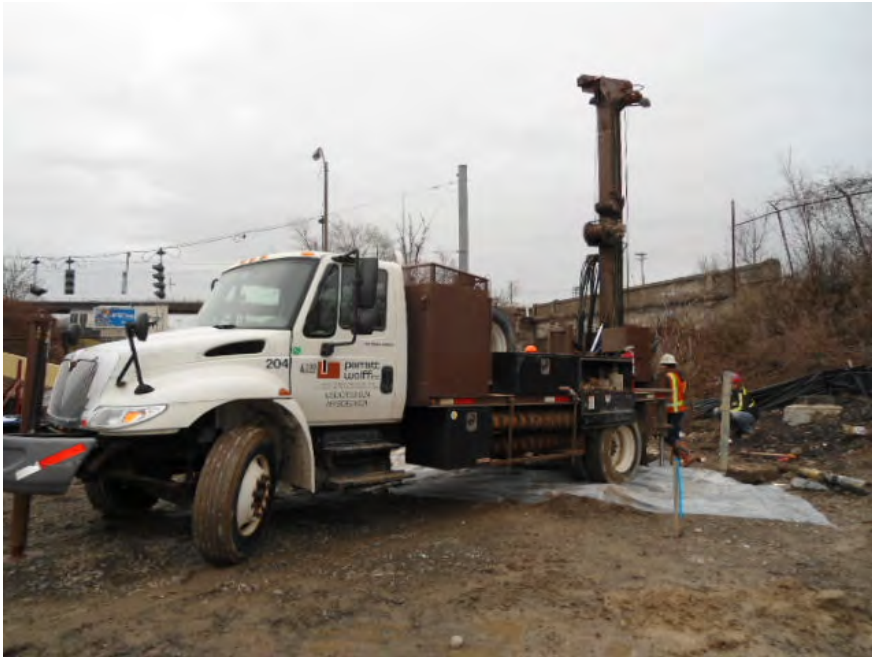
Parratt Wolff and ARCADIS decommissioning wells at north end of the site. Photo taken at north end, facing northwest.
