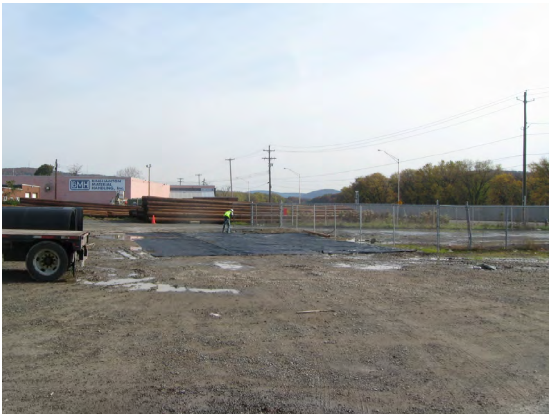
Constructing stabilized construction entrance
