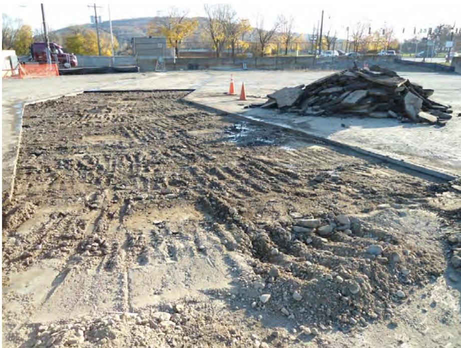
Trench alignment following asphalt demolition
