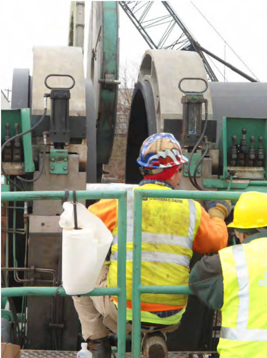
Vari-Tech setting up the south flange and an approximately 54-foot pipe section for surface ‘trimming’ (facing west).
