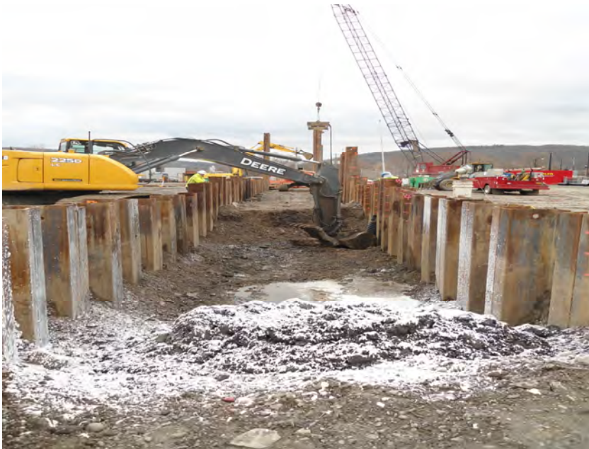
Installation of sump at leaking sheet along west alignment (facing southwest)
