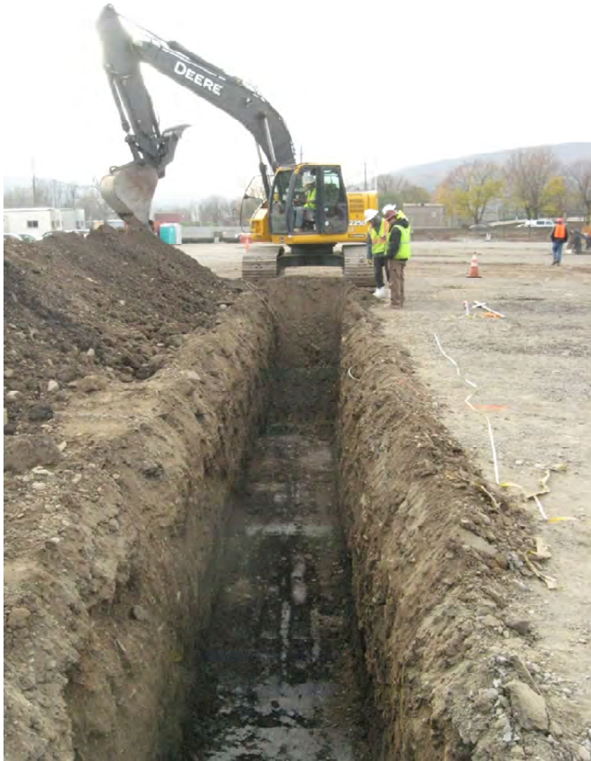
AECOM performing pre-trenching along the east sheeting alignment
