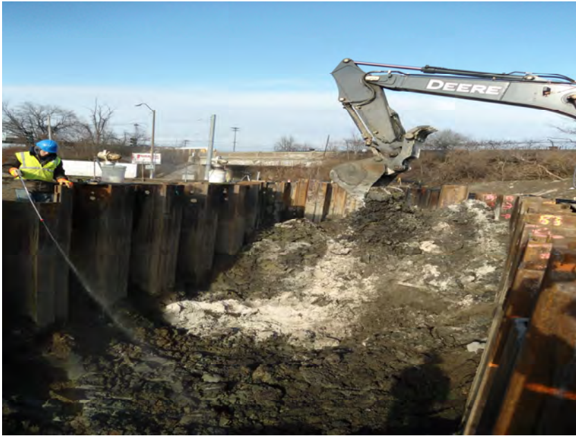
Performing trench excavation and dewatering with CKD (facing north)
