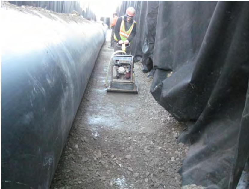
View of compaction alongside the HDPE pipe. Geotextile fabric is visible on the side of the trench.
