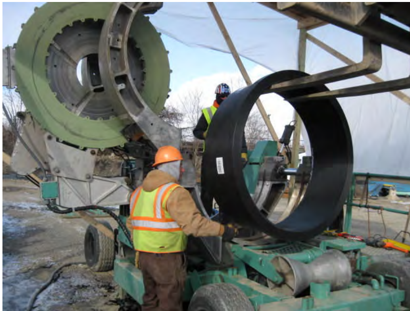
View of Vari-Tech welding a flange on the HDPE.
