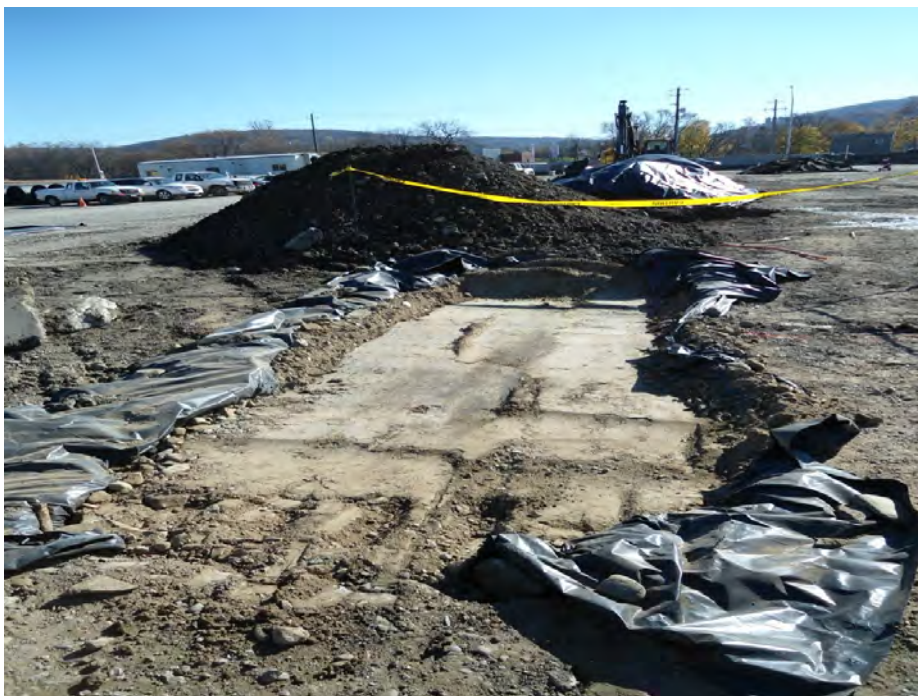
Lined excavation areas backfilled with non-visually impacted material
