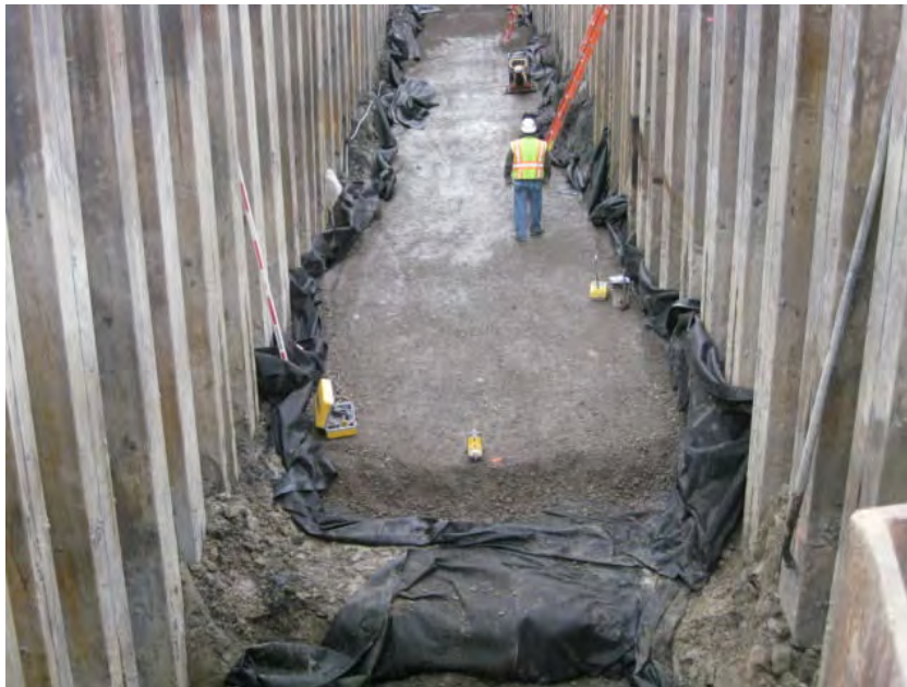
View of compaction testing on the crushed stone.
