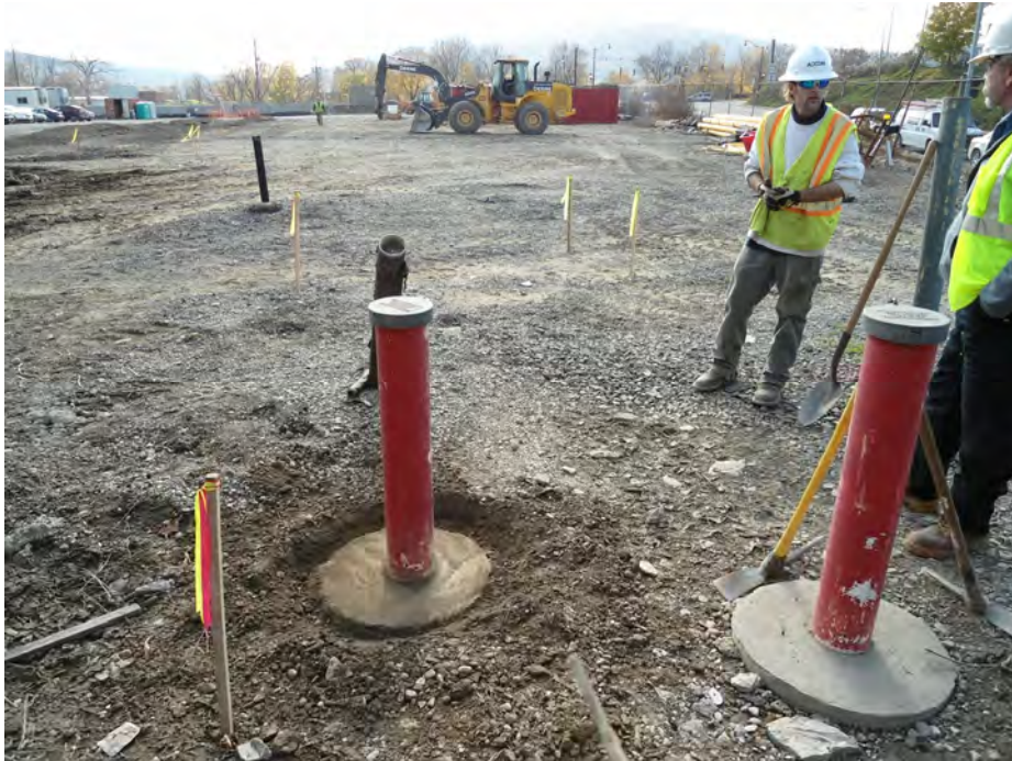
West trench alignment stake adjacent to monitoring wells MW93-6S (left), MW93-6D (right), and piezometer PZ01-05 (background)
