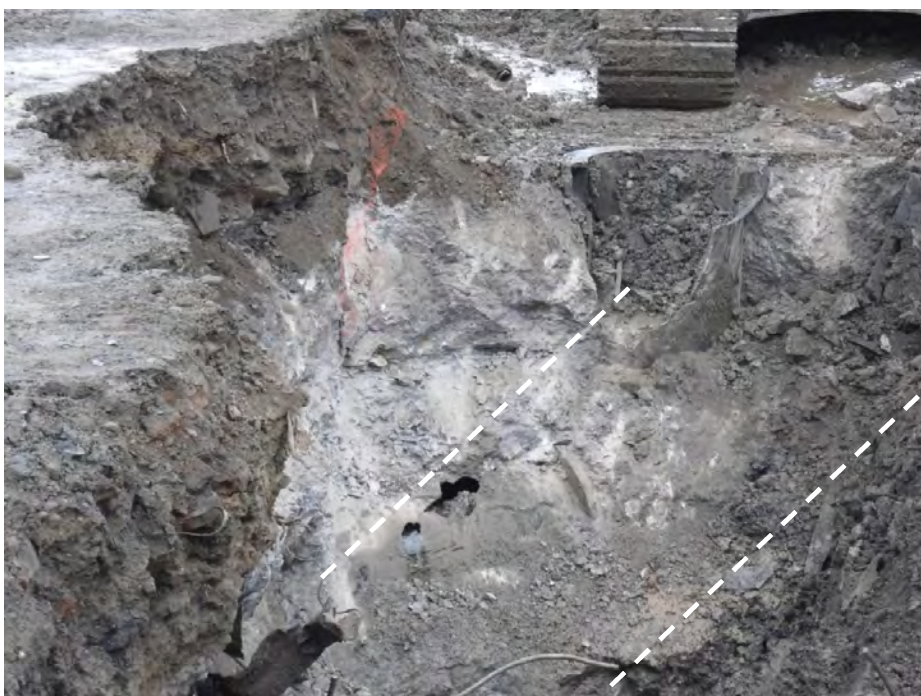
30" diameter cast iron pipe, embedded in concrete with visible coal tar product present
