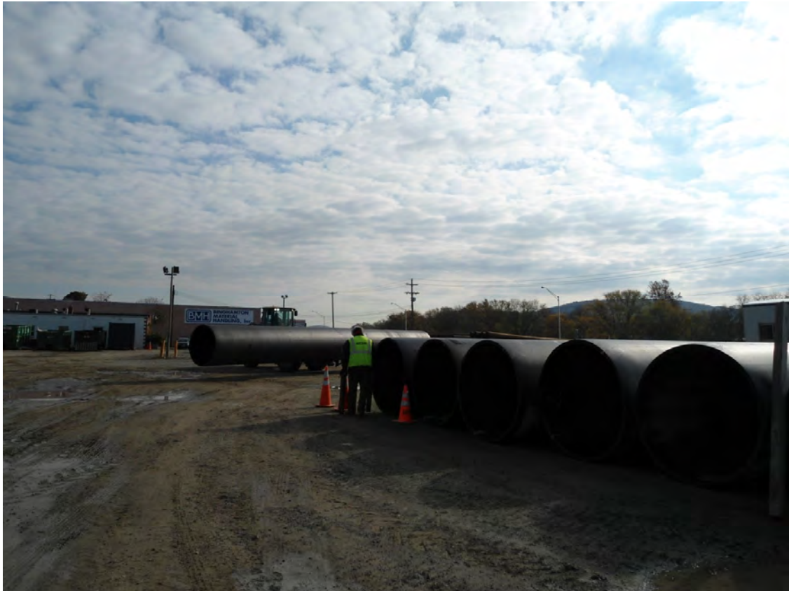
Relocating and stockpiling HDPE pipe
