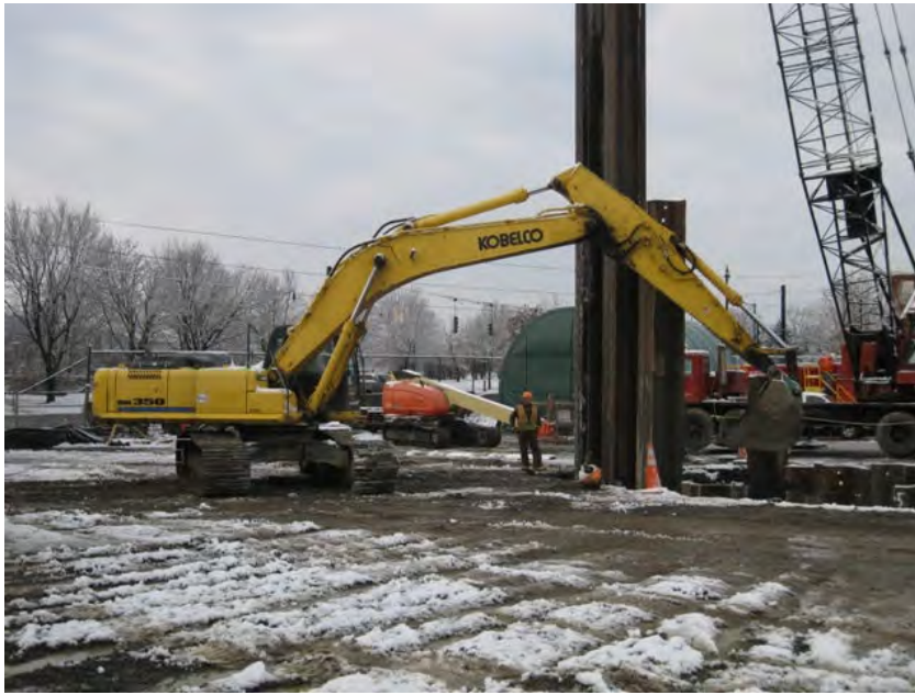
Tioga installing sheets at southern end of site. Photo facing south west.
