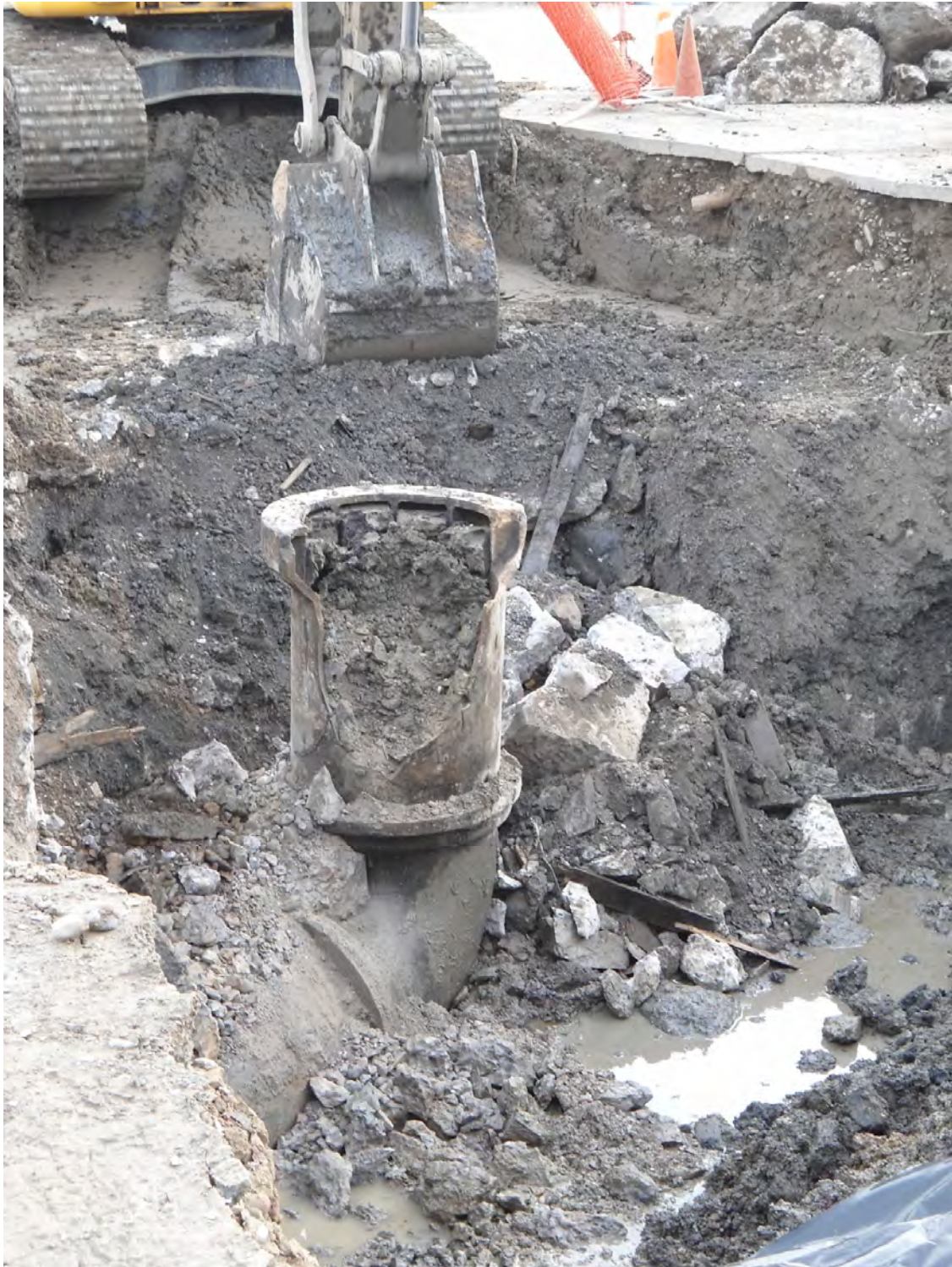
30" diameter cast iron pipe, exposed 90 degree section
