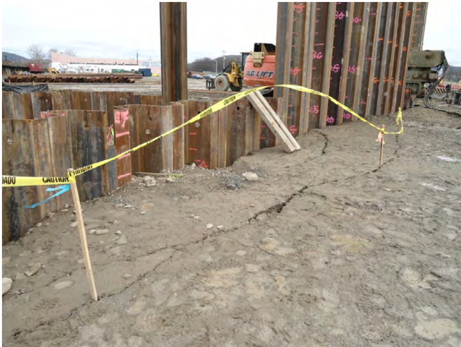
Compaction and cracking along the west sheeting alignment
