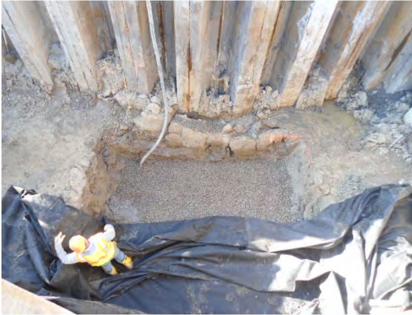
Tioga placing geo-textile over #1 and #2 stone excavation for MH-1C. Photo taken at north end of site from east side of sheet wall.
