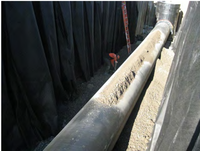
View of temporary connection at MH-1C (to secure HDPE for backfill until new rings arrived onsite)
