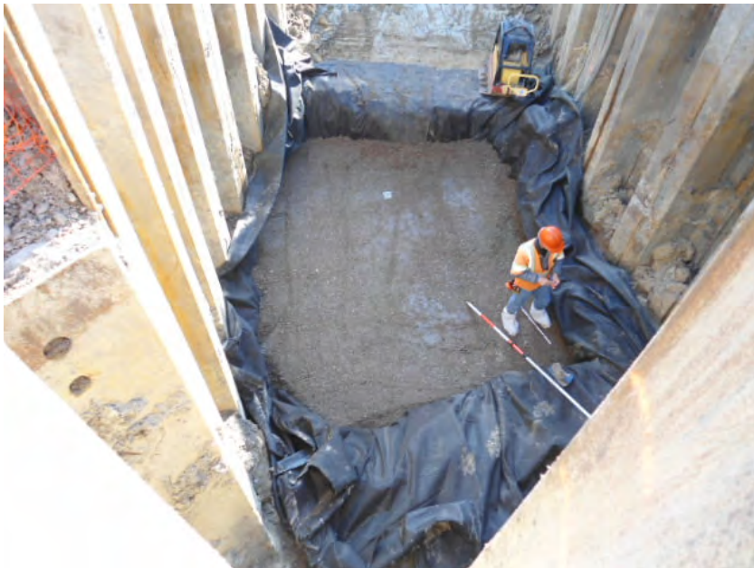
Keystone associates surveying corners of MH-1C alignment. "F" type stone placed over geo-textile fabric and compaction completed. Photo taken from north end of site.
