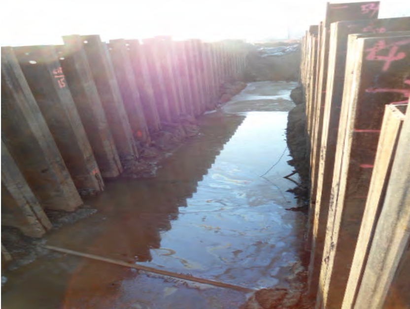
View of trench looking south, following initial dewatering efforts at start of day.
