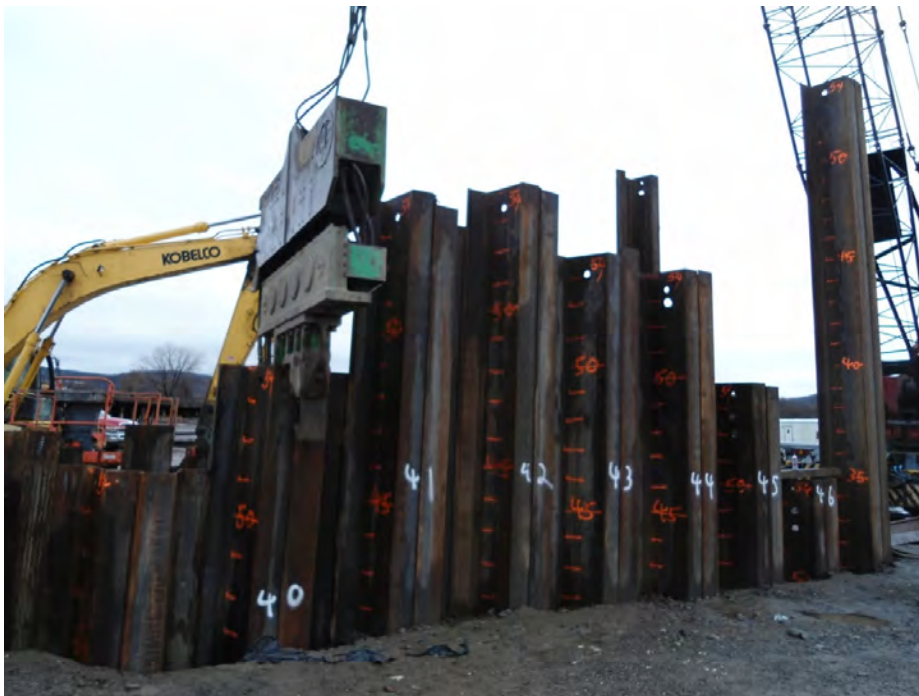
Area of problematic sheets along the west sheeting alignment. Photo was taking from the west looking left at the exterior of the sheet wall.
