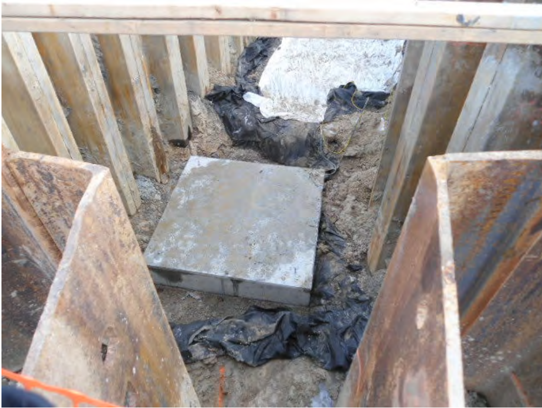
The footer cleared by Tioga Construction for the northern manhole (facing southeast).
