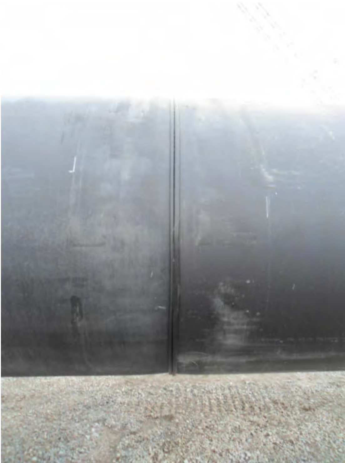
A successful butt-fusion of HDPE sections two and three (facing west).
