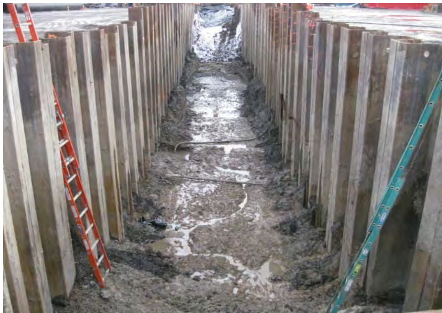
View of excavation showing water from leaks. Photo taken from north end of excavation facing down and south.
