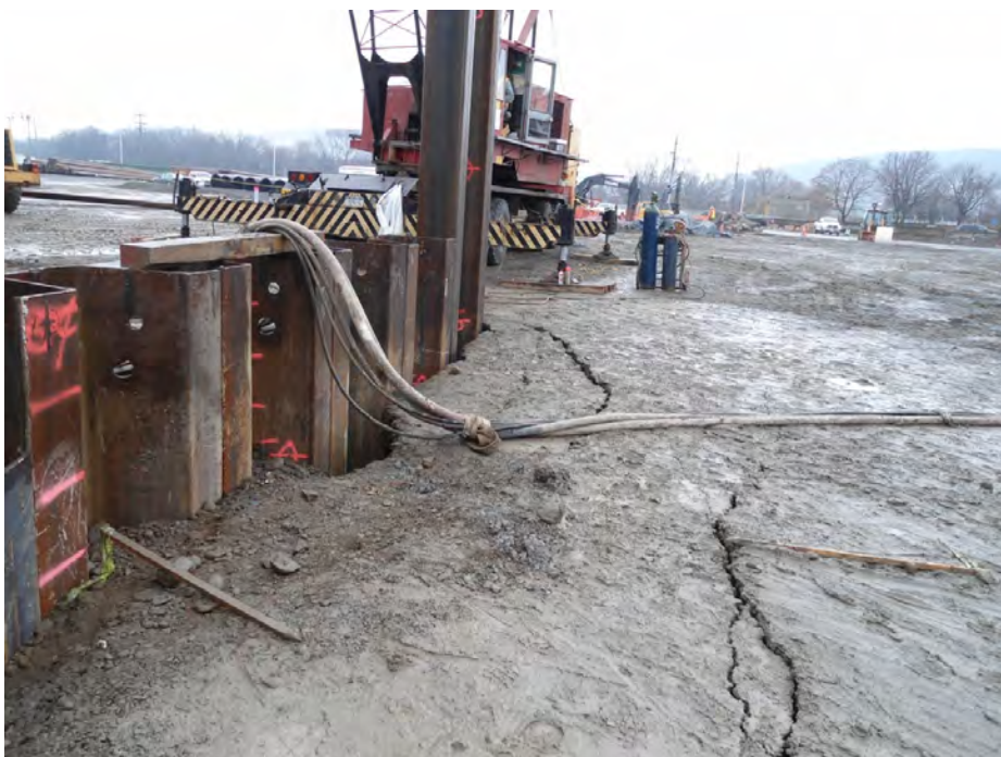
Soil compaction and cracking along west sheeting alignment
