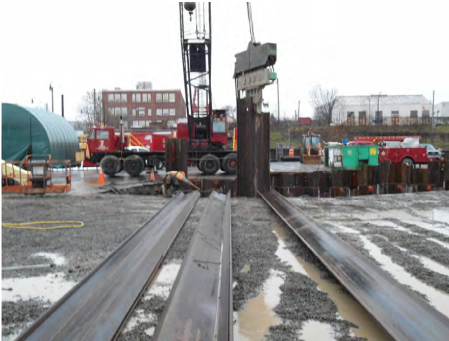
Sheeting installation at southern end of site. Photo facing west.
