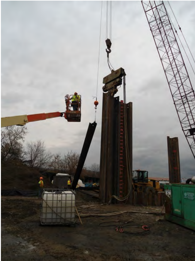
Installing sheets along west sheeting alignment
