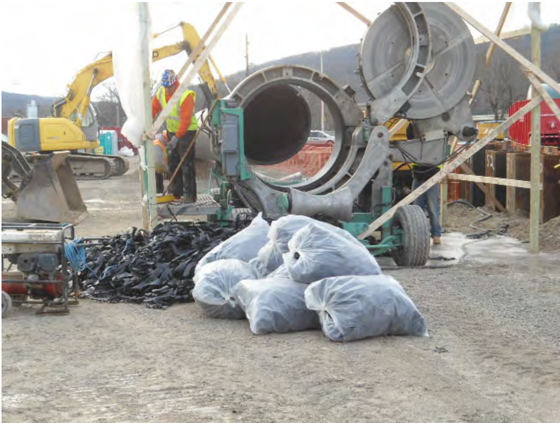
HDPE pipe trimmings generated during butt-fusing of the fourth section of pipe (facing south).
