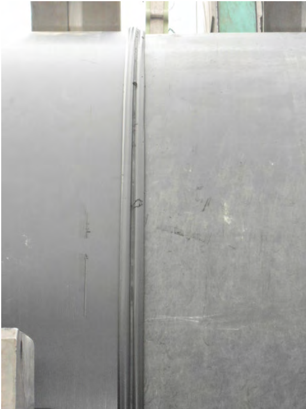
A completed butt fusion of the south flange and an approximately 54-foot section of HDPE (facing west).
