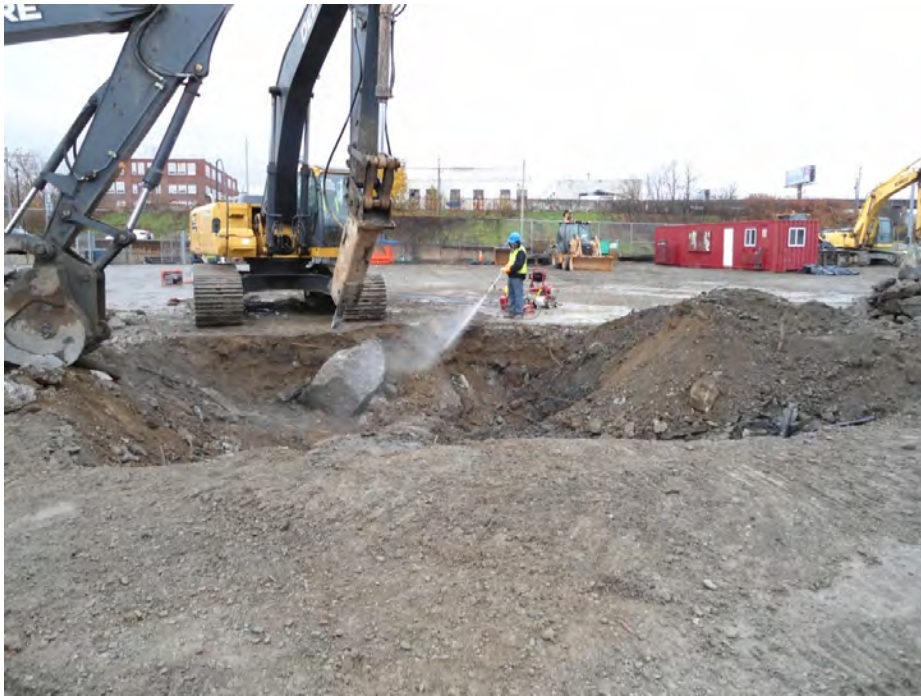
No. 4 Gas Holder foundation demolition
