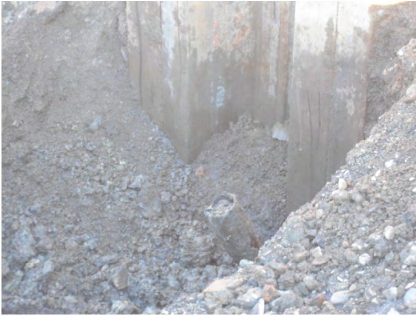
4" pipe conduit located along east alignment in northern half of trench. Determined to be debris pipe after AECOM verified there wasn't pipe in the same vicinity along the west alignment (facing east).
