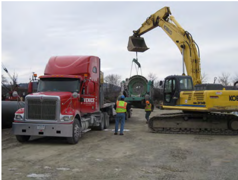
View of the HDPE welder being demobilized.
