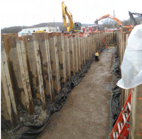
View of trench, Tioga compacting stone overlying geo-textile fabric. Photo taken from southern end of site, facing north.
