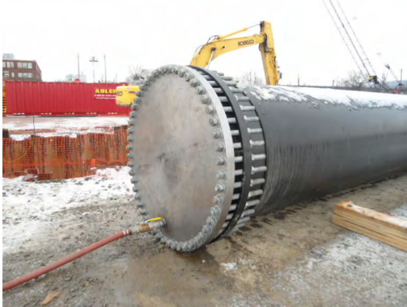
View of blind flange attached to HDPE pipe.
