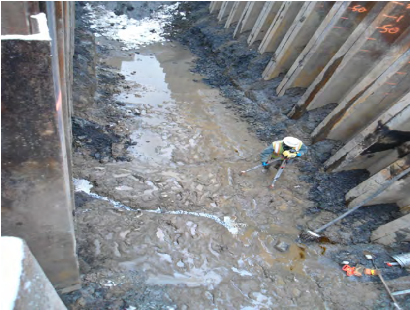
Survey to confirm excavated depths at north end of trench. Photo facing into trench from north end.
