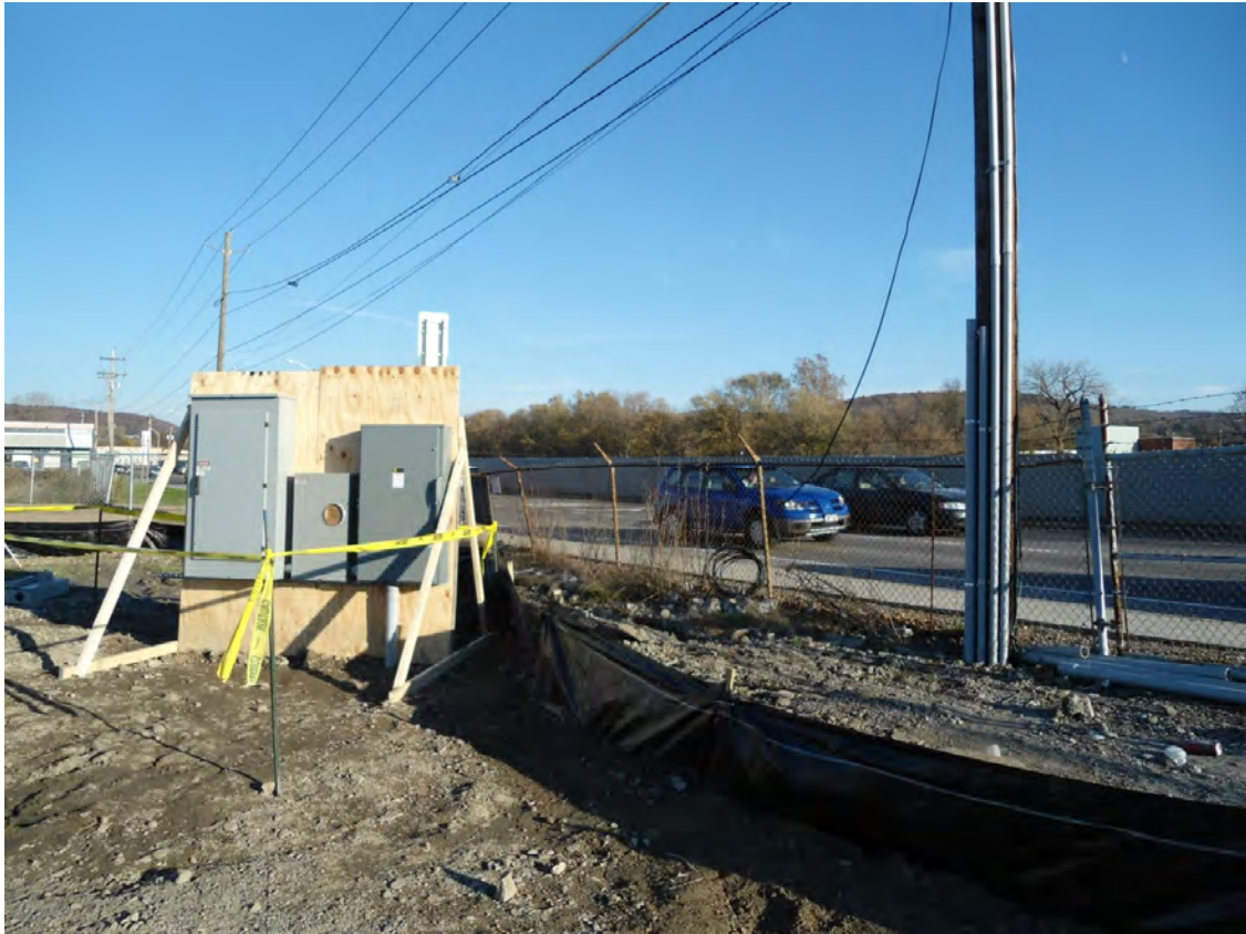
Electrical subpanel
