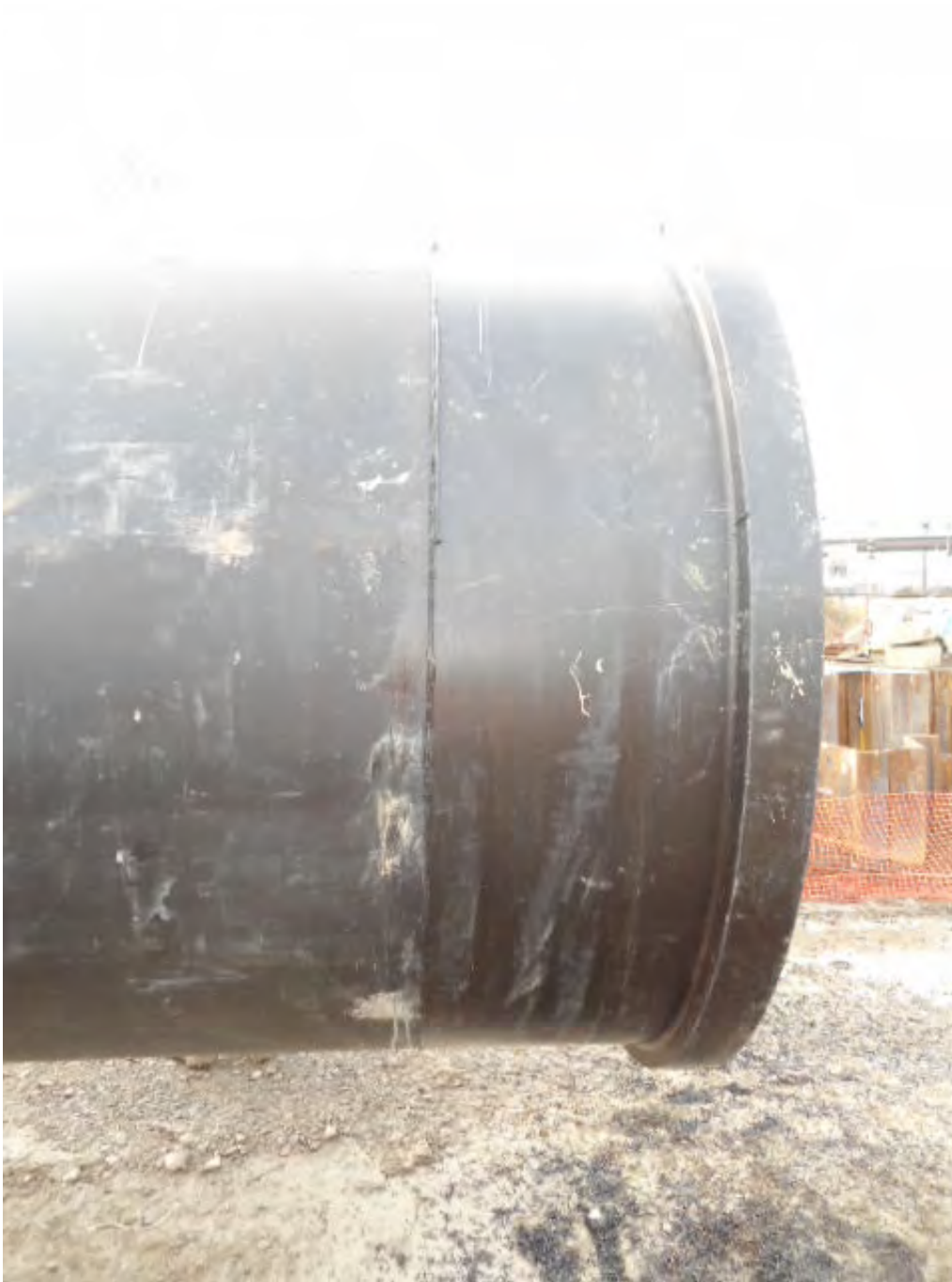
A butt-fused section of HDPE and a flange. The excess material HDPE extruded (bead) during fusion was removed as the pipe cooled (facing west).
