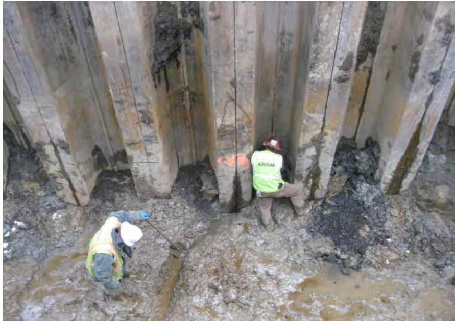
View of AECOM attempting to repair leaking sheets. Photo taken from the western sheet wall facing east into excavation
