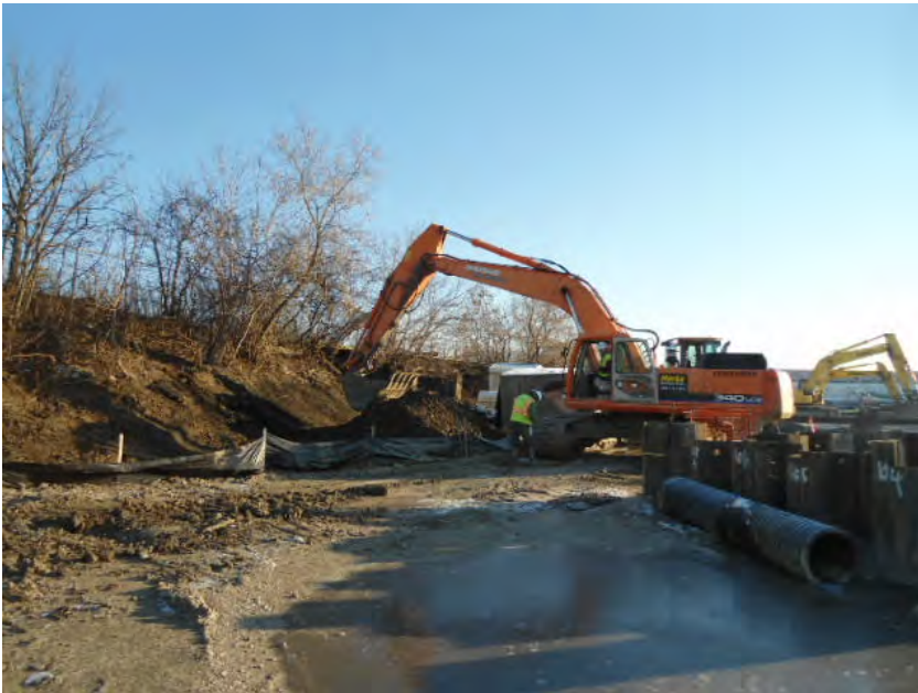
View of AECOM moving stockpiled materials at North end of the site for use in voids and depressions towards to the southern end of the sheet walls. Photo taken from the west, facing east.
