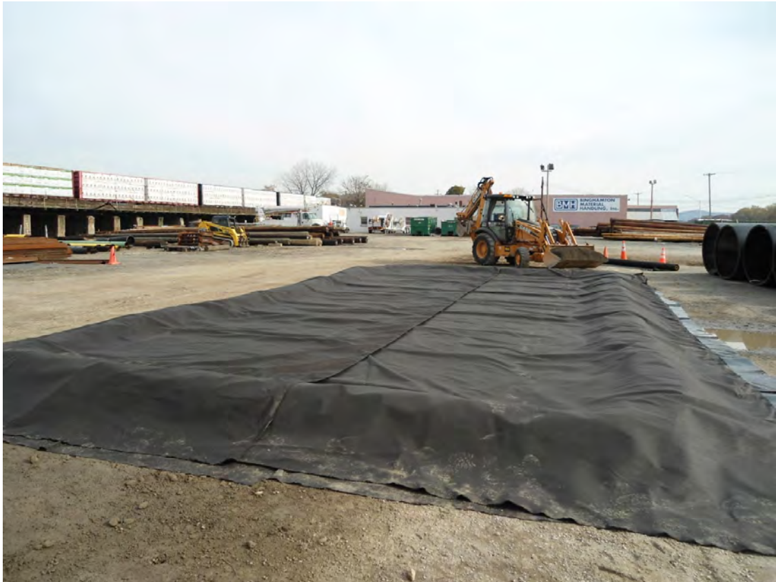
Decontamination Pad liner system (non-woven-geotextile – HDPE liner – non-woven geotextile)
