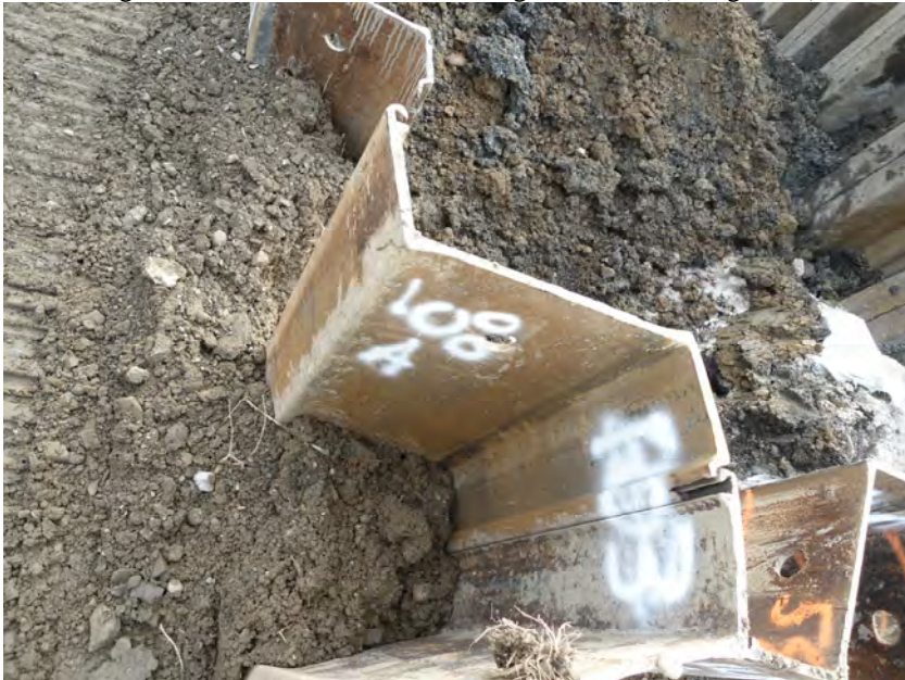
North western corner of sheet pile. Corner piece fabricated onsite by Tioga. Photo taken from above sheet corner at northwest corner of the sheet alignment.
