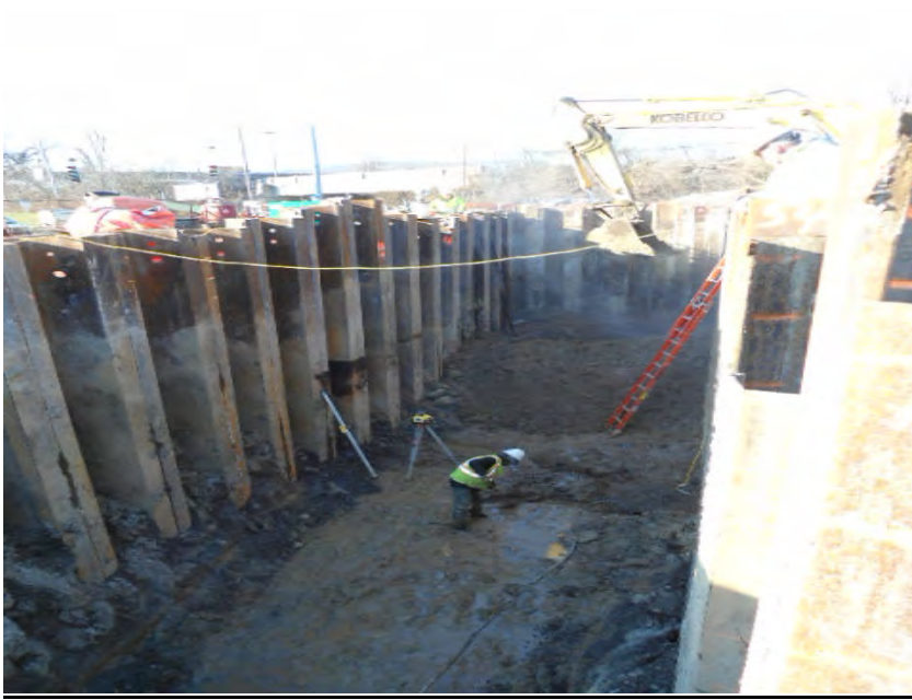
Photo shows trench excavation and AECOM performing dewatering activities in base of trench, at northern end. Photo taken facing north.
