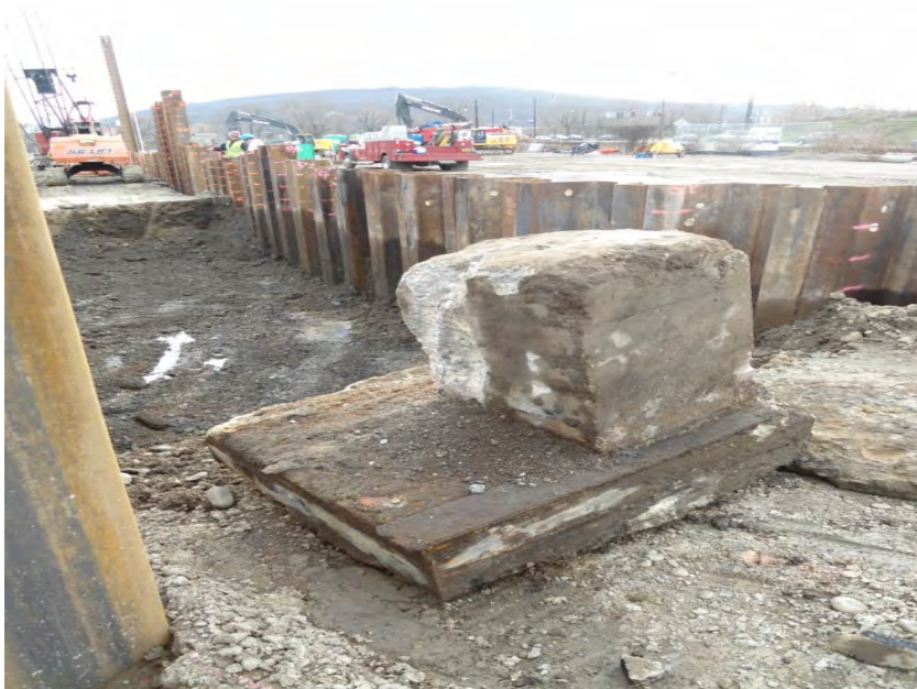
Concrete footing removed from the Manhole MH-1C vicinity. Refer to Drawing 9 for details.
