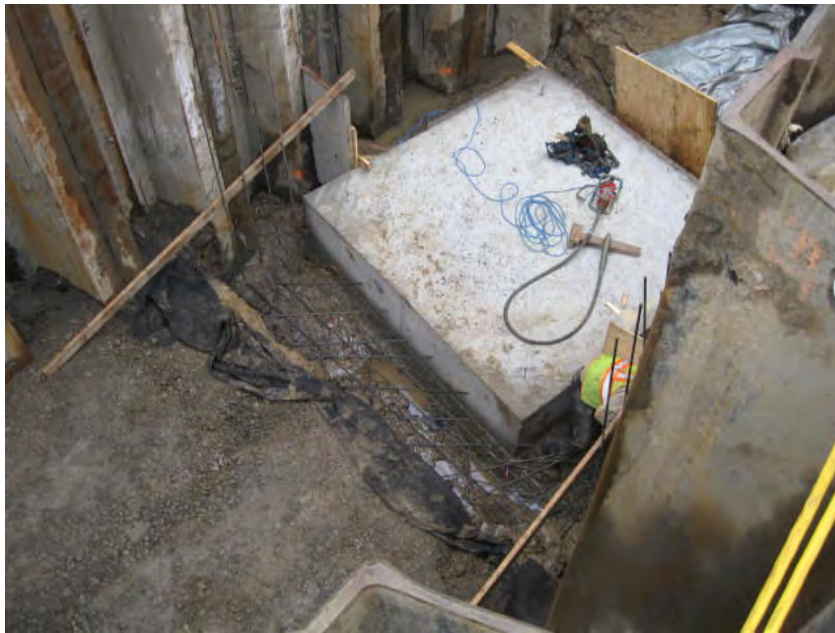
View of the rebar placed for the northern collar at MH-1B.
