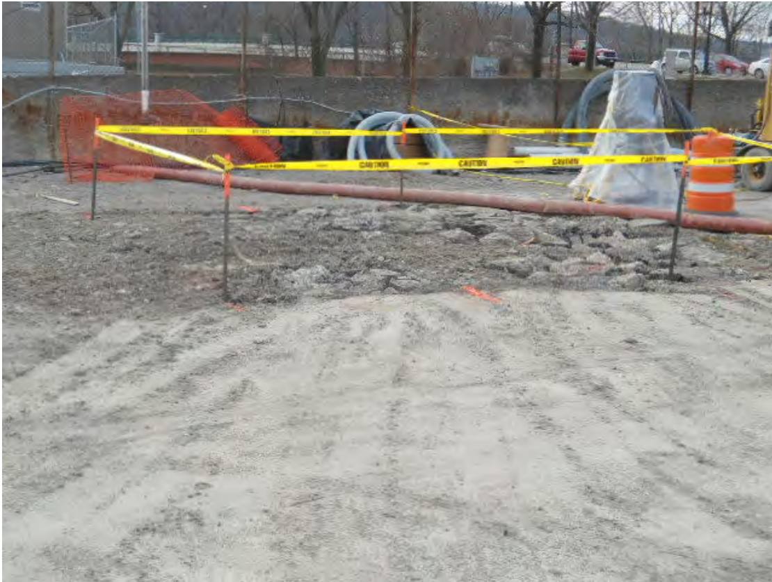
Discharge line of treated groundwater Batches 2-2 and 3. The backfilled test pit excavated 12/27/11 is shown in the secured area (facing southwest).
