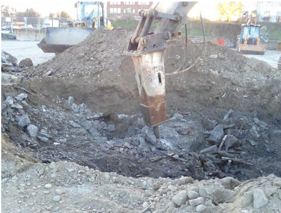
North edge of No. 4 Gas Holder foundation demolition
