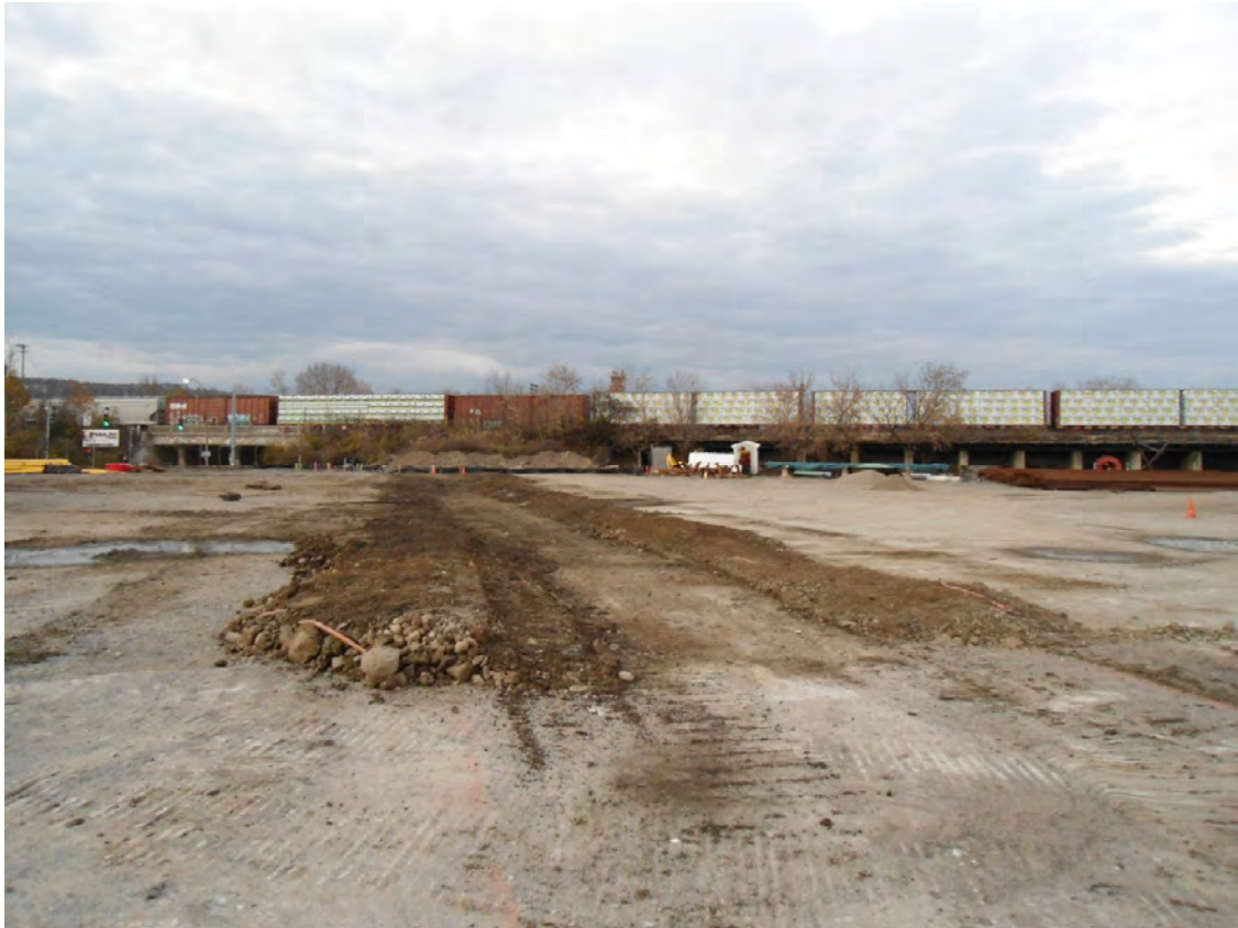
Pre-trenches backfilled
