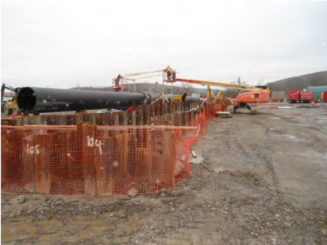
Vari-Tech butt-fusing a section of HDPE and constructing a temporary structure (facing south)
