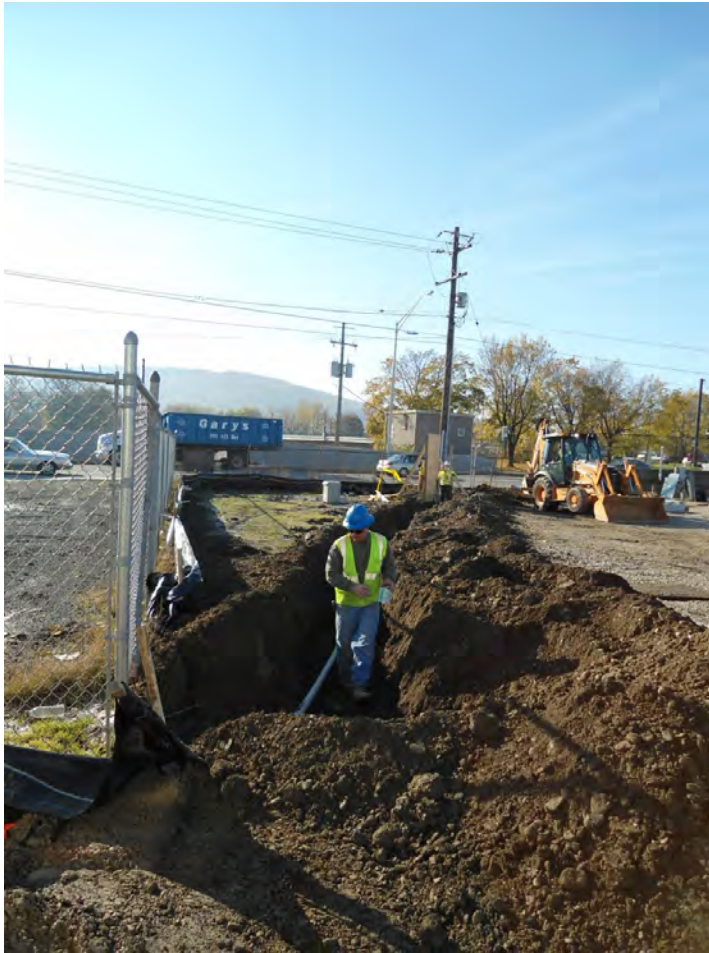
Trench for electrical subpanel power
