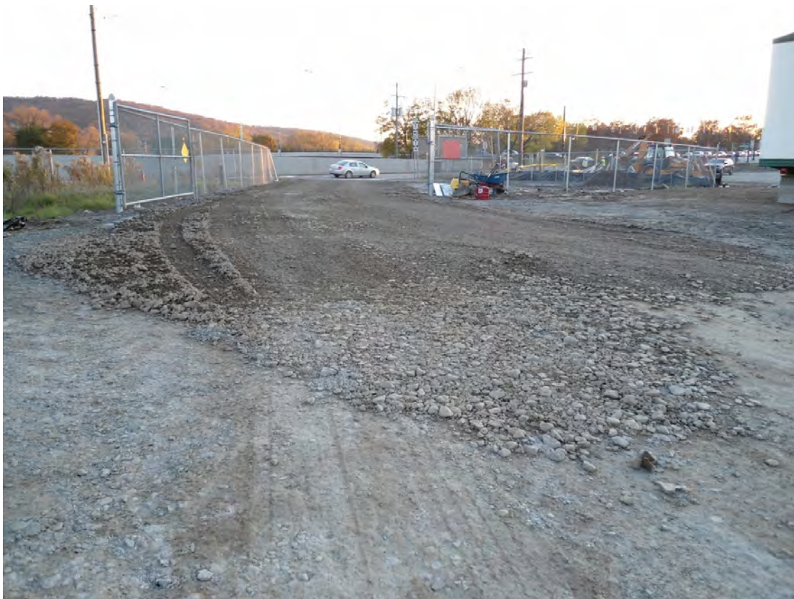
Stabilized Construction Entrance
