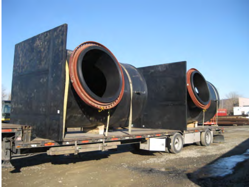
View of the manholes being delivered.
