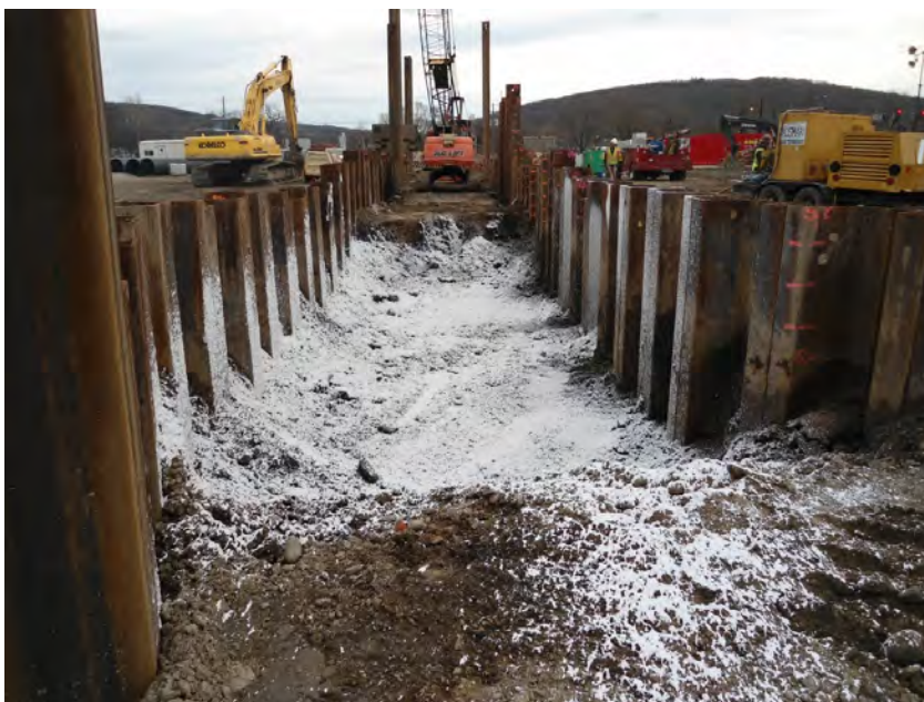
Application of Rusmar foam (facing south)
