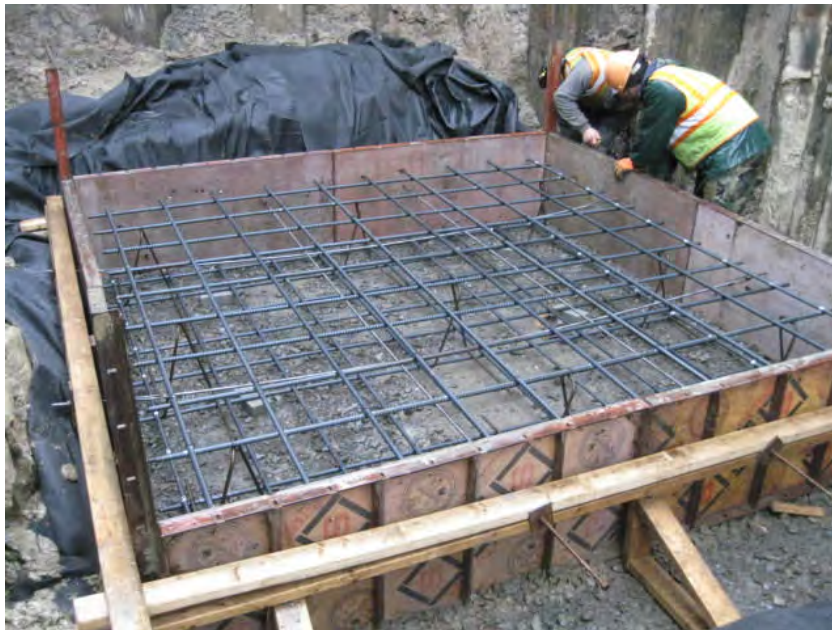
View of concrete forms for MH-1C.
