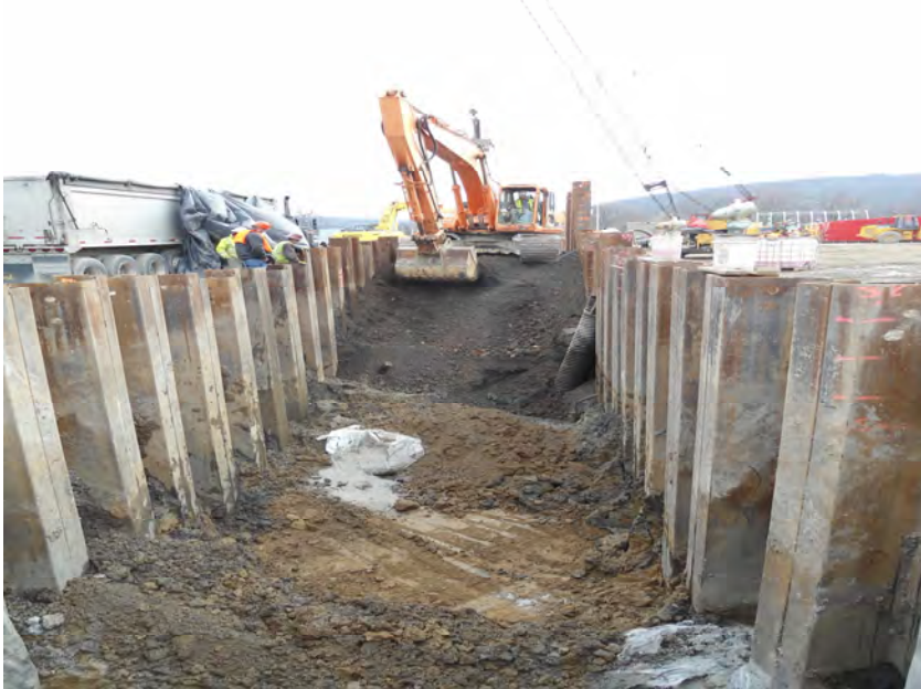
Trench excavation and load-out of material to ESMI at north end of site. Grey CKD can be seen in the excavation, shown prior to mixing in the middle and lower right side of this photo. Photo taken from the north end of the excavation facing south.
