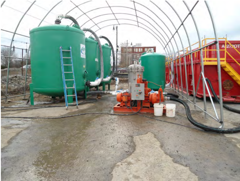
Temporary Water Treatment System components shown after initial system start up, prior to secondary containment being place and completion of tent. Photo facing west.
