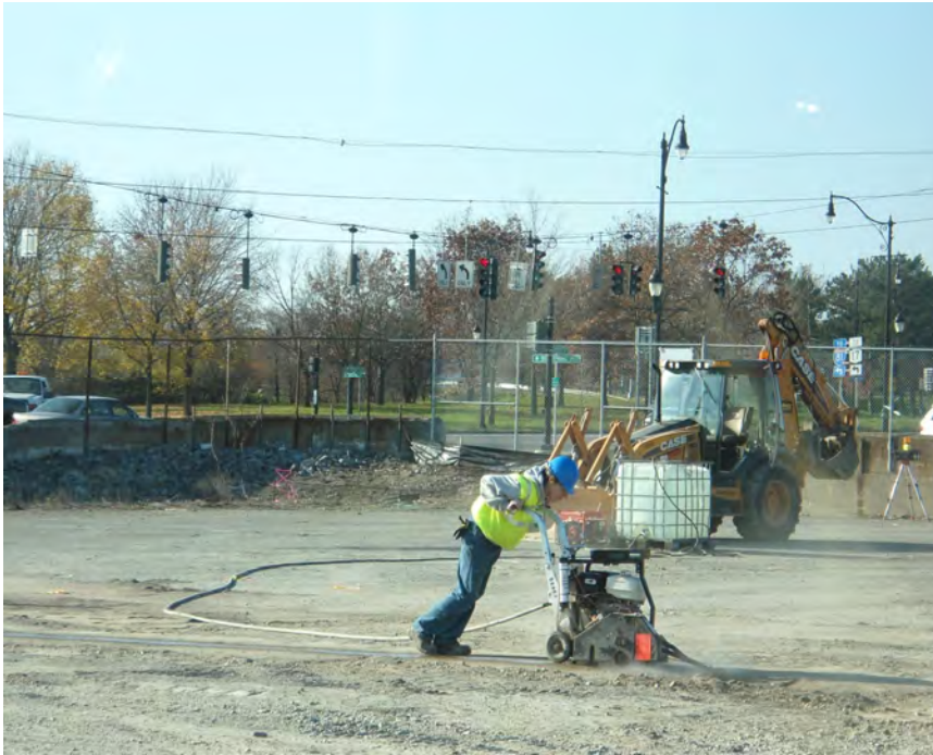
Saw cutting asphalt slab over No. 4 Gas Holder foundation
