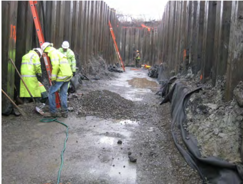
View of AECOM installing dewatering sumps below the crushed stone layer.
