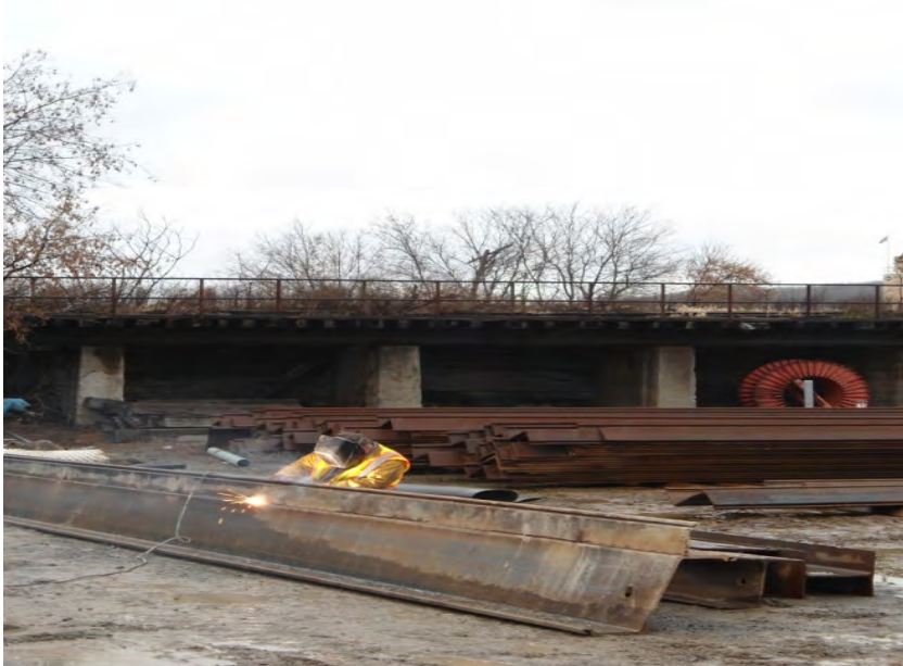
Fabricating corner sheets to be used at north and south ends of the sheet alignment. (facing north)
