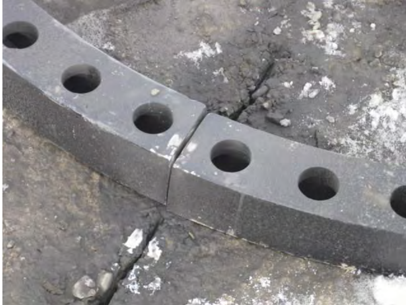
View of a backer ring cut in half to fit over the HDPE ring.
