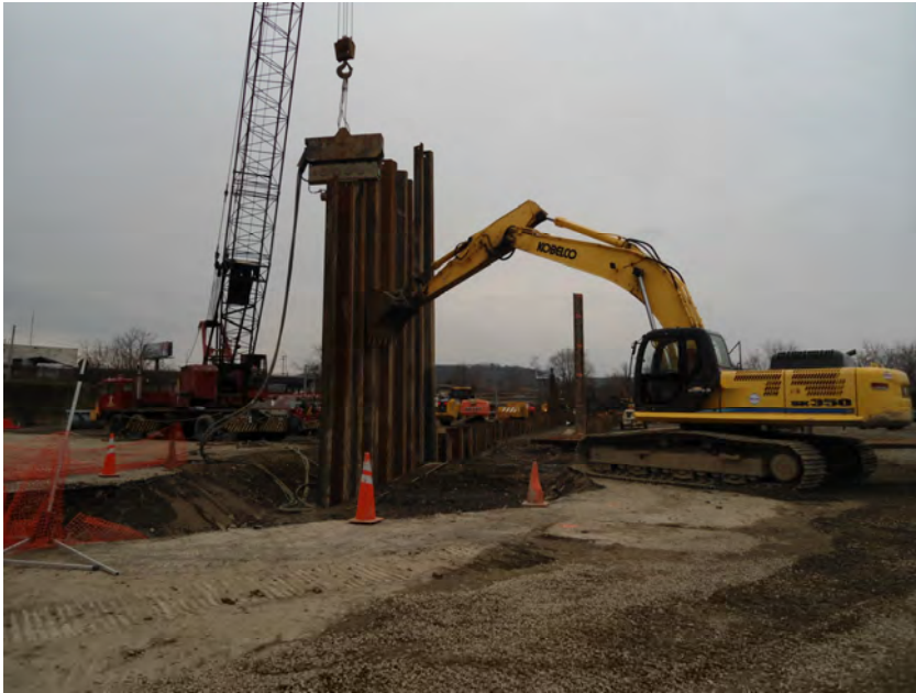
Installing the sheets along the west alignment (facing northwest).
