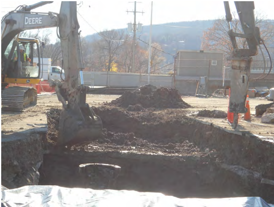
Continued No. 4 Gas Holder foundation demolition and pipe trench excavation
