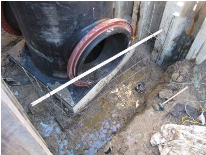
View of re-bar being placed for the southern collar at MH-1C.
