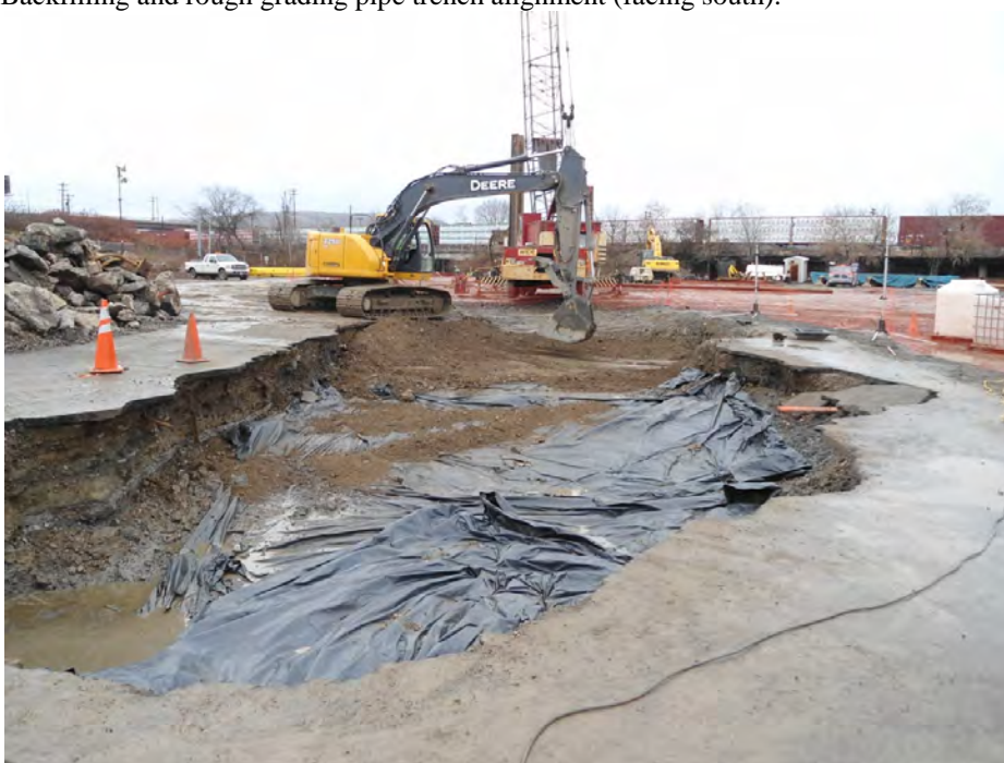
Temporarily backfilling the No. 4 Gas Hold foundation (facing north)
