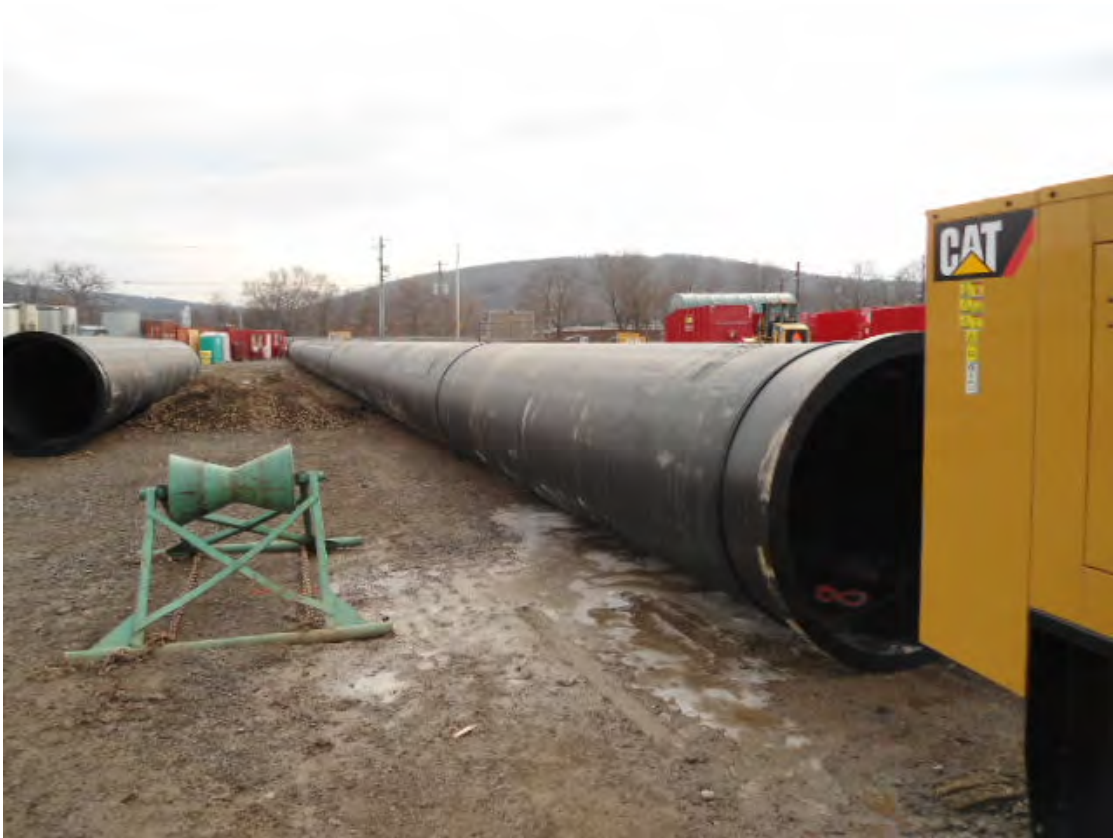
A completed butt-fused section of HDPE piping (facing southwest).
