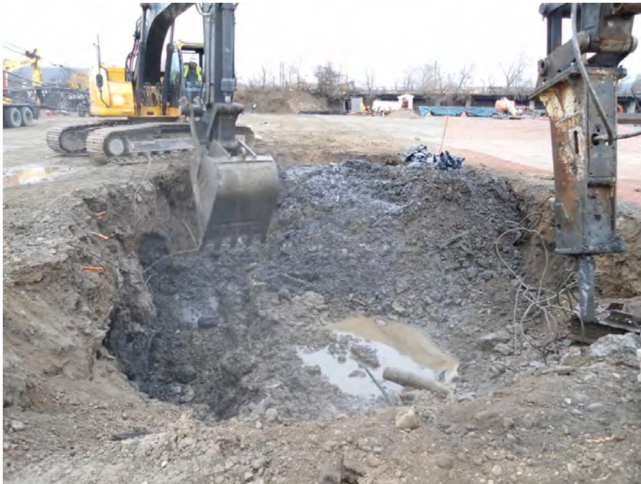
No. 4 Gas Holder foundation demolition
