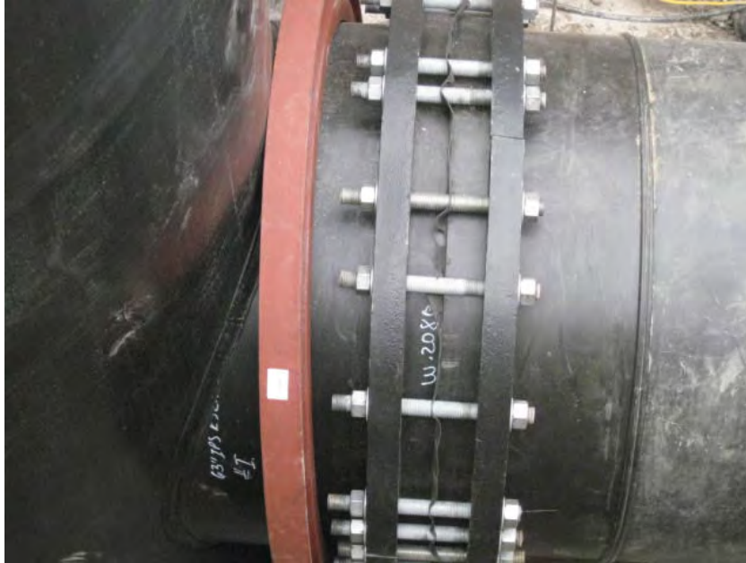
View of temporary connection at MH-1C (to secure HDPE for backfill until new rings arrived onsite)
