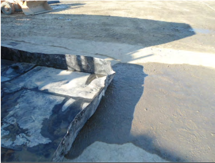
Leaks in secondary containment under Frac Tank. Photo taken at south west corner of site near TWTS.
