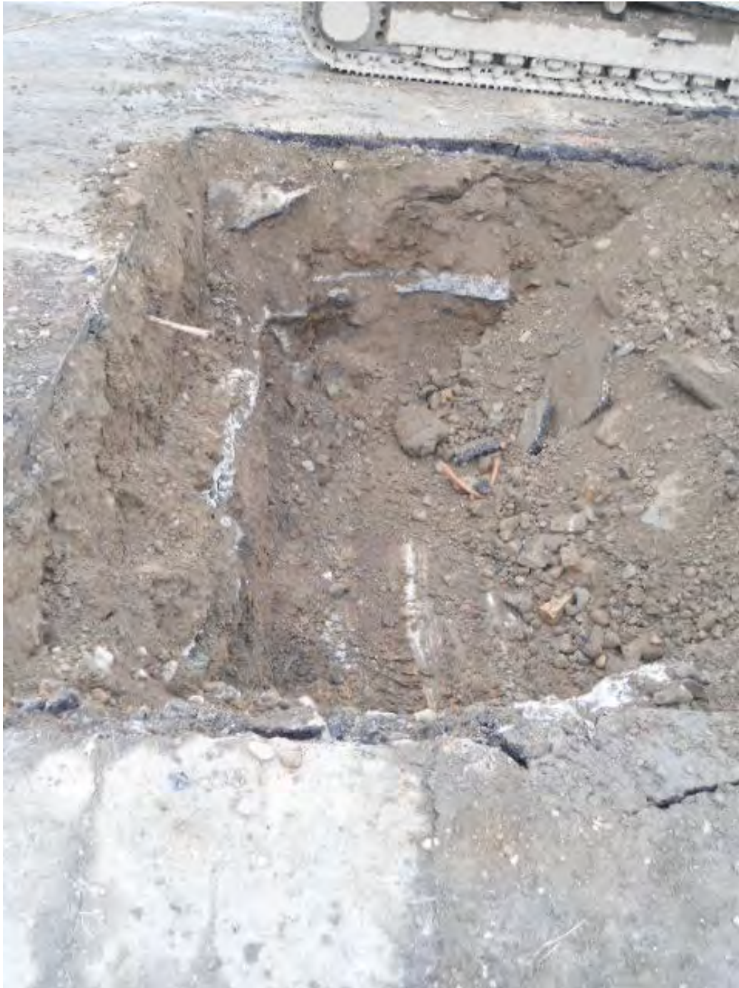
Test pit to locate the existing storm sewer. The test pit was located adjacent to the southwest corner of the trench north of the existing manhole along Court Street. (facing north).
