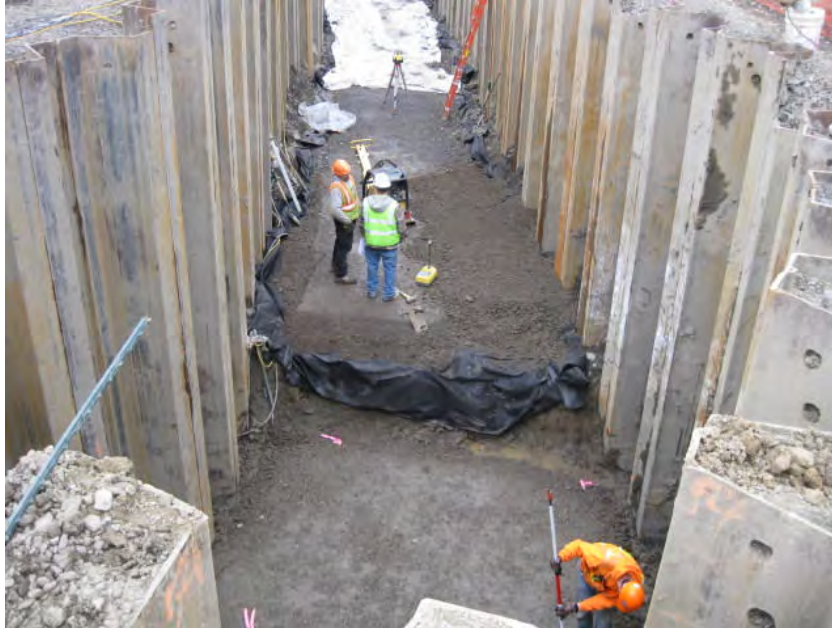
View of ATL testing compaction.
