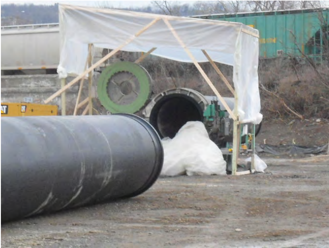
Butt-fusing a section HDPE piping and flange with a second flange (facing north).
