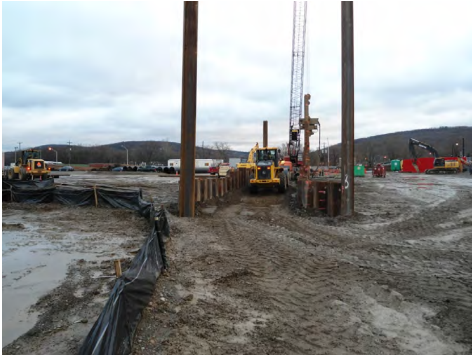
Backfilling and rough grading pipe trench alignment (facing south).
