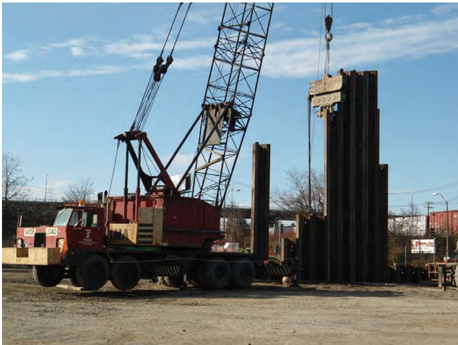
Sheeting installation along east alignment, facing northwest.
