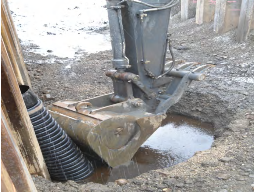
Maintenance of sump at northwest side of trench. Photo taken looking over west sheet alignment.
