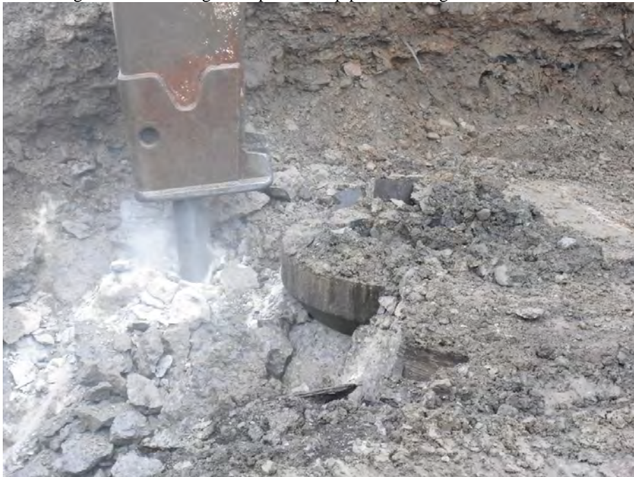
No. 4 Gas Holder foundation demolition, 30" diameter vertical iron pipe encountered
