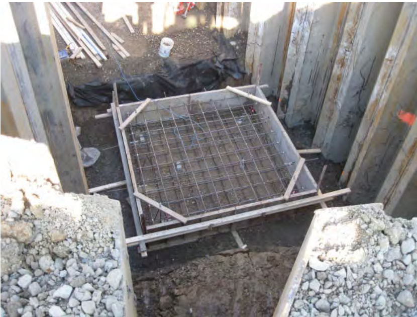
View of forms and re-bar for the base of MH-1B.
