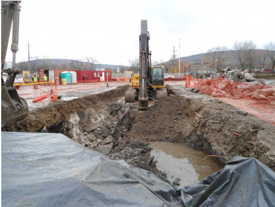
Performing excavation along north portion of pipe trench alignment
