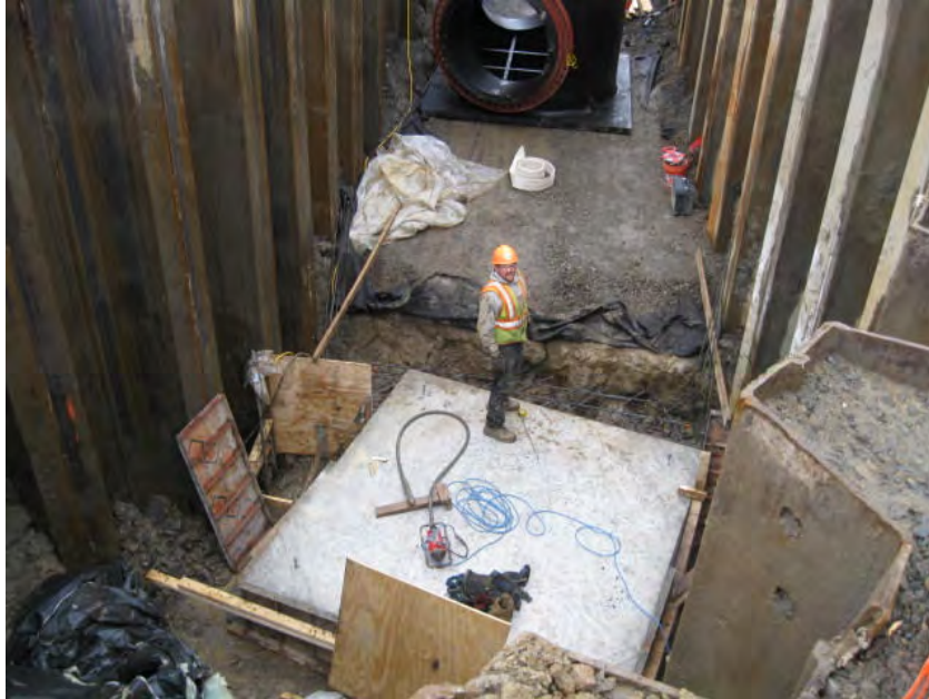
View of the base for MH-1B after forms are removed.
