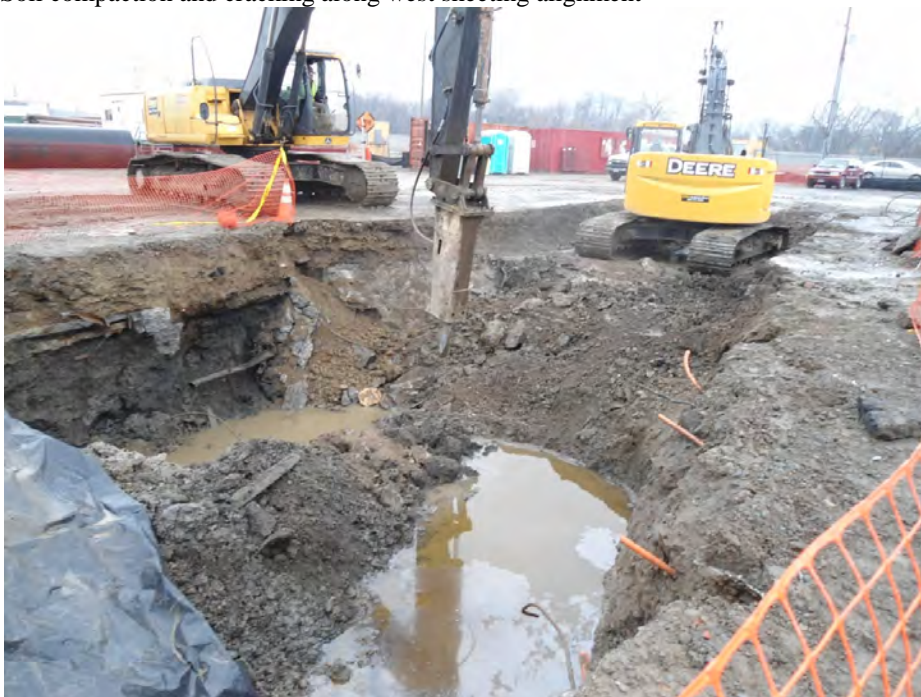
No. 4 Gas Hold foundation demolition and pipe trench excavation
