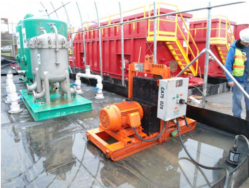
Secondary containment in place under TWTS components. Photo taken at south end of site facing west.
