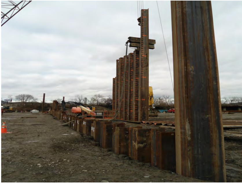
Tioga installing sheets along the east sheeting alignment (facing northeast)
