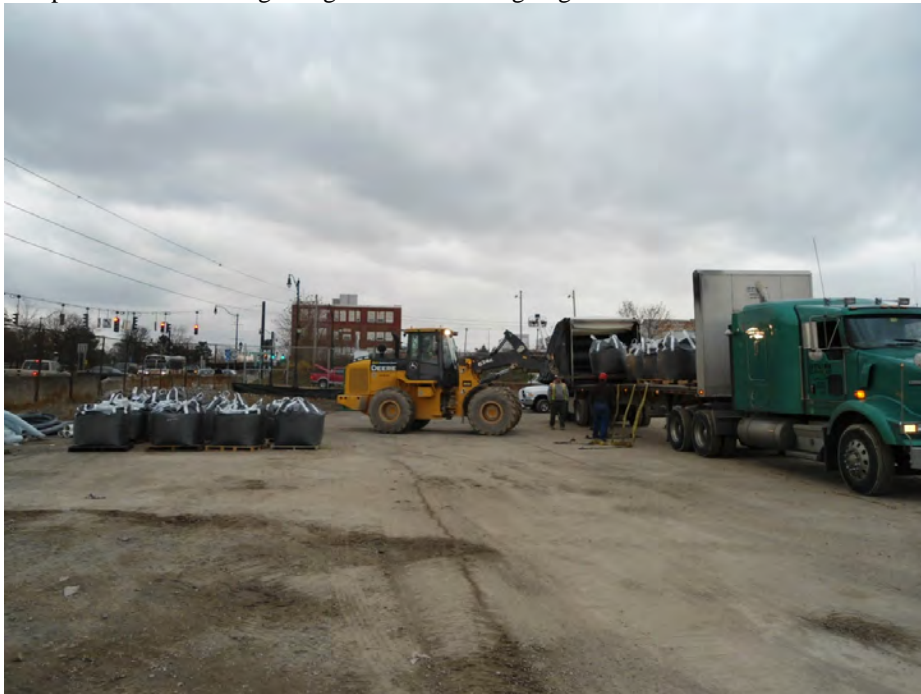
Mobilization of TWTS components and media
