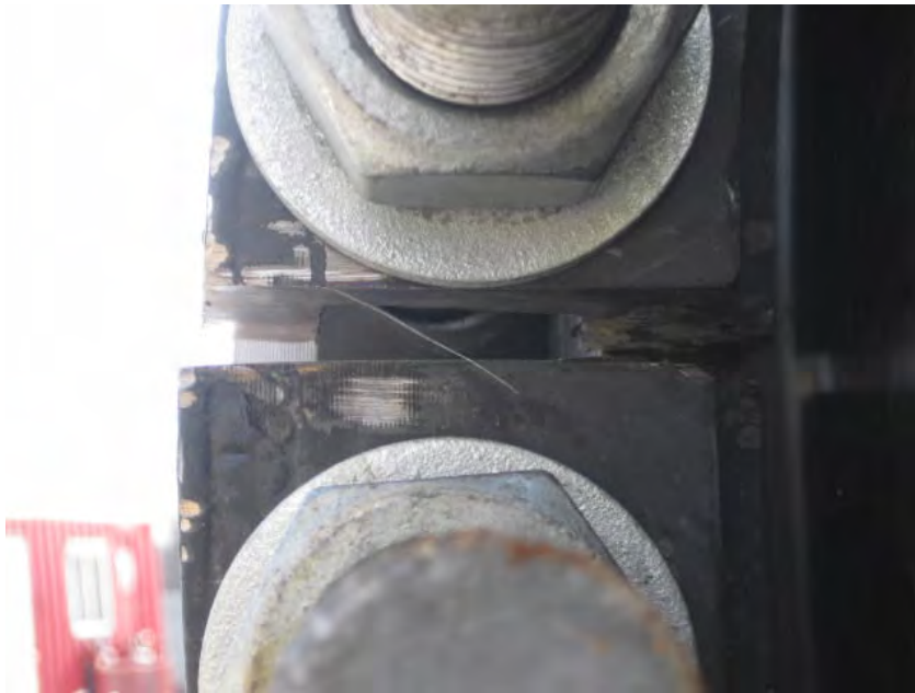
View showing a split backer ring installed on the pipe.
