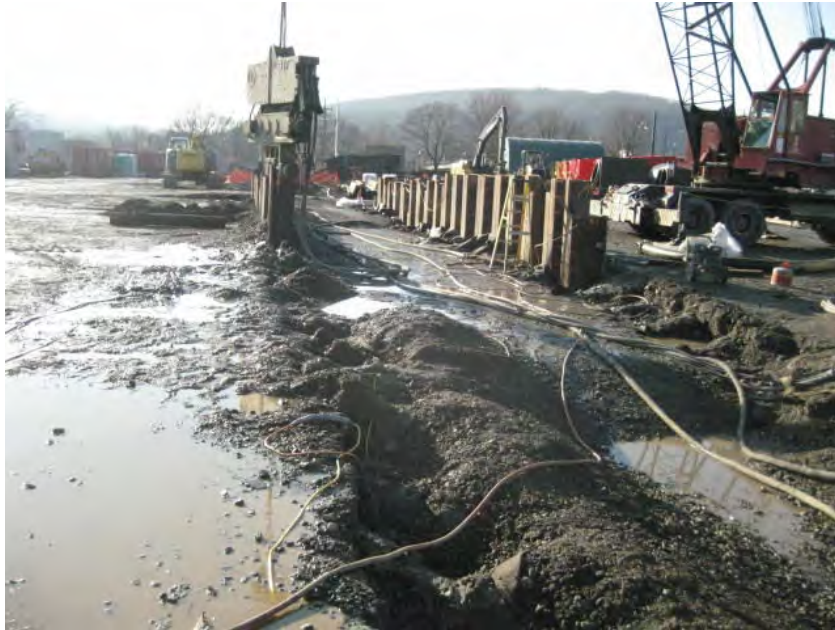
View of Phase One sheeting being removed.
