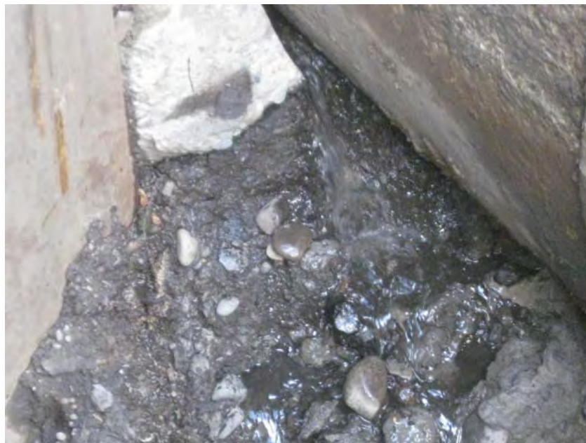
View of water leaking from the (lower/bottom) SW corner of manhole MH-2. Note that the white rock visible to the right of the pipe appears to be a former “patch” that was placed previously in an attempt to repair the leak.
