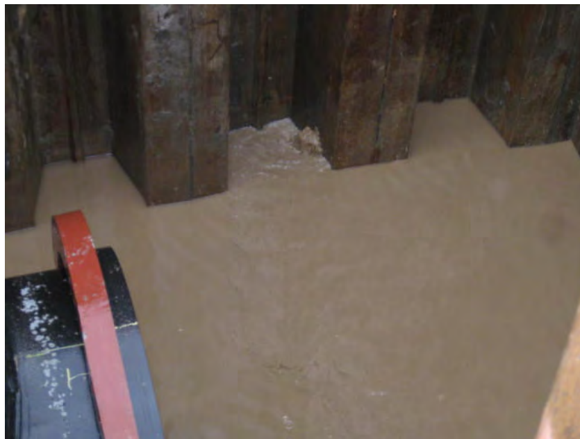
View of water upwelling from below concrete near MH1-C.
