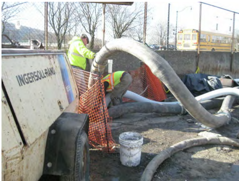
View of AECOM removing the bypass pump lines from MH-1.
