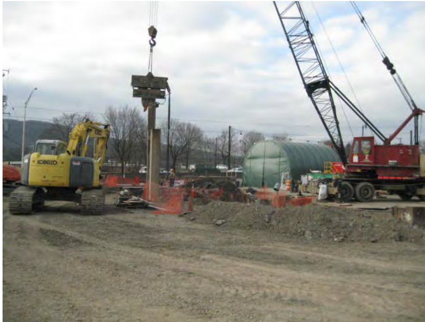
View of Tioga driving sheets at the southern Phase Two area.
