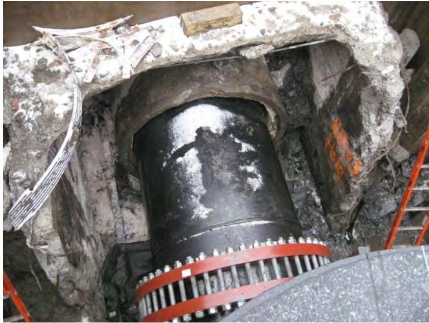
View of the slip-lined portion of HDPE pipe at MH-1.
