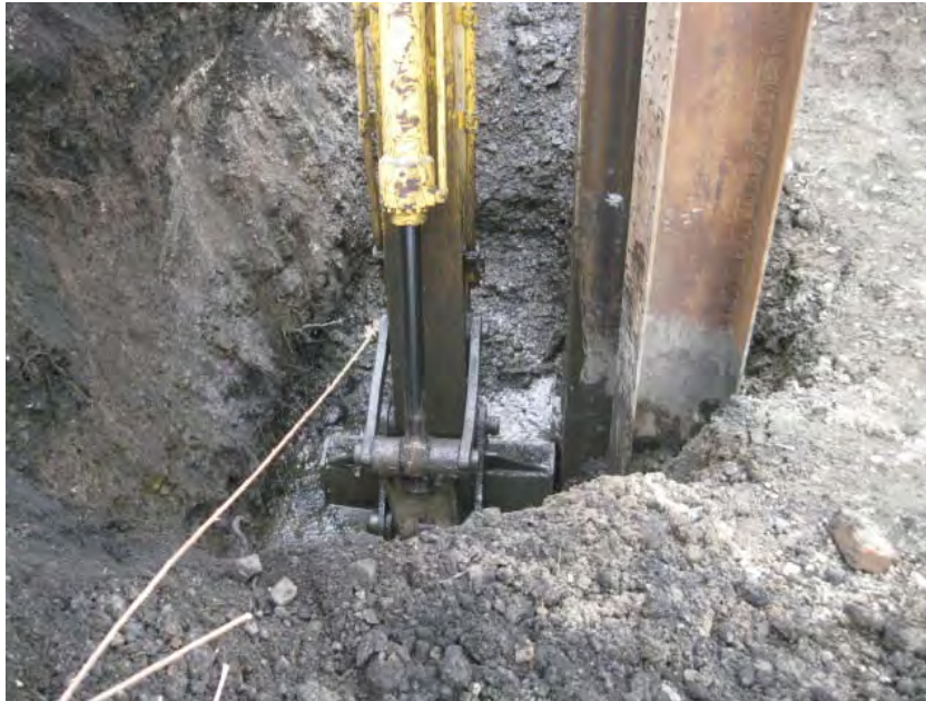
View of Tioga attempt to remove concrete obstructions near MH-2.
