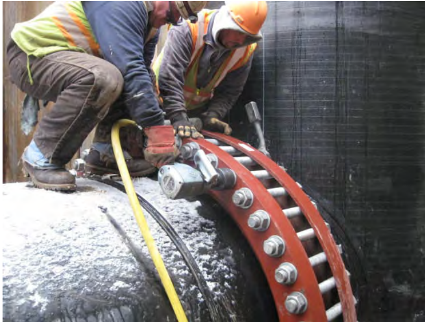
View of Tioga personnel re-setting the torque on the flange connections at MH-1B.
