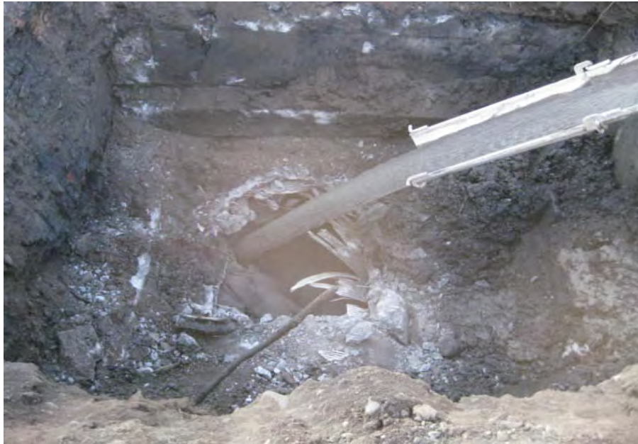
View of CLSM being poured into the existing sewer.
