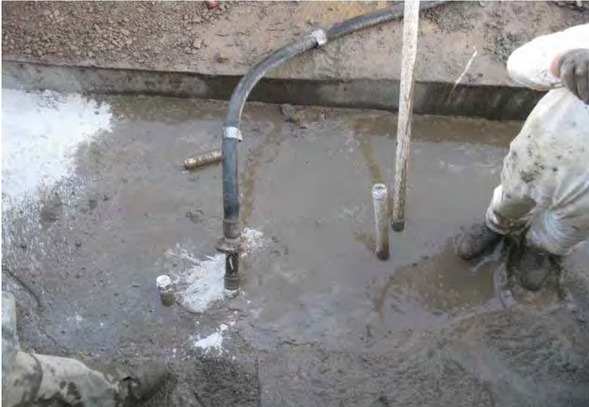
Photo #57 (2012.03.21): View of grouting of the slip-lined section of HDPE pipe at MH-1.
