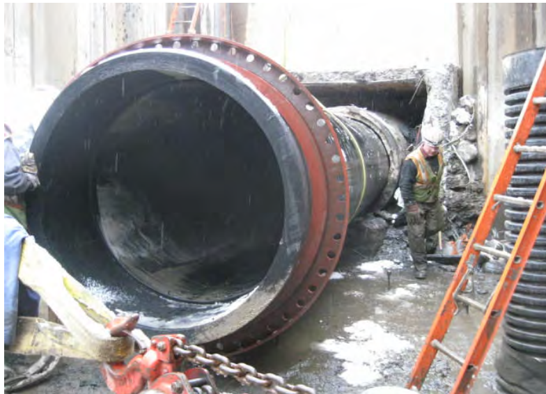
View of the HDPE being slipped into the RCP at MH-1.
