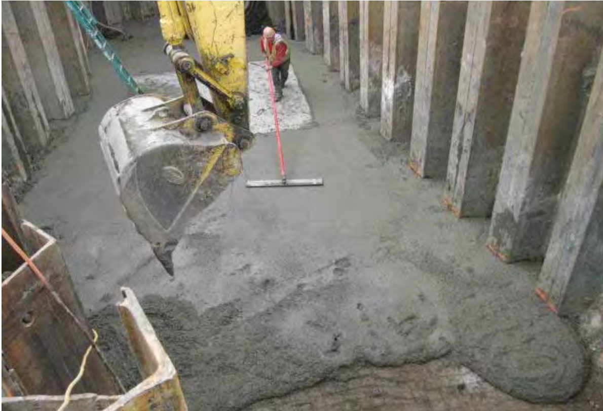
Photo #45 (2012.02.21): View of the emergency concrete spillway between MH-2 and MH-1C being poured.
