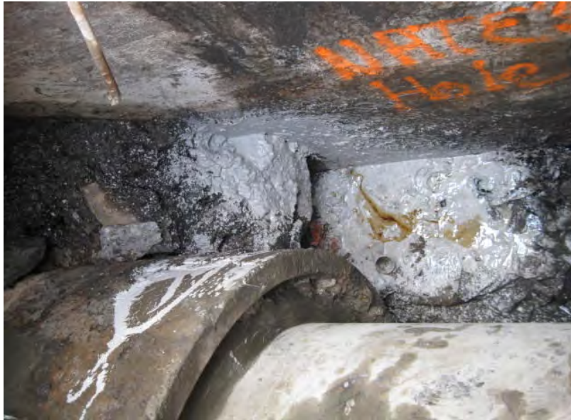
View of the grout leaking from MH-1.
