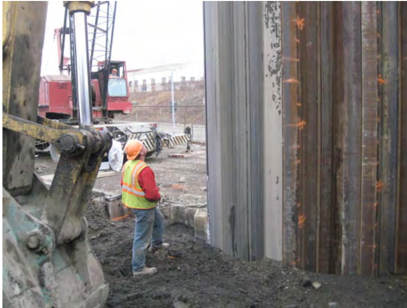
View of Tioga driving sheets at the northern end of the phase two area.
