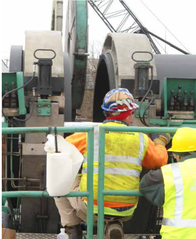
Photo #22 (2011.12.27): Facing west. Vari-Tech setting up the south flange and an approximately 54-foot pipe section for surface 'trimming'.
