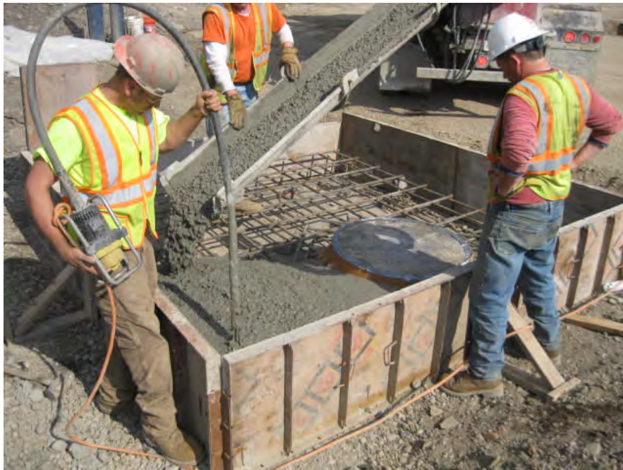
View of concrete being poured at MH-1D.
