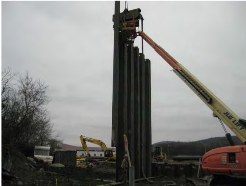
View of Tioga personnel driving the northern section of the phase two sheets (facing east).
