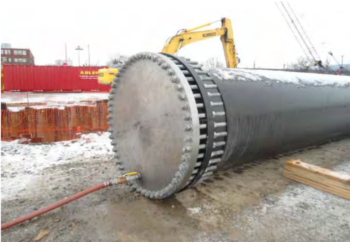
Photo #34 (2012.01.17): Facing west. View of blind flange attached to HDPE pipe for leak test.
