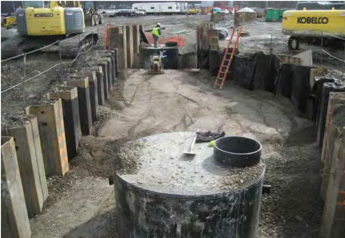
Photo #54 (2012.03.09): View of backfill between MH-1D (foreground) and MH-1C (background).
