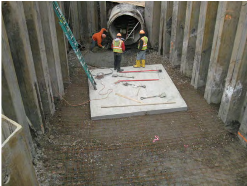
View of the concrete base for MH-1D. Wire “fabric” is also in place for the emergency concrete spillway between MH-2 and MH-1C. (MH-2 is visible at the top of the photo with RCP)
