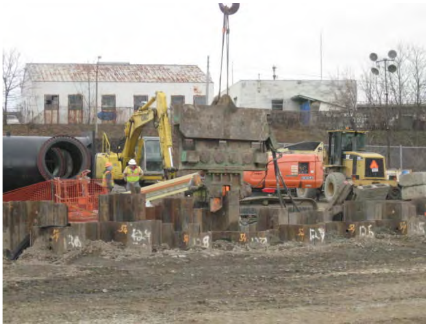
View of Tioga pulling phase one sheeting.
