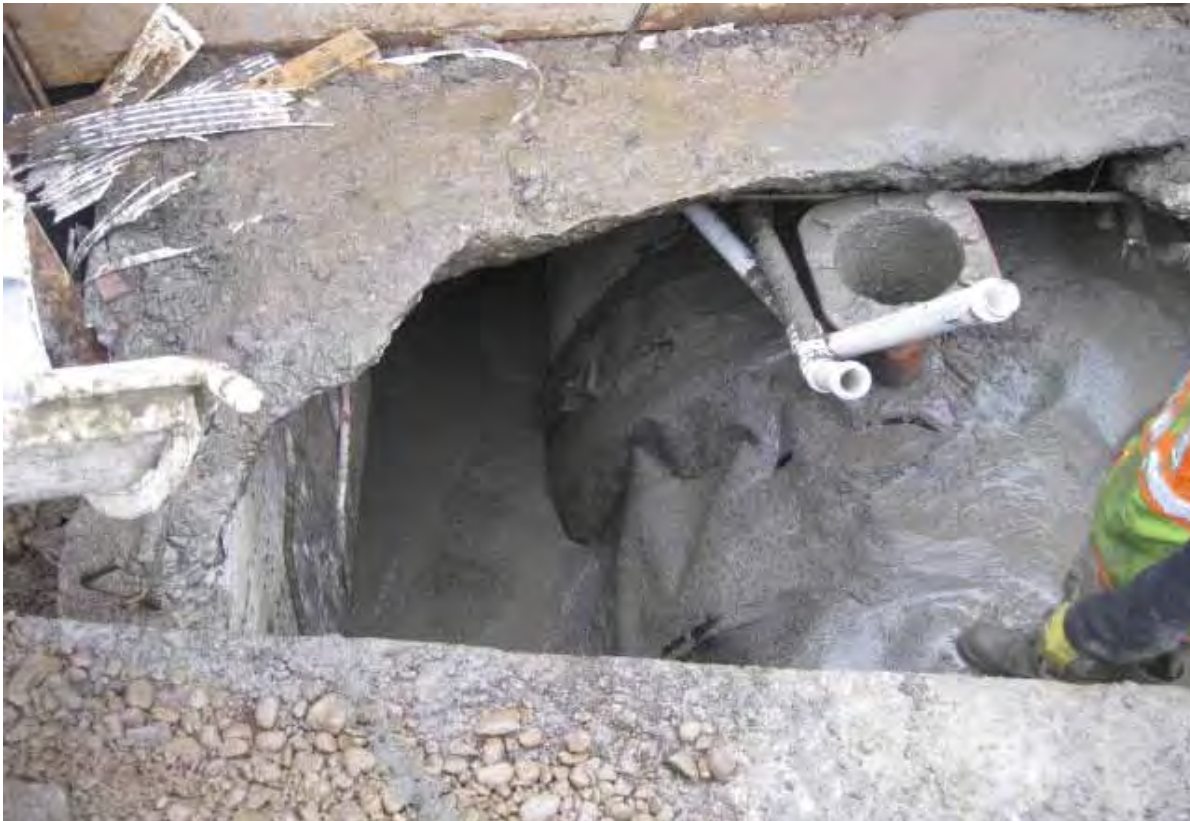
Photo #56 (2012.03.16):View of grout being placed inside Fernco at MH-1 and CLSM being poured outside the Fernco.
