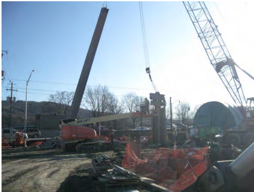
View of Tioga driving Phase Two sheets at the south end of Phase Two area.
