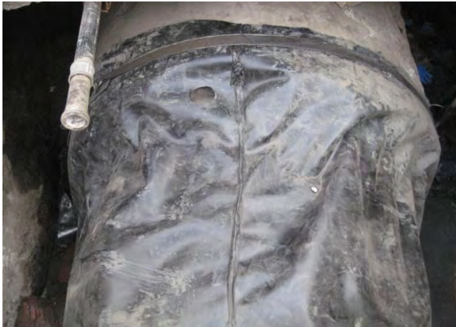
View of the completed Fernco connector at MH-1.
