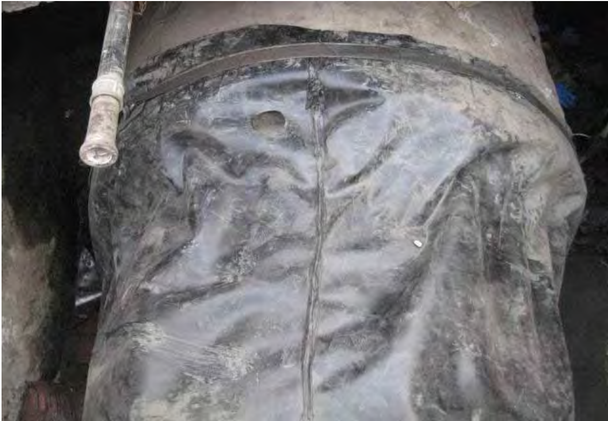
Photo #55 (2012.03.15):View of the completed Fernco connector at MH-1.
