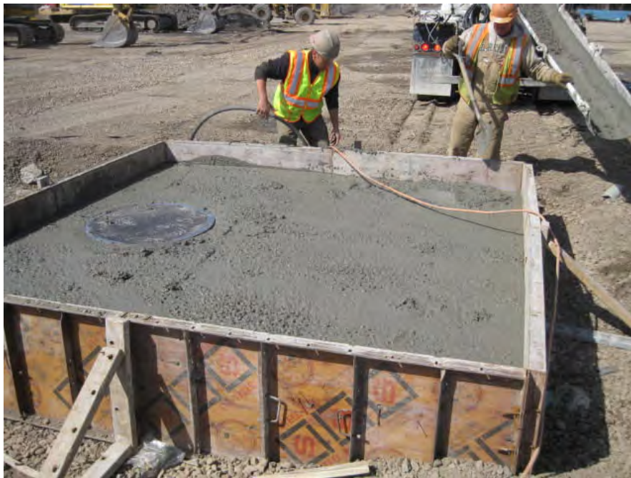
View of concrete being poured at MH-1B.
