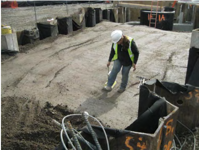
View of compaction testing near MH-1A.
