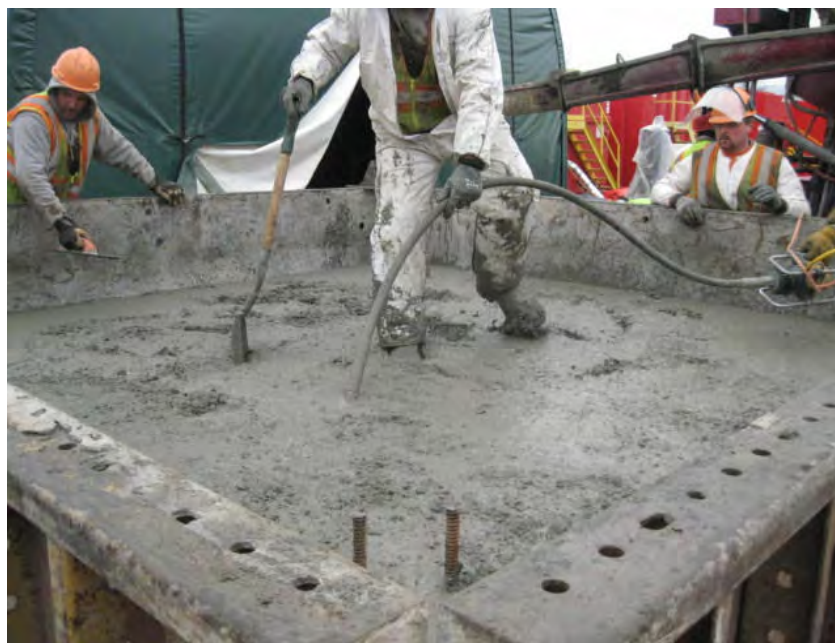
View of MH-1A base showing lifting rods poured into the base (lower/center in photo).
