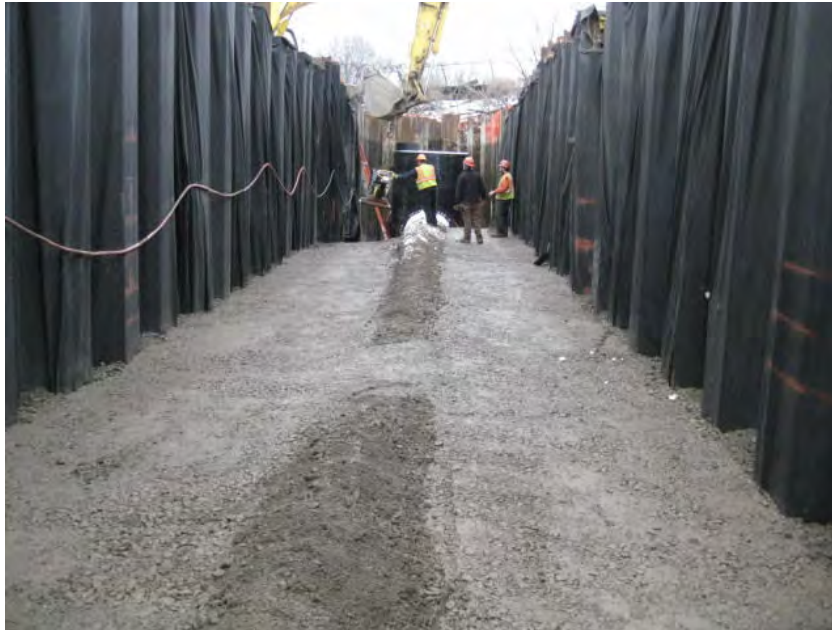
View of backfill being placed on top of the HDPE pipe. Geotextile fabric is visible on the side of the trench (facing north).
