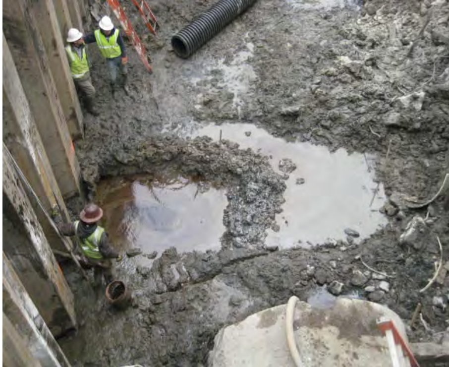
View of impacted water upwelling from the subgrade at MH-1A.
