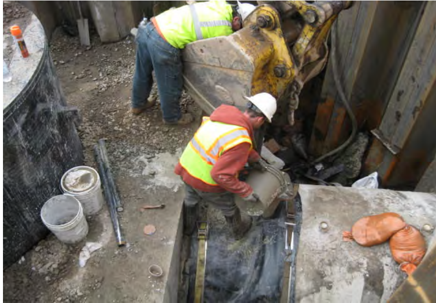
View of AECOM pouring grout into the Fernco at MH2.
