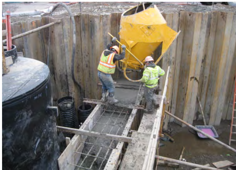
View of the concrete collar being poured at MH-1A.
