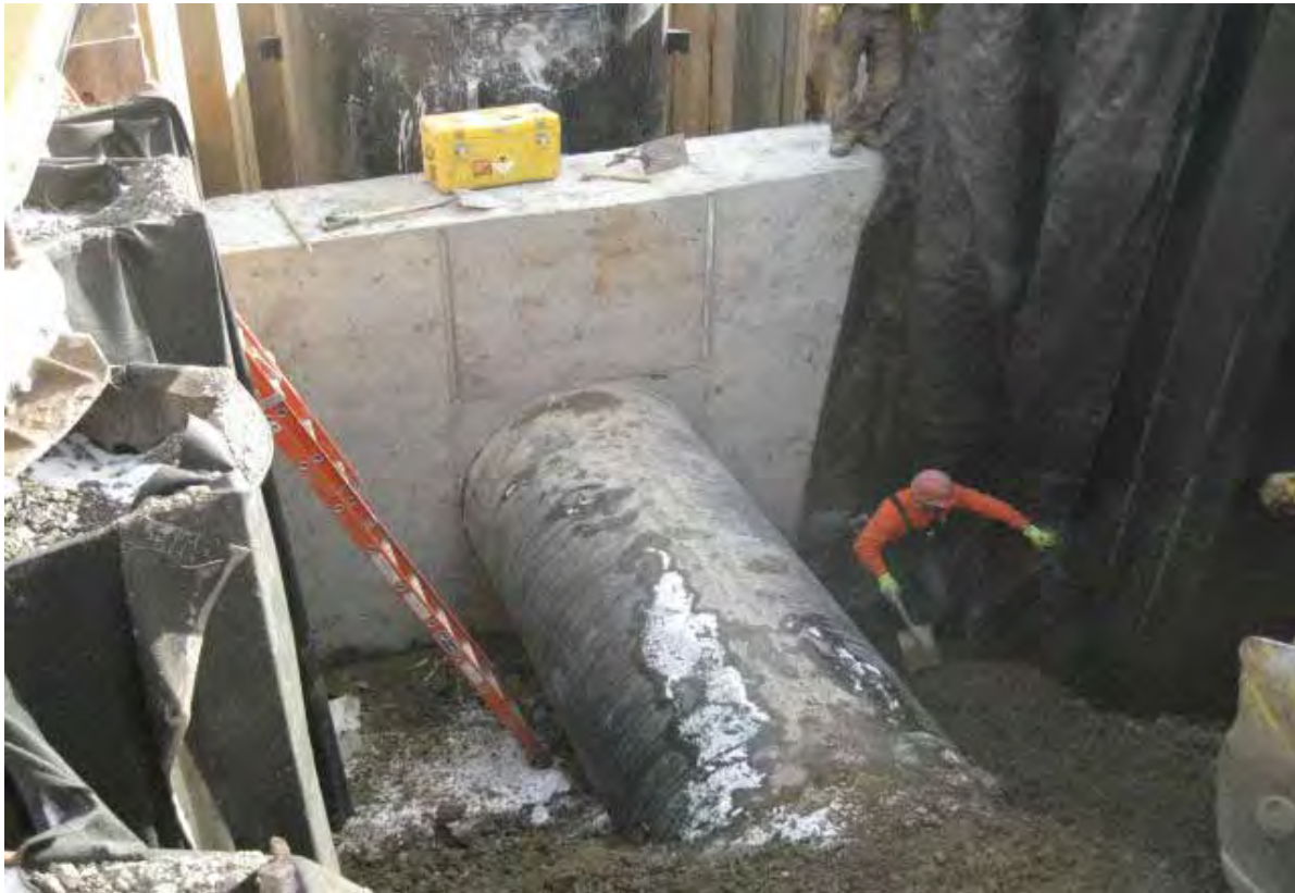
Photo #39 (2012.01.30): View of concrete collar at MH-1B.
