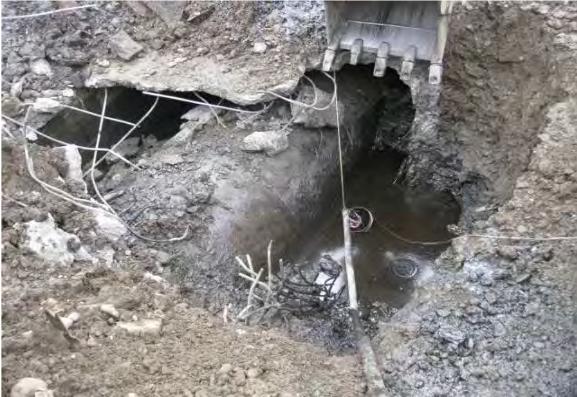
Photo #41 (2012.02.01): View of concrete pipe chase and exposed RCP sewer.
