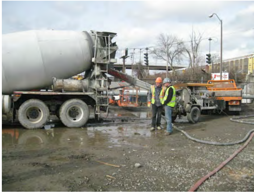
View of the grout pump used for the slip-lined sections.
