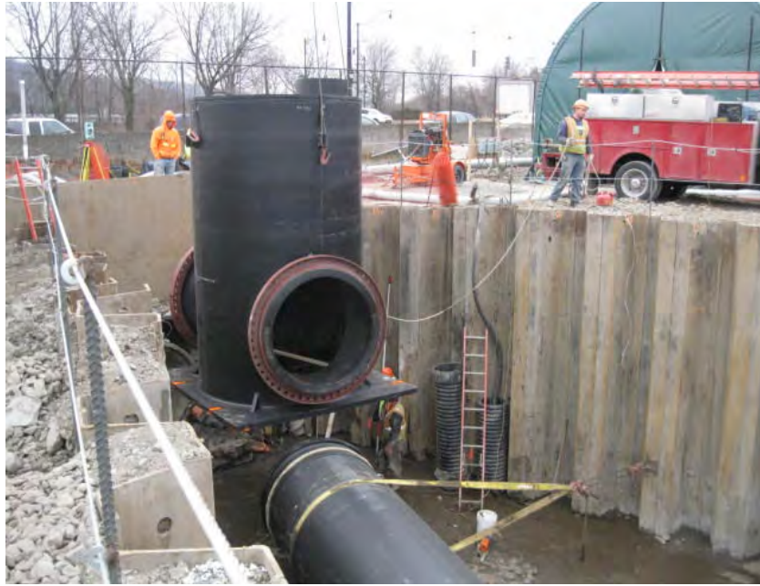
View of MH-1A being lowered into position.
