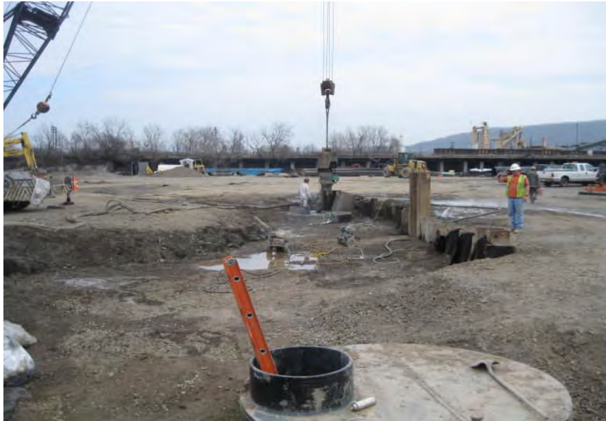
View of sheeting removal near MH-1B.
