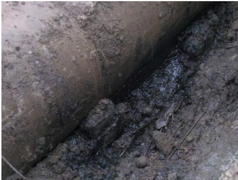
View of concrete below RCP showing water and NAPL below the RCP.
