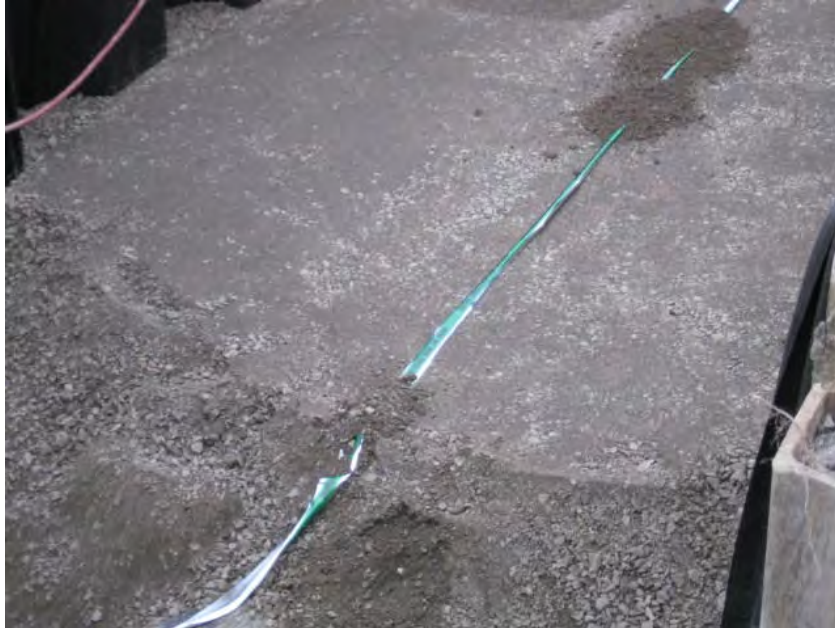
View of utility marking tape placed on top of the HDPE pipe.
