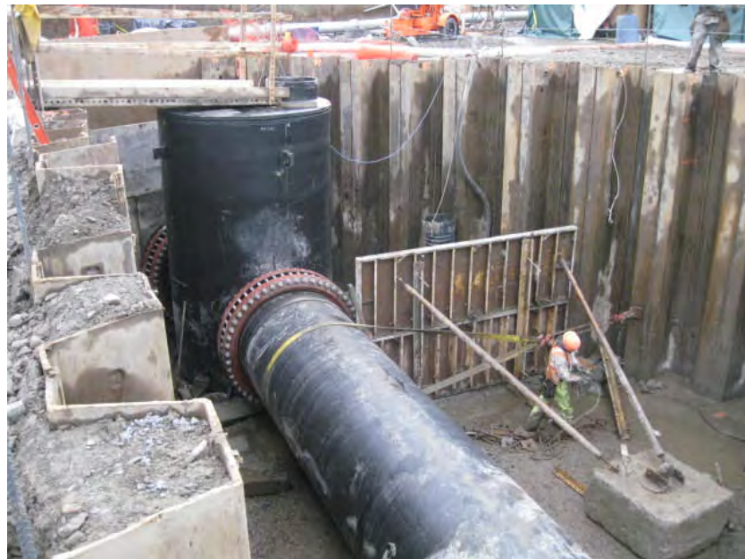
View of the northern concrete collar at MH-1A.
