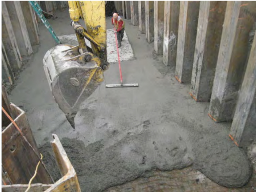
View of the emergency concrete spillway between MH-2 and MH-1C being poured.
