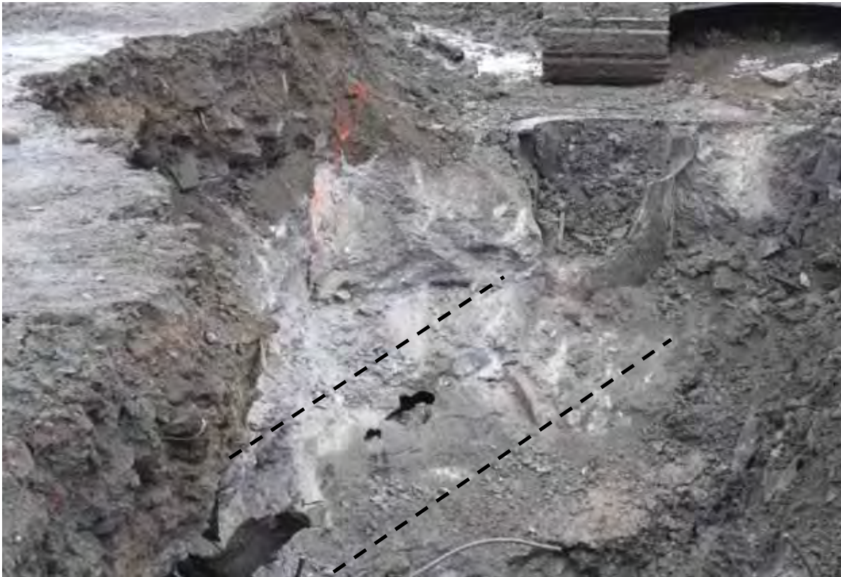
Photo #9 (2011.11.16): 30" diameter cast iron pipe, embedded in concrete with visible coal tar product present.
