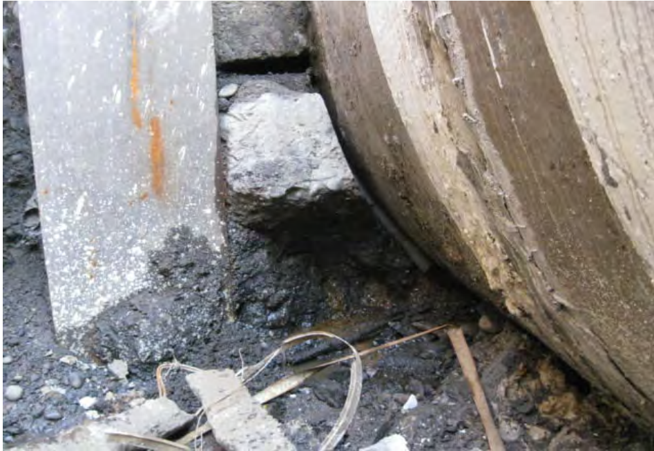
View of leak at MH-2 after hydraulic cement is applied to the leak.
