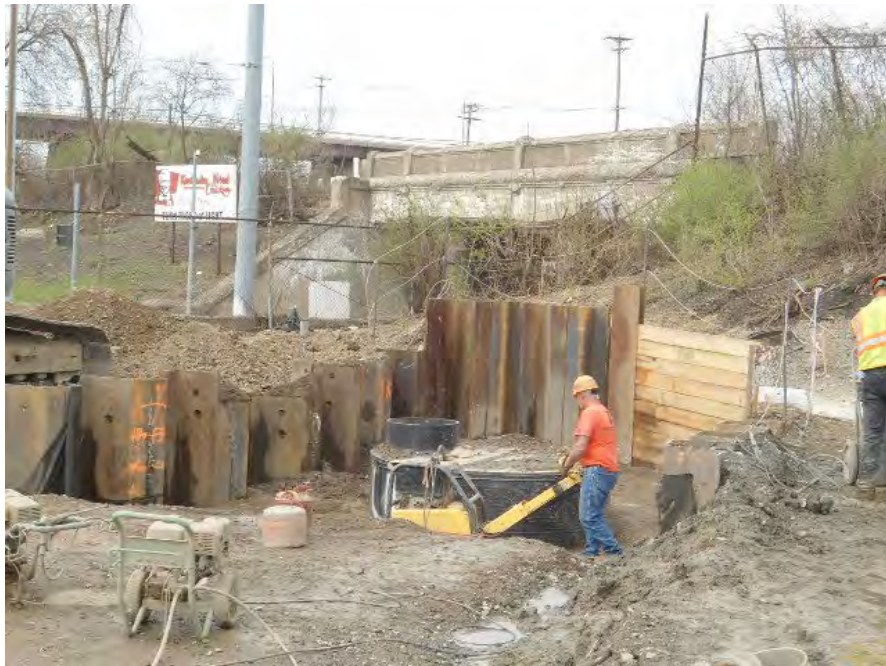
View of backfill being placed at MH-1D.
