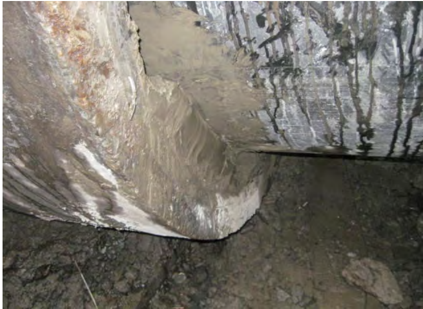
View of the hydraulic cement being installed between the HDPE pipe and the RCP at MH-1
