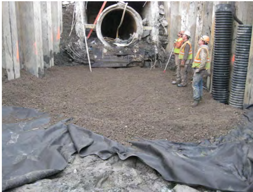
View of the second layer of Geotextile placed at MH-1A (covered with Crusher run) also showing the dewatering sumps (on the right/east) View is facing south at MH-1.
