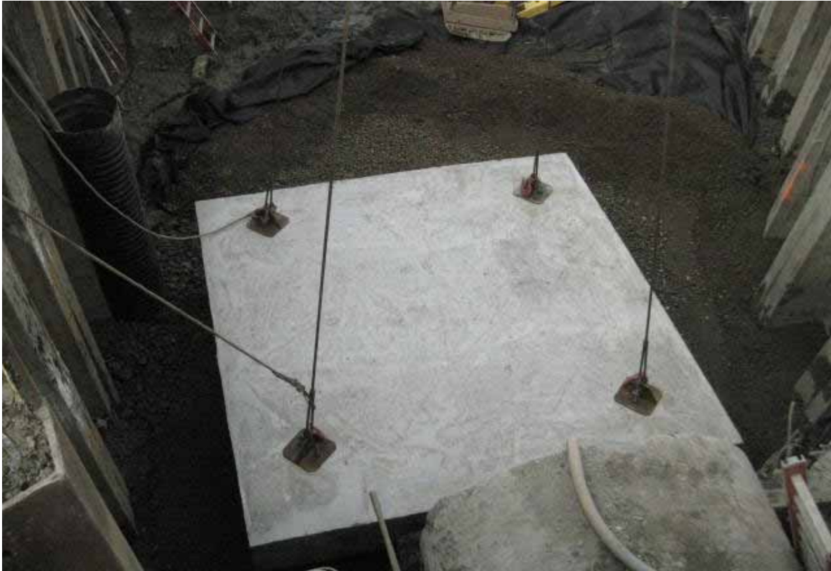
Photo #47 (2012.02.22): View of the concrete base for MH-1A being lowered into position.
