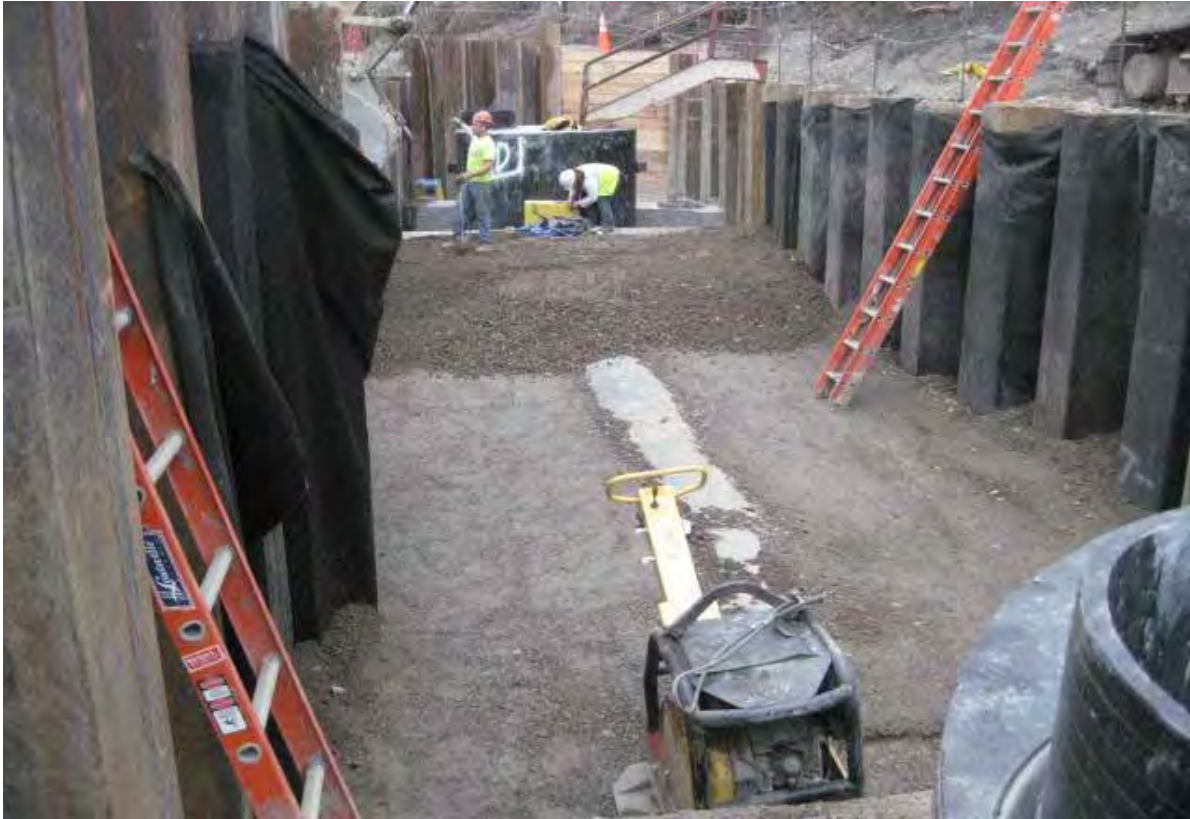
Photo #53 (2012.03.08): View of backfill between manholes MH-1C and MH-1D.
