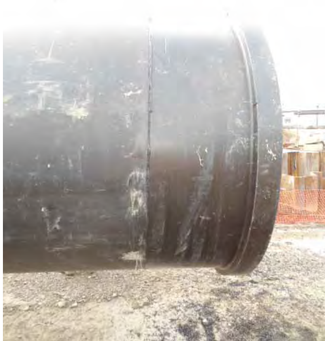
Photo #27 (2011.12.30): Facing west. A butt-fused section of HDPE and a flange.
