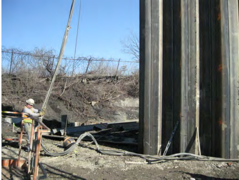
View of Tioga driving phase two area sheets at the northern end.
