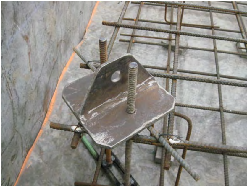
View of the lifting hooks that will be poured into the MH bases.
