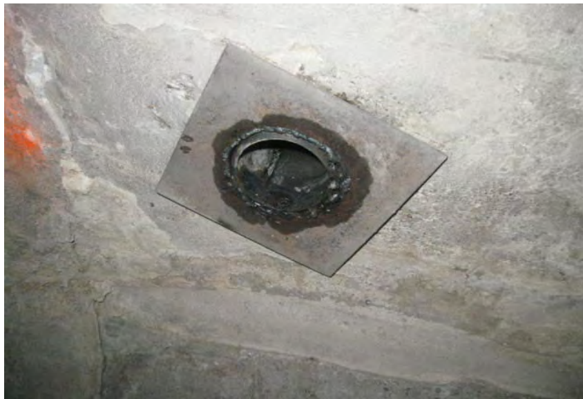
View of the grout tube installed into the RCP at MH-1. (View from inside the RCP)
