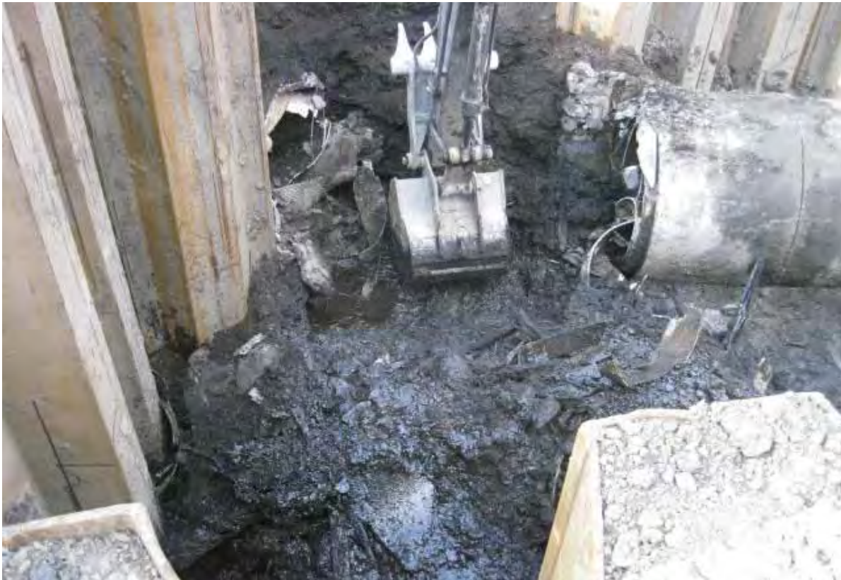
Photo #44 (2012.02.20): View of the existing RCP sewer being removed.
