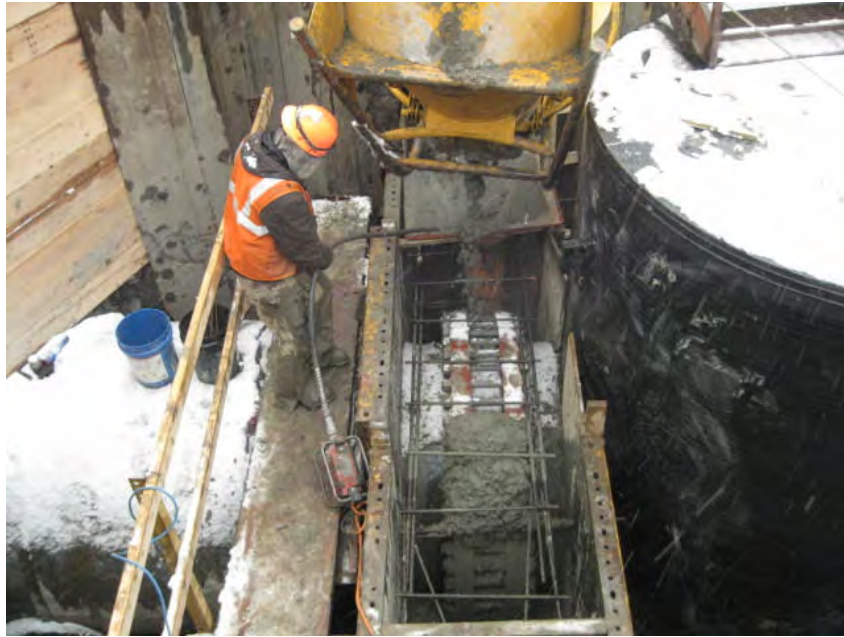
View of the northern concrete collar at MH-1D.
