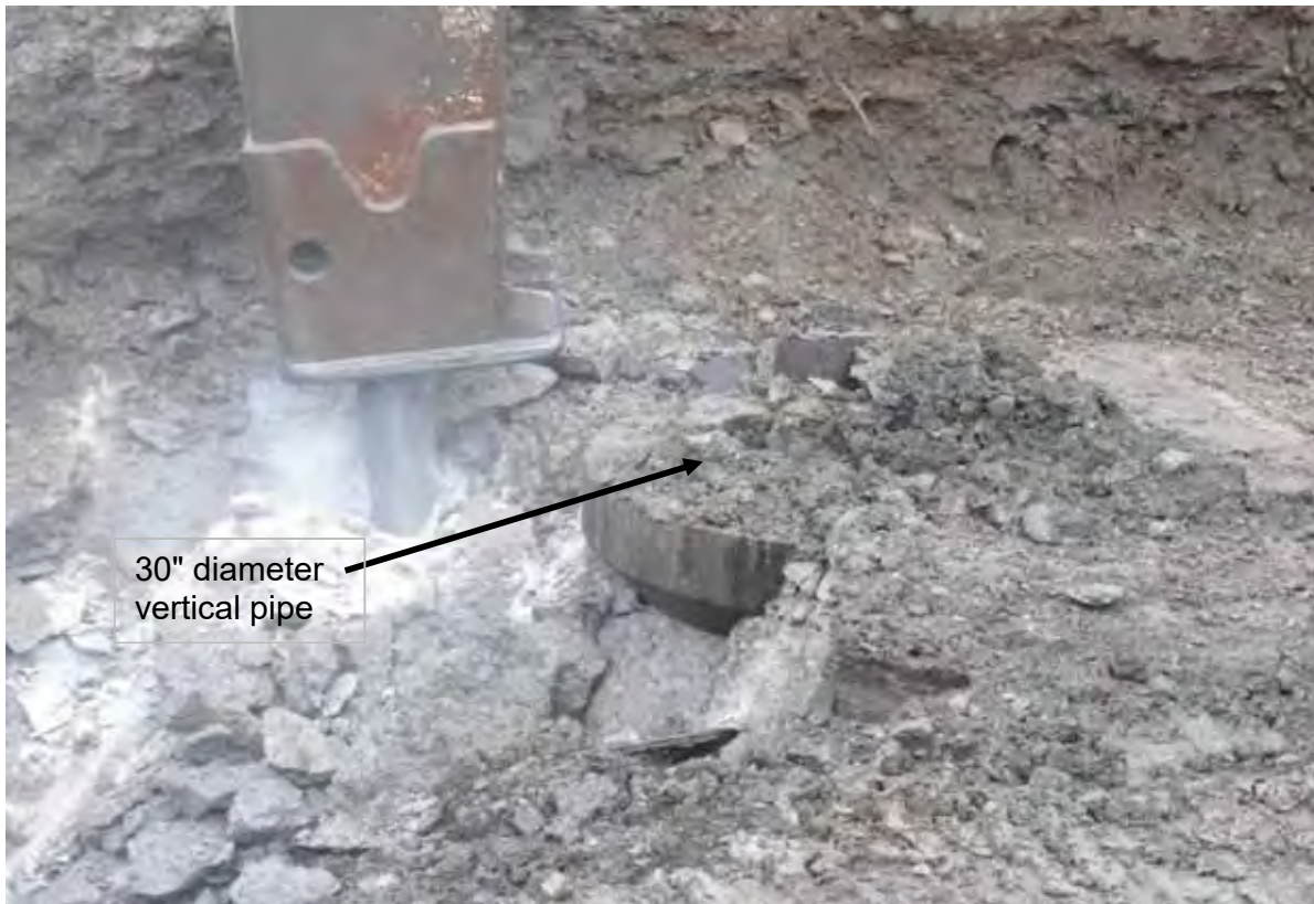
Photo #7 (2011.11.15): Gas holder NO. 4 foundation deolition, 30" diameter pipe encountered.
