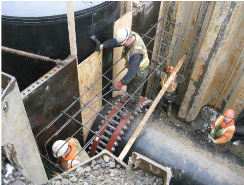
View of concrete formwork for the northern collar at MH-1B.
