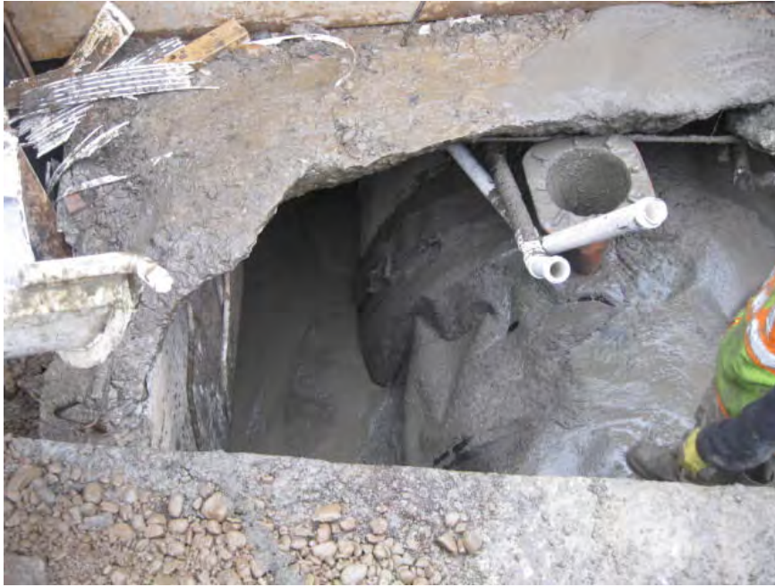
View of grout being placed inside Fernco at MH-1 and CLSM being poured outside the Fernco.
