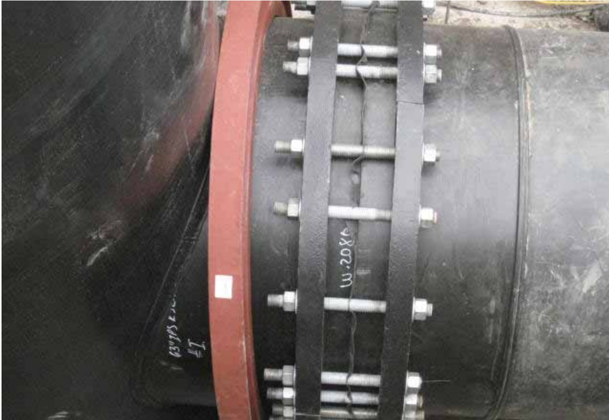
Photo #35 (2012.01.19): View of temporary connection at MH-1C (to secure HDPE for backfill). ~ ~
