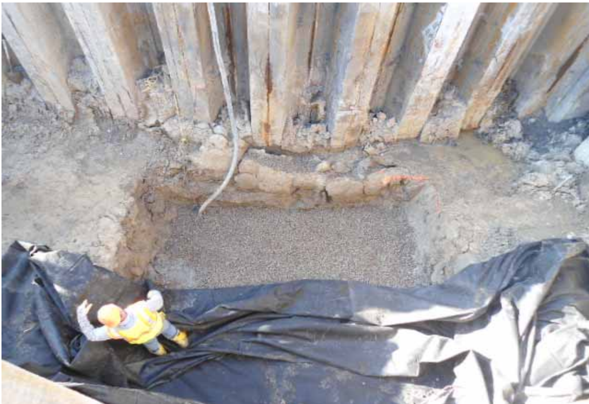
Photo #20 (2011.12.19): Facing west at the northern end of trench. Tioga placing geo-textile over #1 and #2 stone excavation for MH-1C.
