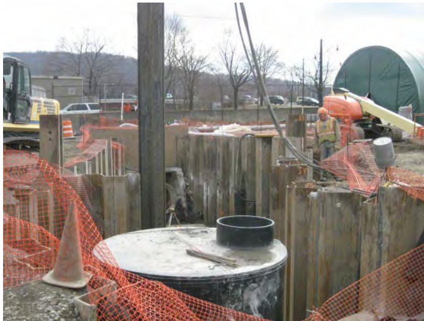
View of the Phase One sheeting being removed near MH-1B.
