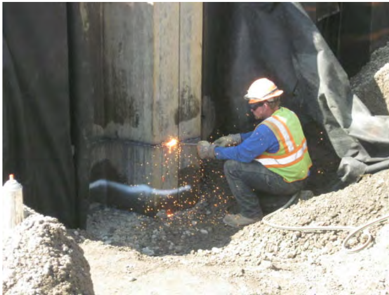
View of Tioga cutting sheets at a concrete collar.
