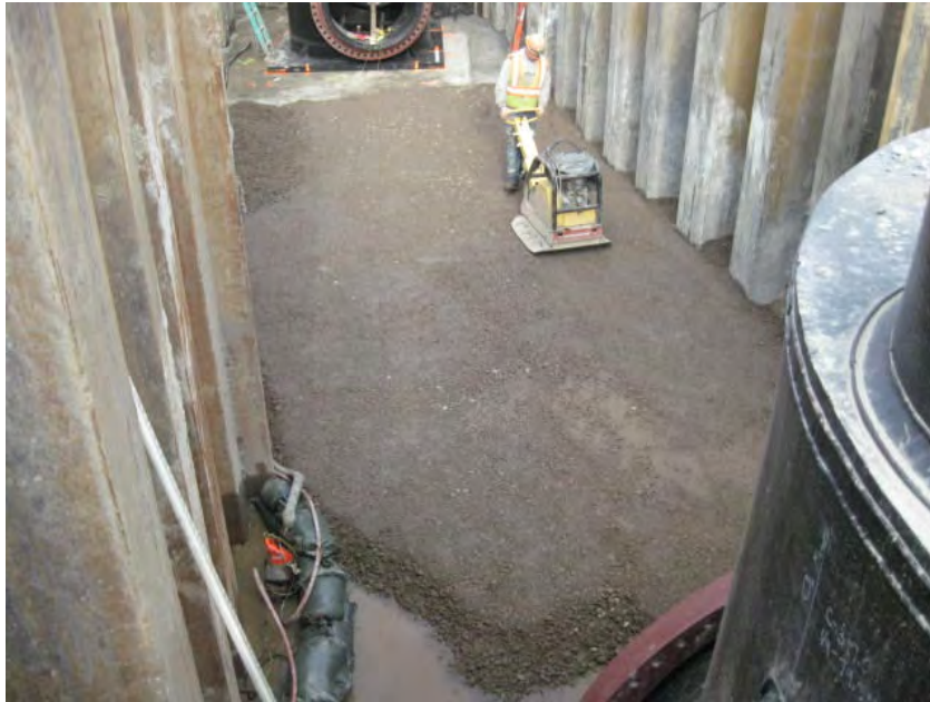
View of the crusher run sub base being compacted between MH-1C and MH-1D (looking north at MH-1D).
