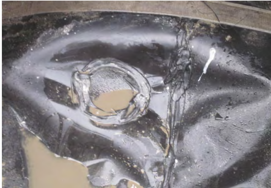
View of the grout hole after it has been welded closed.
