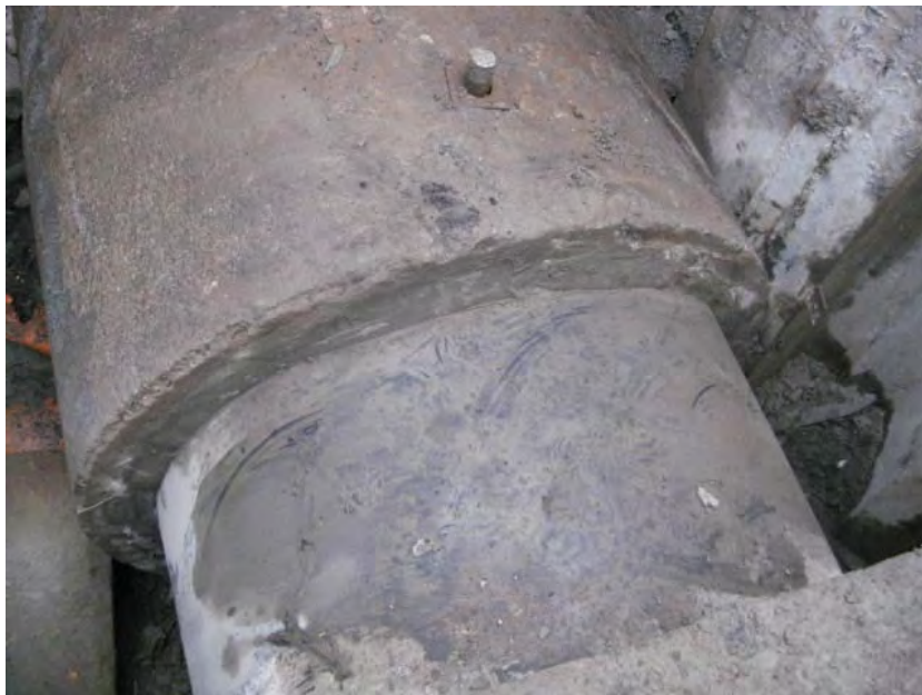
View of the slip-lined section near MH-1 showing the completed hydraulic cement and the grout tube.
