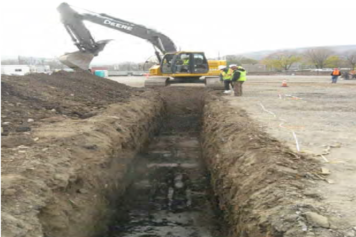
Photo #3 (2011.11.07): AECOM performing pre-trenching along the east sheeting alignment.
