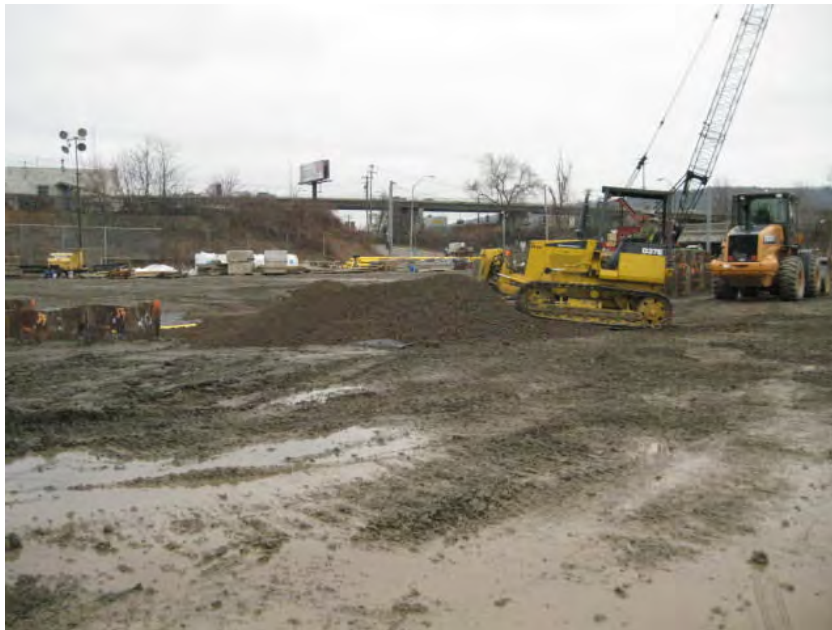
View of AECOM personnel placing crusher run stone for the access road across the phase one area (facing west).
