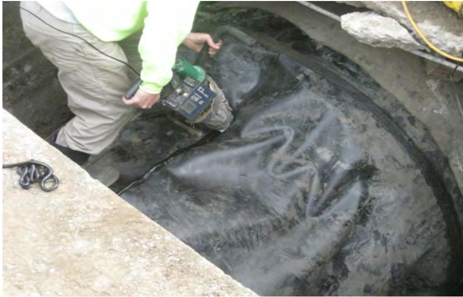
View of Chenango welding the HDPE seam on the Fernco connector.
