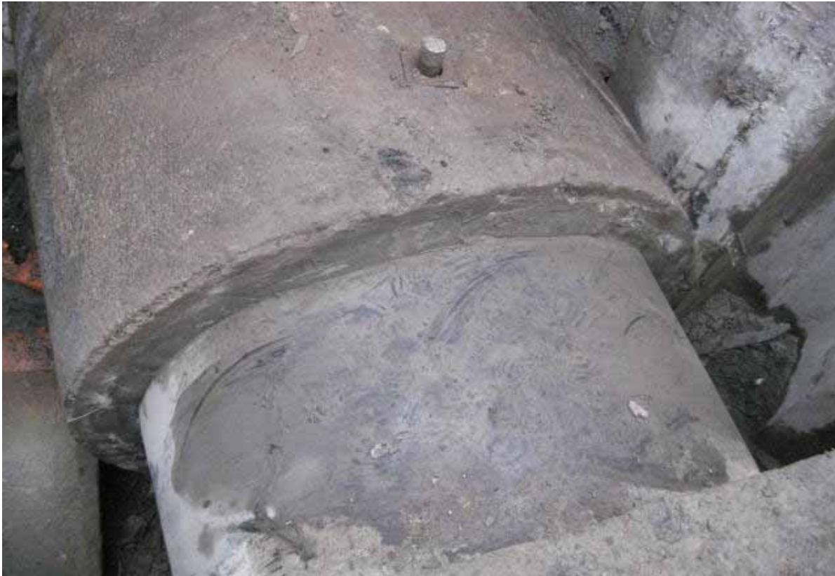
Photo #51 (2012.03.01): View of the slip-lined section near MH-1 showing the completed hydraulic cement and the grout tube.
