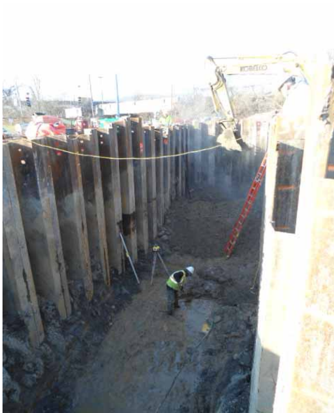
Photo #19 (2011.12.13): Facing north. Trench excavation at northern end. AECOM performing dewatering activities in base of trench.
