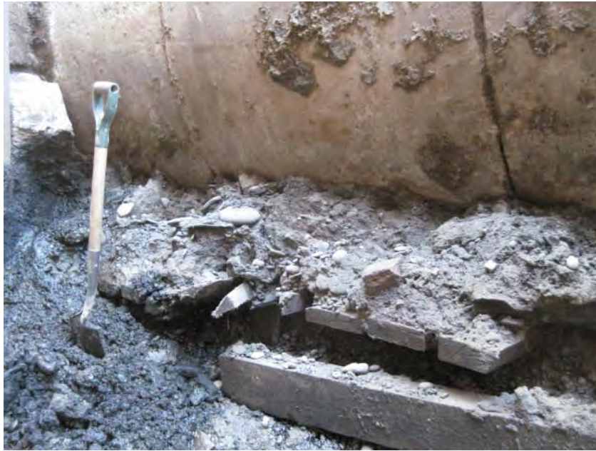
View of the wood “cribbing” used to support the existing sewer on the north end.
