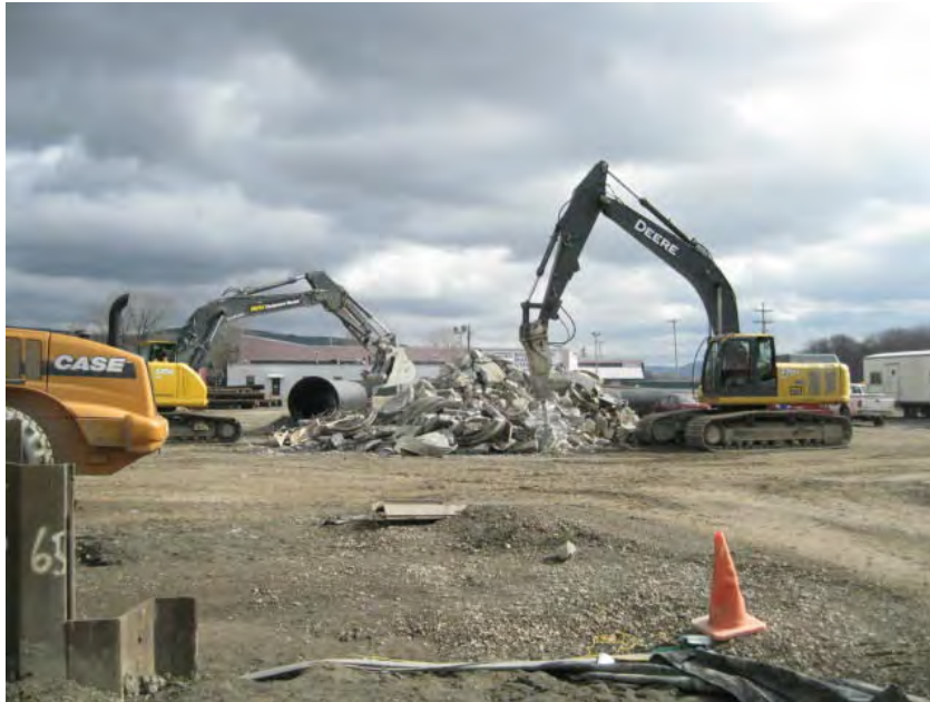
View of the RCP sections being downsized for offsite disposal.
