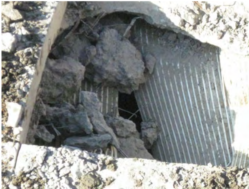
View of access hole cut through the top of the RCP pipe. The Danby liner is visible below the concrete.
