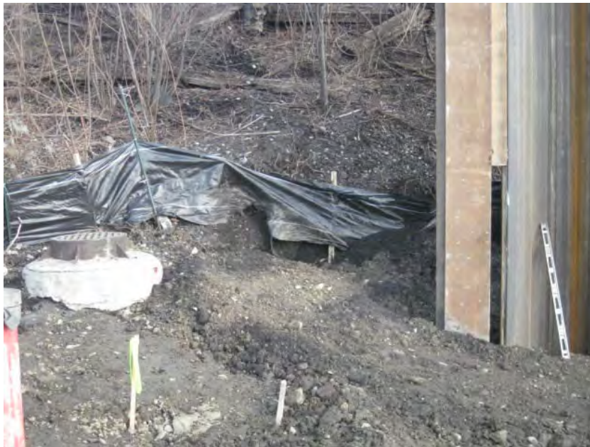
View of area around MH-2 where obstructions encountered (H-pile and sheeting are observed on right).
