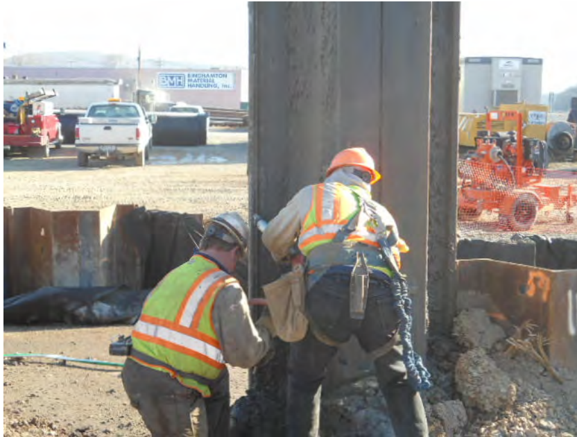
View of Tioga cleaning and caulking sheets.
