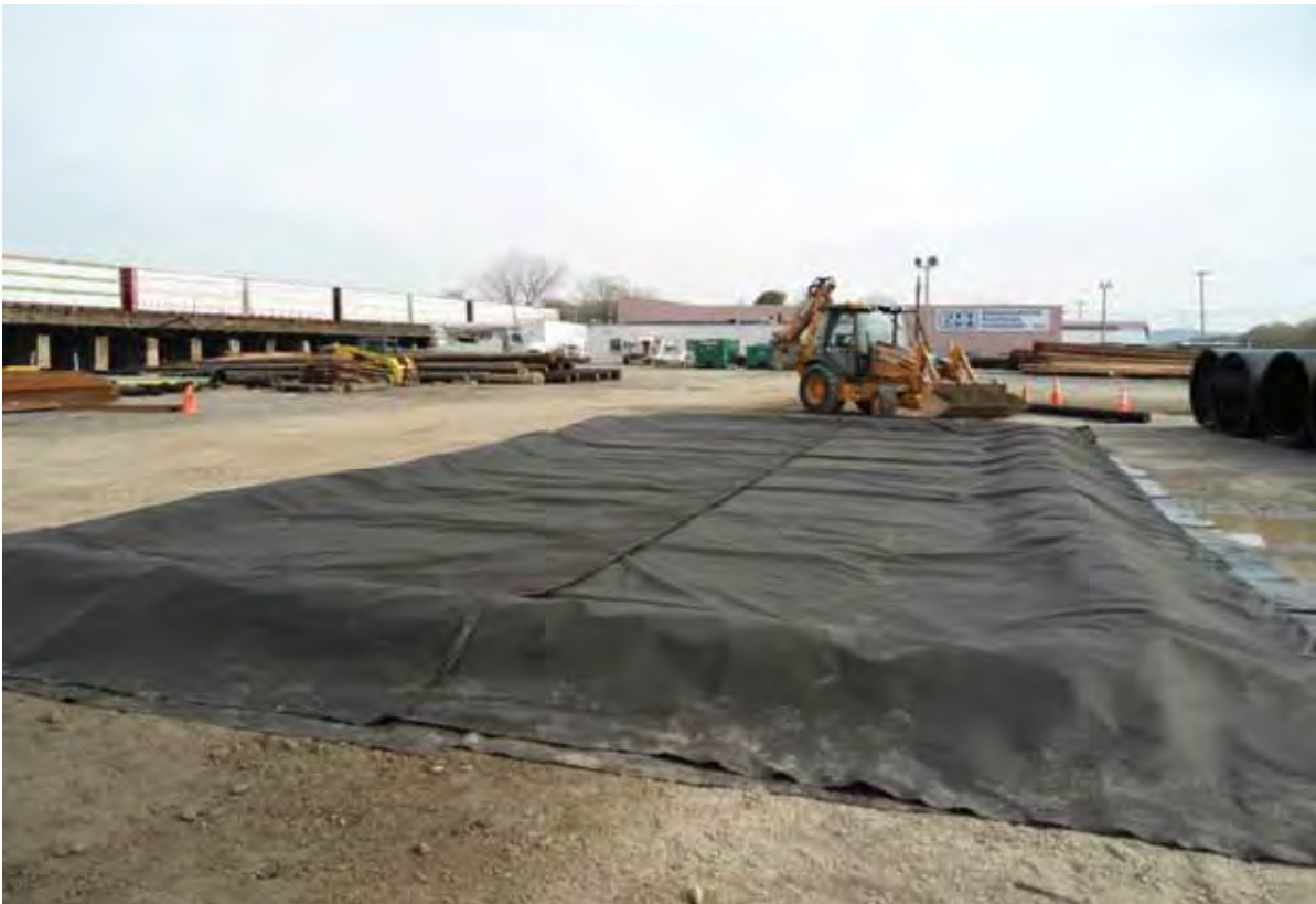
Photo #2 (2011.11.03): Looking east. Decontamination Pad Liner system (non-woven-geotextile HDPE liner)
