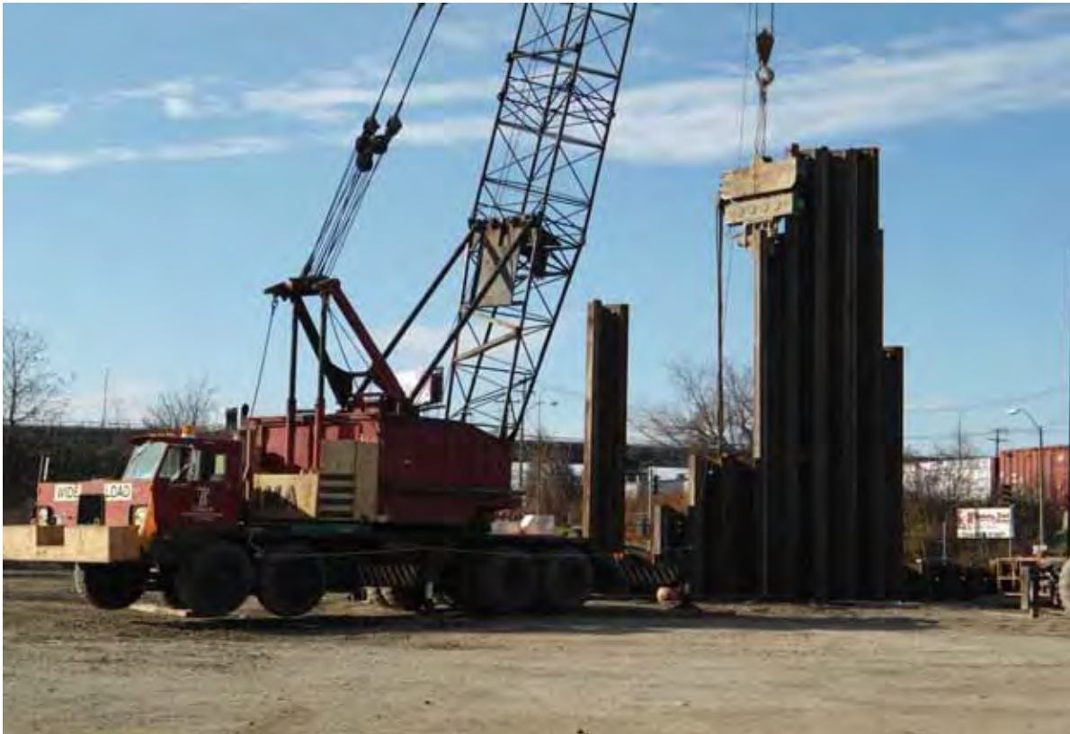
Photo #11 (2011.11.21): Facing northwest. Sheetting installation along east alignment.
