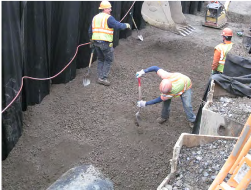
View of backfill being placed on top of the HDPE pipe.
