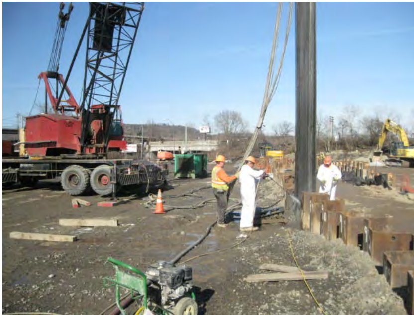
View of Tioga personnel removing sheets from the center of the phase one area. (facing north)
