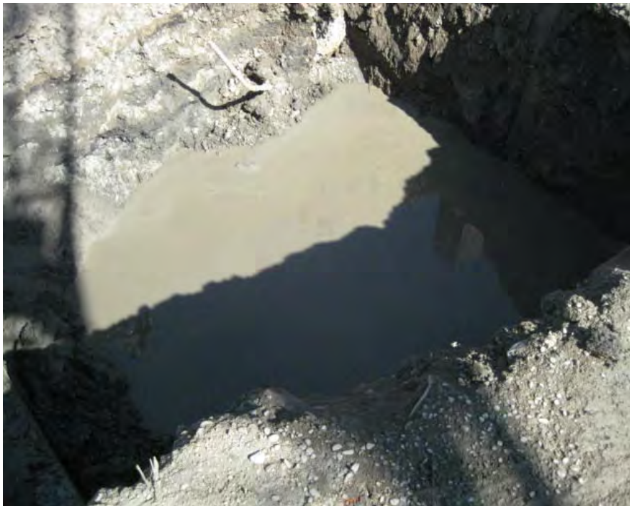
View of existing sewer after CLSM has been poured.
