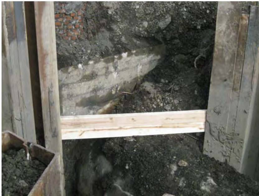
View of the wood lagging being installed at the northern end.
