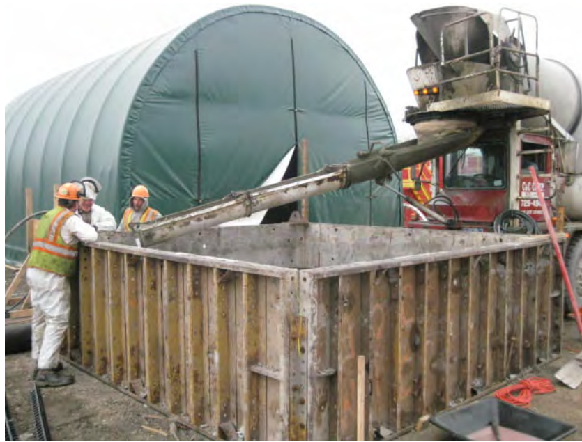
View of manhole MH-1A base being poured.
