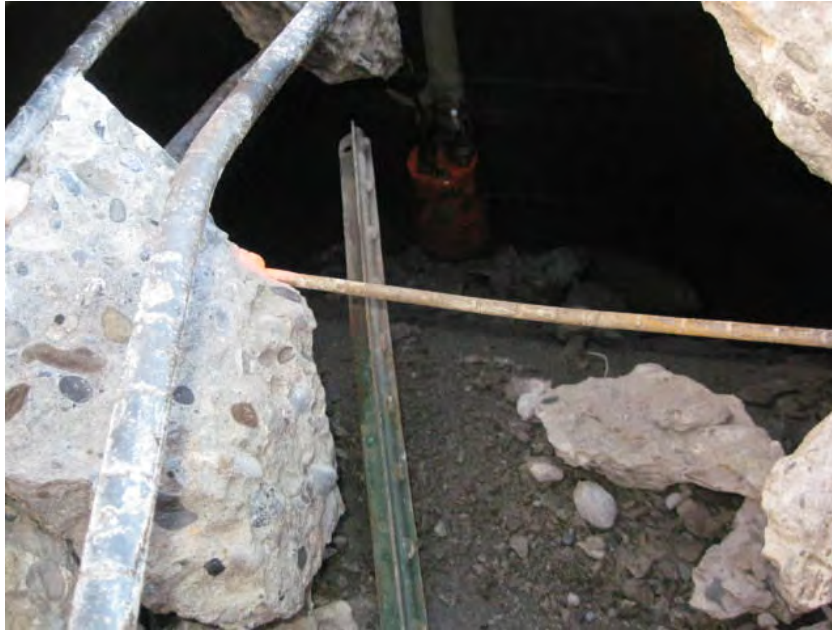
View of the dewatering process from inside the pipe chase (the existing sewer is visible in the foreground)
