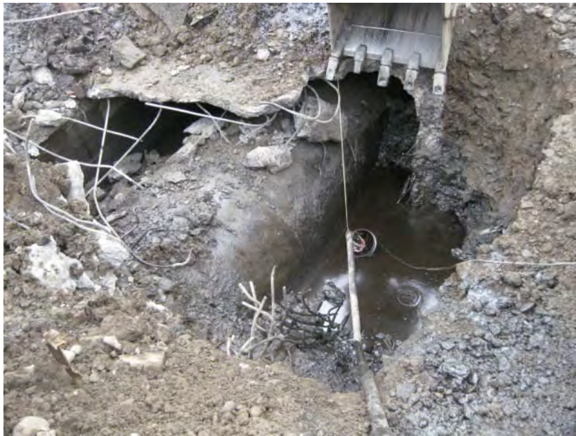
View of concrete pipe chase and the exposed RCP sewer.
