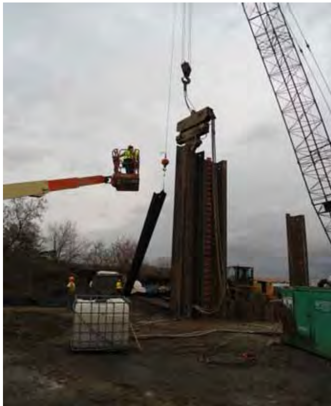
Photo #8 (2011.11.15): Installing sheets along west sheting alignment.
