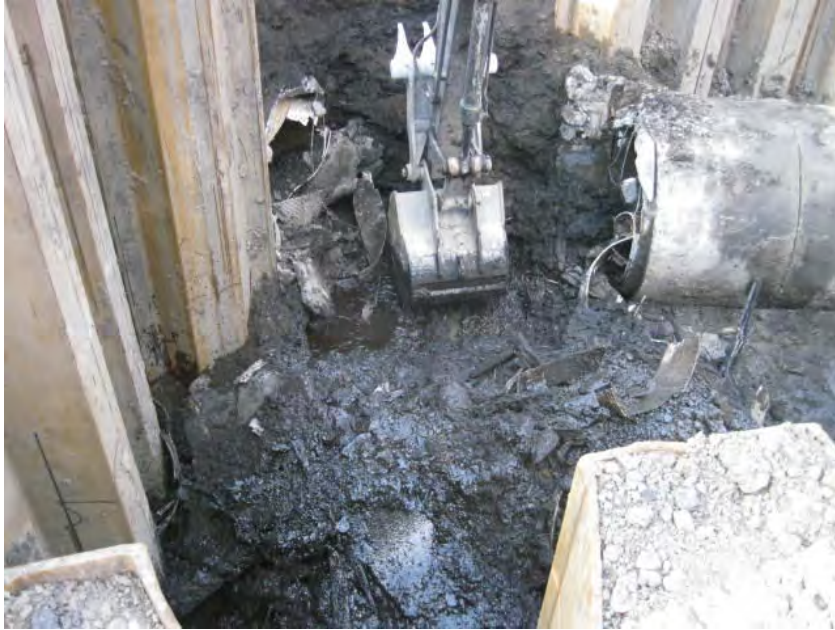
View of the existing RCP sewer being removed.
