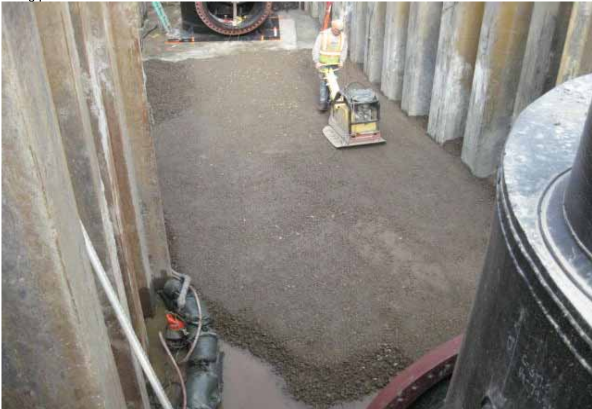
Photo #46 (2012.02.22): Looking north at MH-1D. View of the crusher run sub base being compacted between MH-1C and MH-1D.
