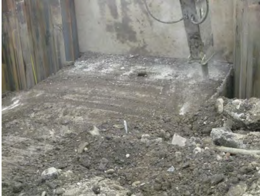
View of concrete pipe chase with hole broken through the top.
