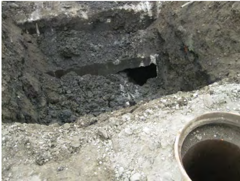
View of test pit near manhole MH1-B showing northern end of the pipe chase.
