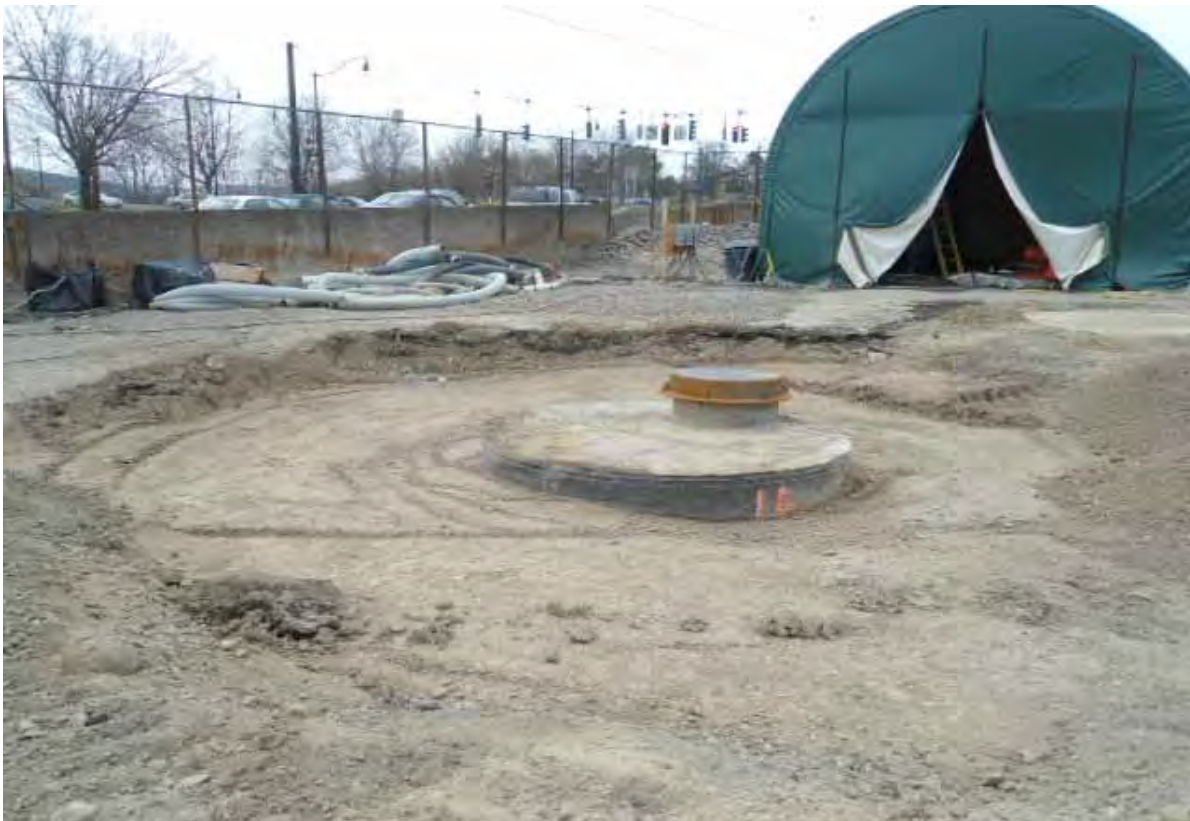
Photo #58 (2012.03.23): View of the southern end of the site at MH-1A after sheetpiling was removed. concrete was poured outside the Fernco.
