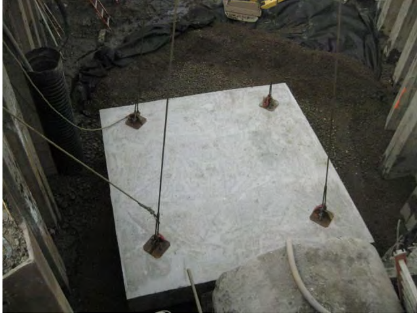
View of the concrete base for MH-1A being lowered into position.
