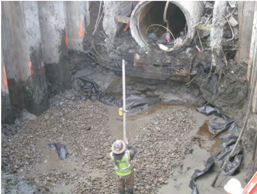
View of the stone at MH-1A showing the existing RCP at MH-1.
