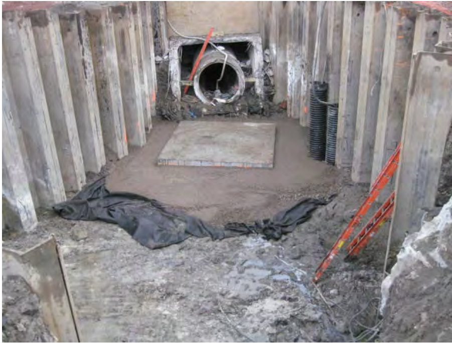
View of the concrete base for MH-1A.
