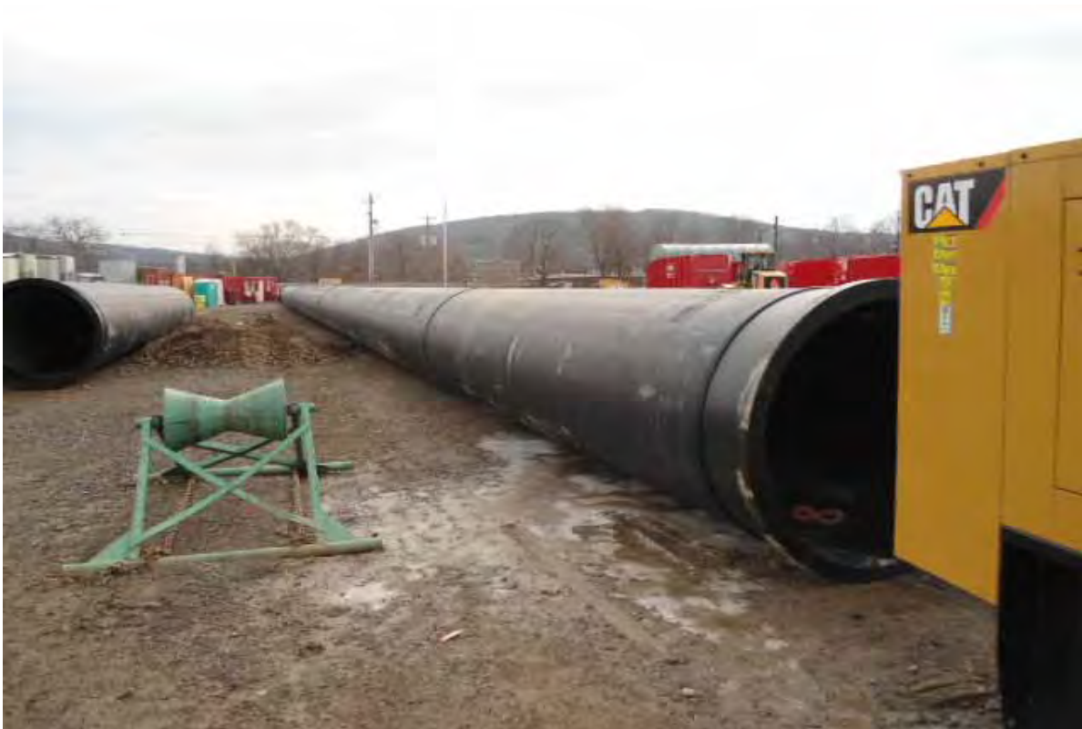
Photo #26 (2011.12.30): Facing southwest. A completed butt-fused section of HDPE piping.
