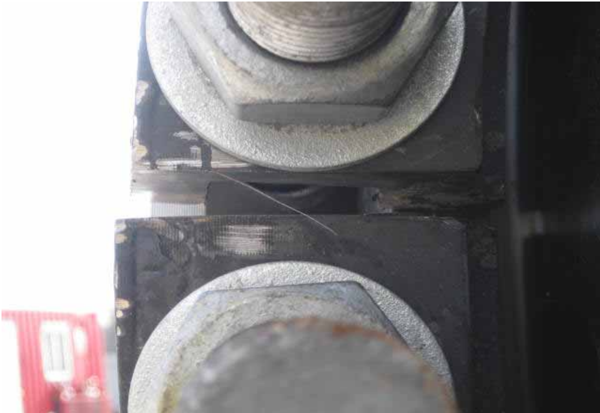
Photo #33 (2012.01.16): View showing a split backer ring installed on the pipe.
