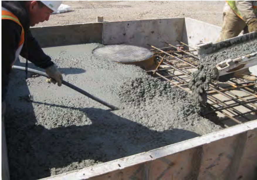
View of concrete being poured for MH-1A.
