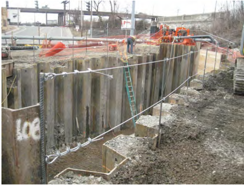
View of the safety railing being installed around the northern sheeting.
