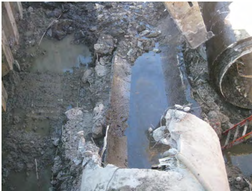
View of the concrete “cradle” below the RCP sewer at the south end. Remnants of the concrete pipe chase and the RCP are visible on both sides of the cradle. NAPL is also visible in the cradle itself.
