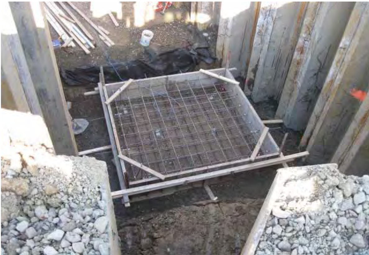
Photo #30 (2012.01.11): View of forms and re-bar for the base of MH-1B.
