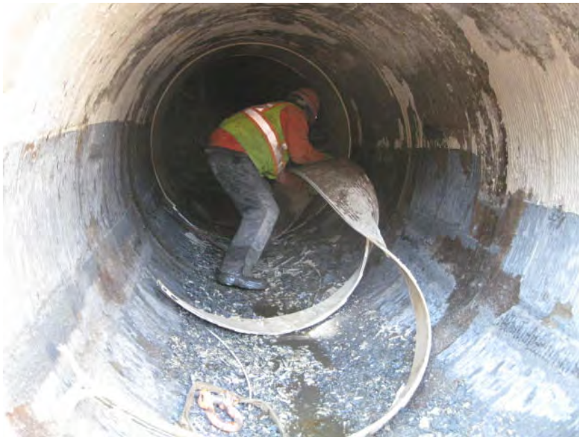
View of the Danby liner being removed. Note the two different grout types used behind the liner (white grout on the top and gray grout on the bottom)
