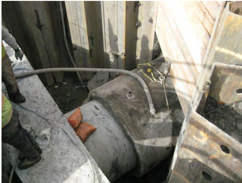
View of MH-2 prior to grouting.
