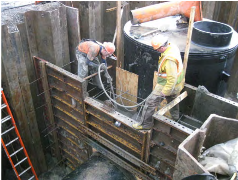
View of the pouring of concrete at MH-1B.
