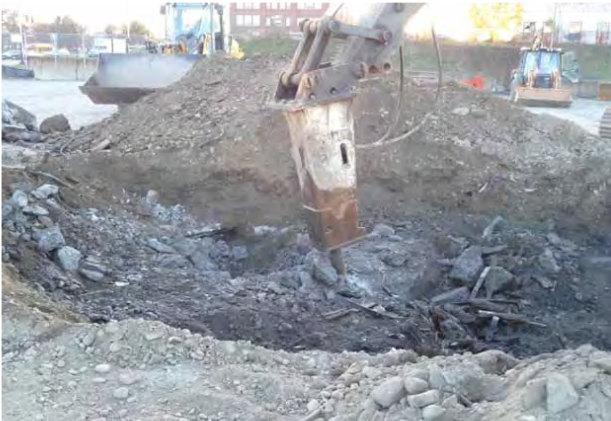
Photo #6 (2011.11.09): North edge of Gas holder No. 4 foundation demolition.
