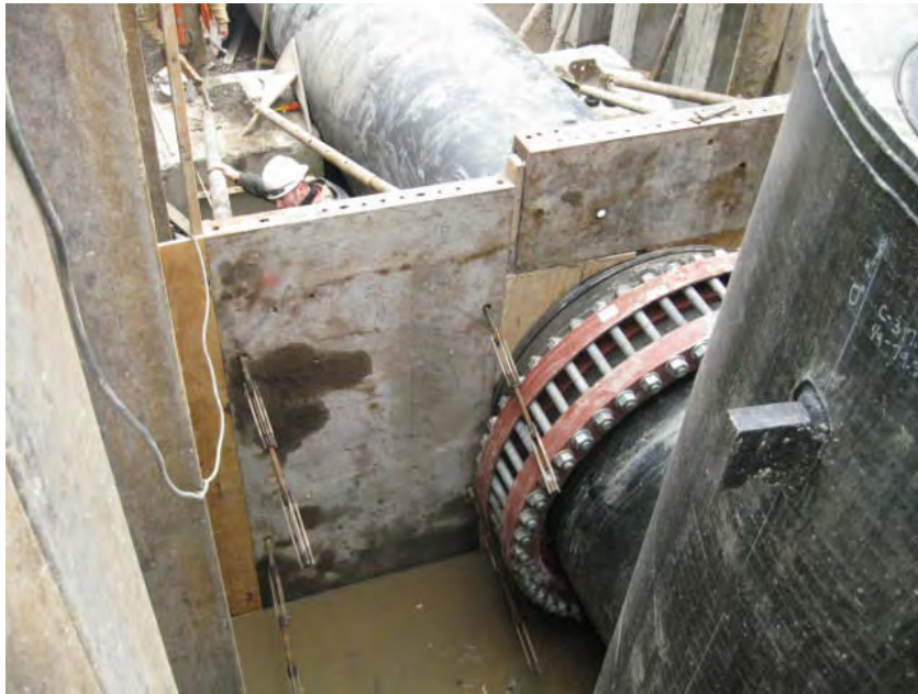
View of the concrete forms being placed at the upstream concrete collar of MH-1C.
