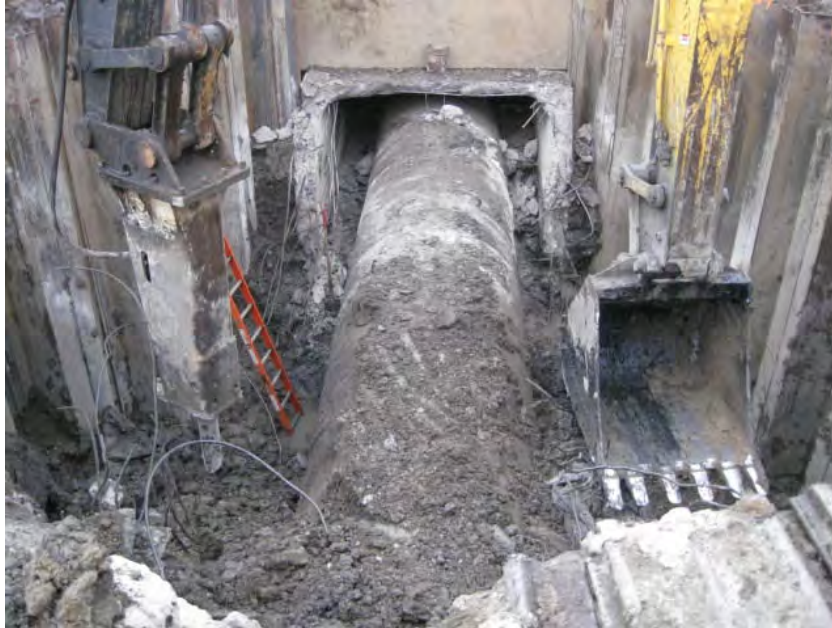
View of the RCP near manhole MH-1 after pipe chase removal.
