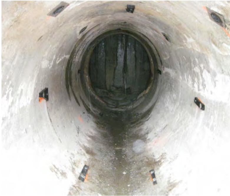
View of the HDPE spacers installed inside the RCP to center the HDPE pipe.
