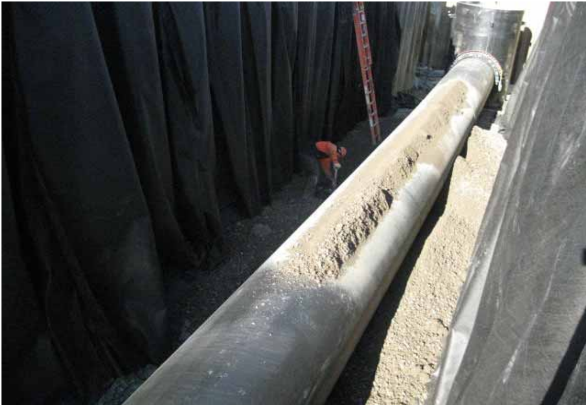
Photo #36 (2012.01.19): View of Tioga placing the first lift of crusher run stone around the HDPE pipe.
