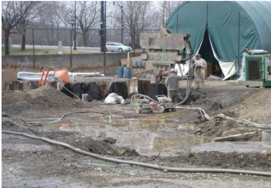
View of sheeting removal near MH-1A.
