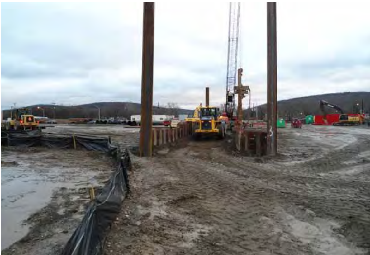
Photo #12 (2011.11.23): Facing south. Backfilling and rough grading pipe trench alignment.
