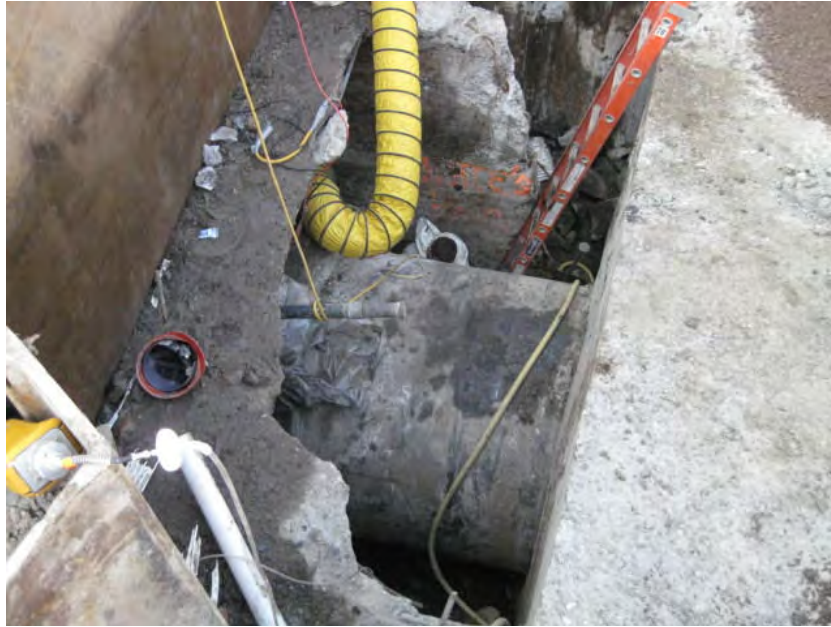
View of Tioga removing debris from the pipe chase at MH-1.
