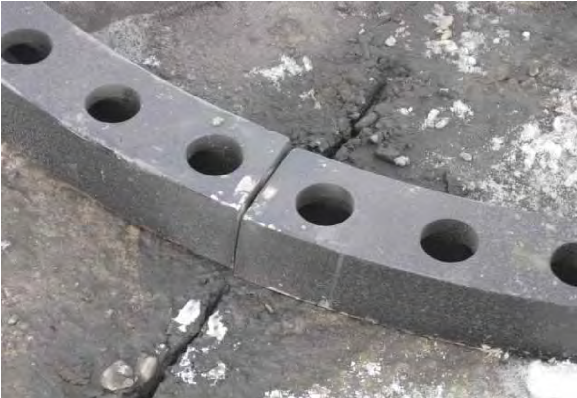
Photo #32 (2012.01.16): View of a backer ring cut in half to fit over the HDPE ring.
