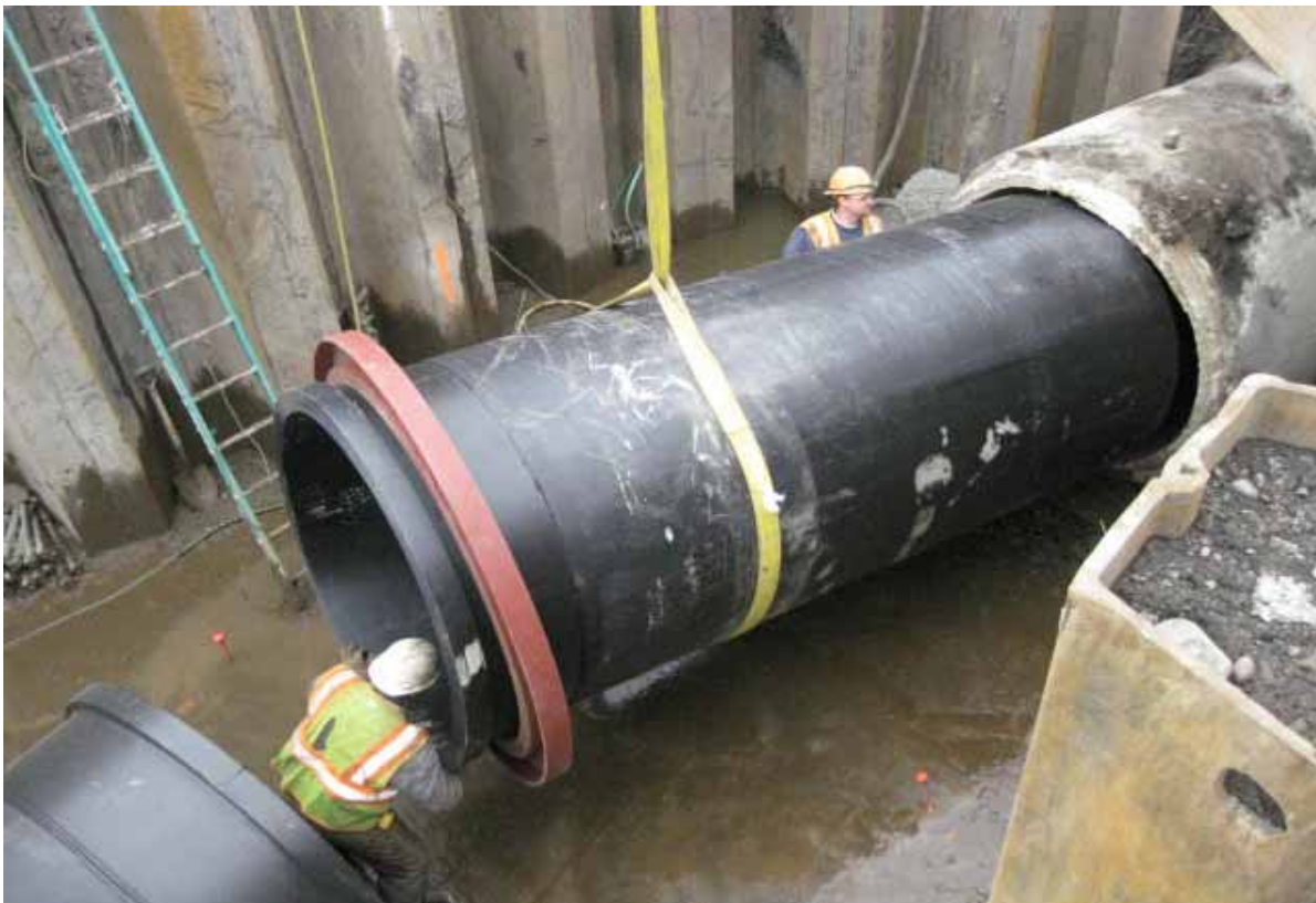
Photo #48 (2012.02.27): View of the HDPE pipe being slipped inside of the existing RCP sewer at MH-2.
