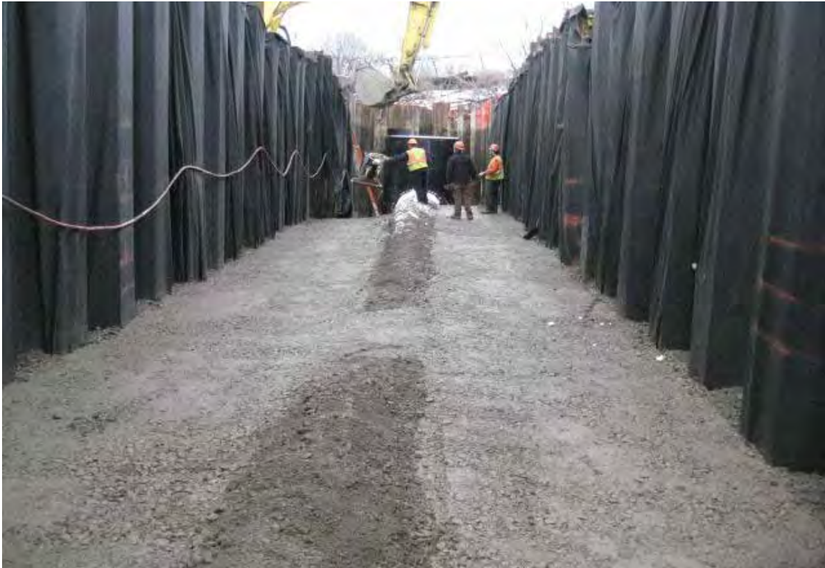
Photo #37 (2012.01.23): Facing north. View of backfill being placed on top of HDPE pipe. Geotextile ~ fabric is visible on each side of the trench.
