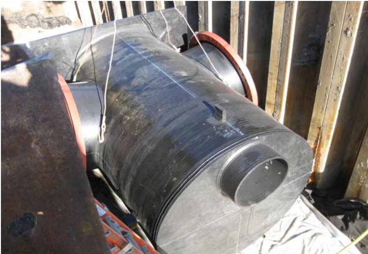
Photo #2 (2012.01.09): View of MH-1C being lowered into position.
