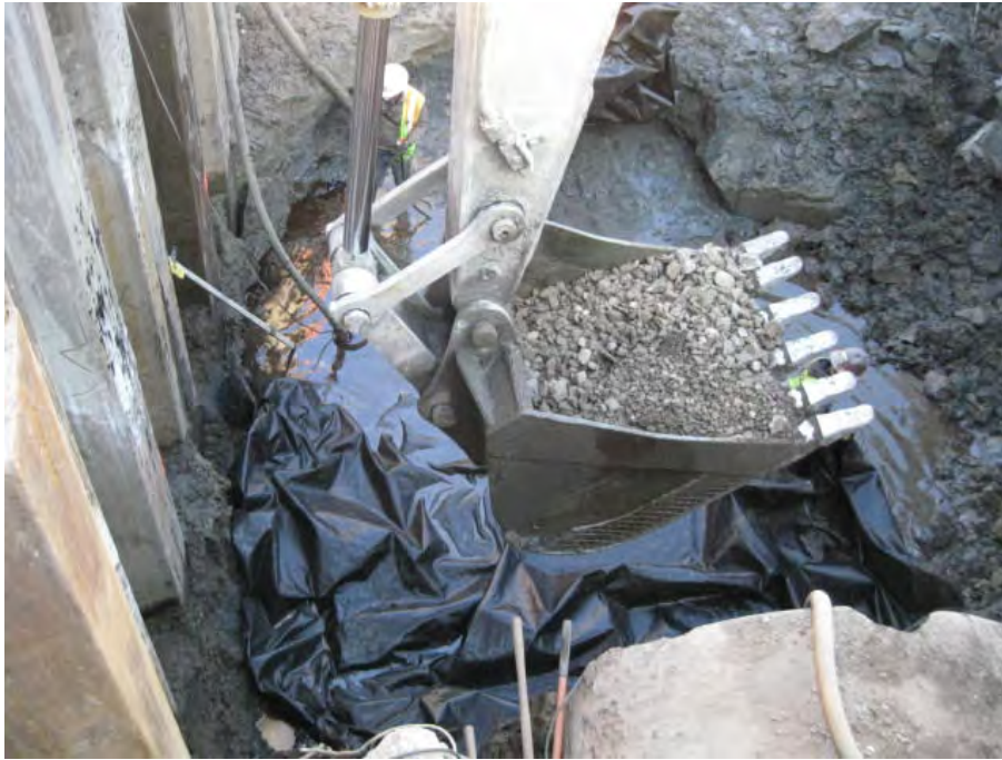
View of 3-4" diameter stone being placed to form the type 2 sub base at MH-1A.
