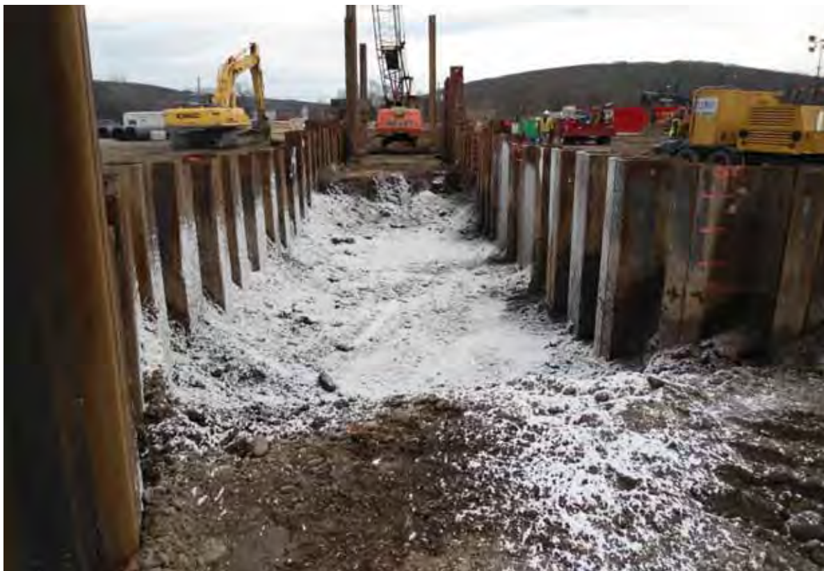
Photo #14 (2011.11.28): Facing south. Application of Rusmar foam.
