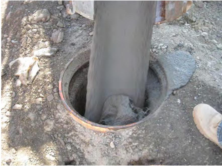
View of CLSM being poured into the former MH-1B.
