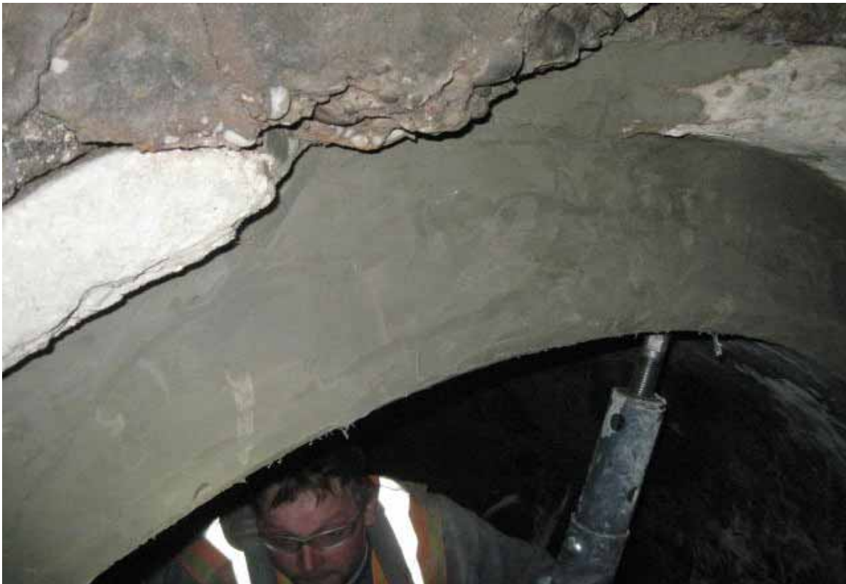
Photo #50 (2012.02.28): View of the HDPE pipe/RCP after the hydraulic cement has been installed. sewer at MH-2.
