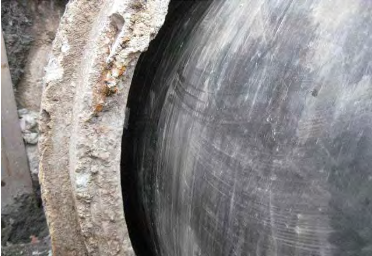
Photo #49 (2012.02.27):View of the spacing between the HDPE and the existing RCP.
