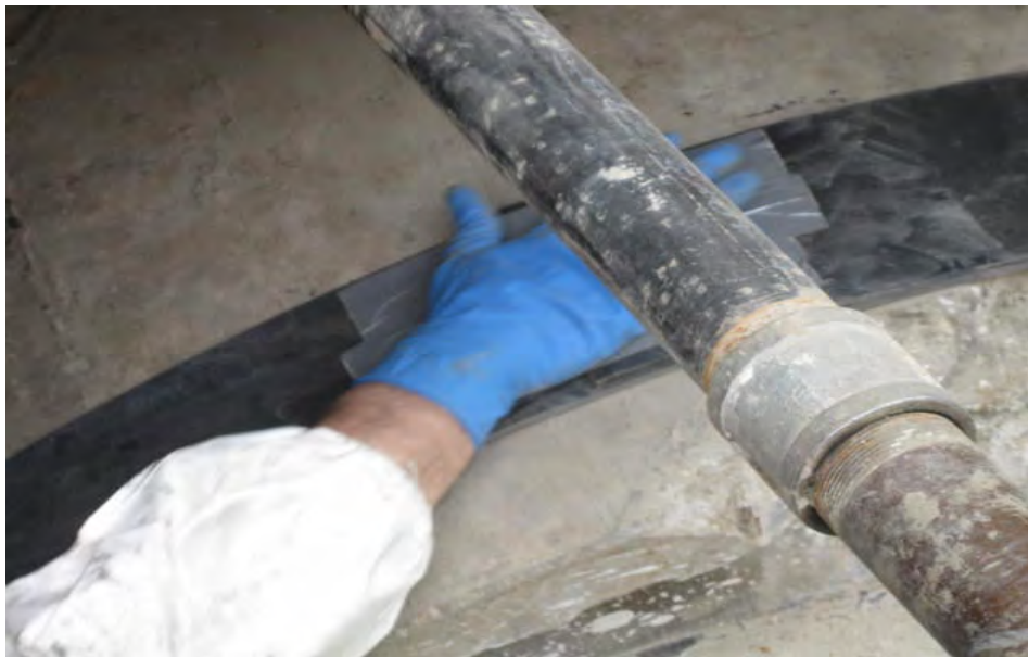
View of Chenango installing the Viton seal for the Fernco connector.
