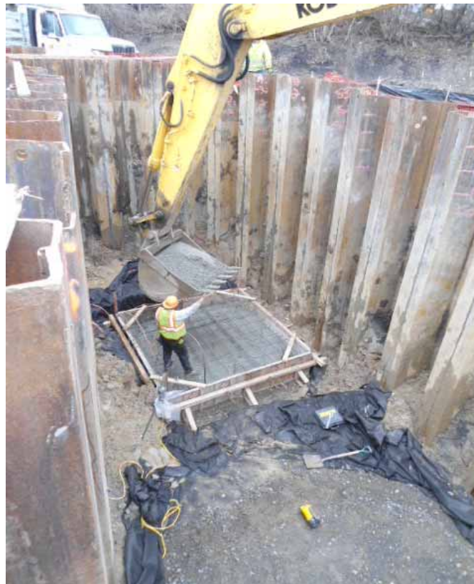
Photo #22 (2011.12.22): Facing north. AECOM and Tioga placing concrete in form for MH-1C.
