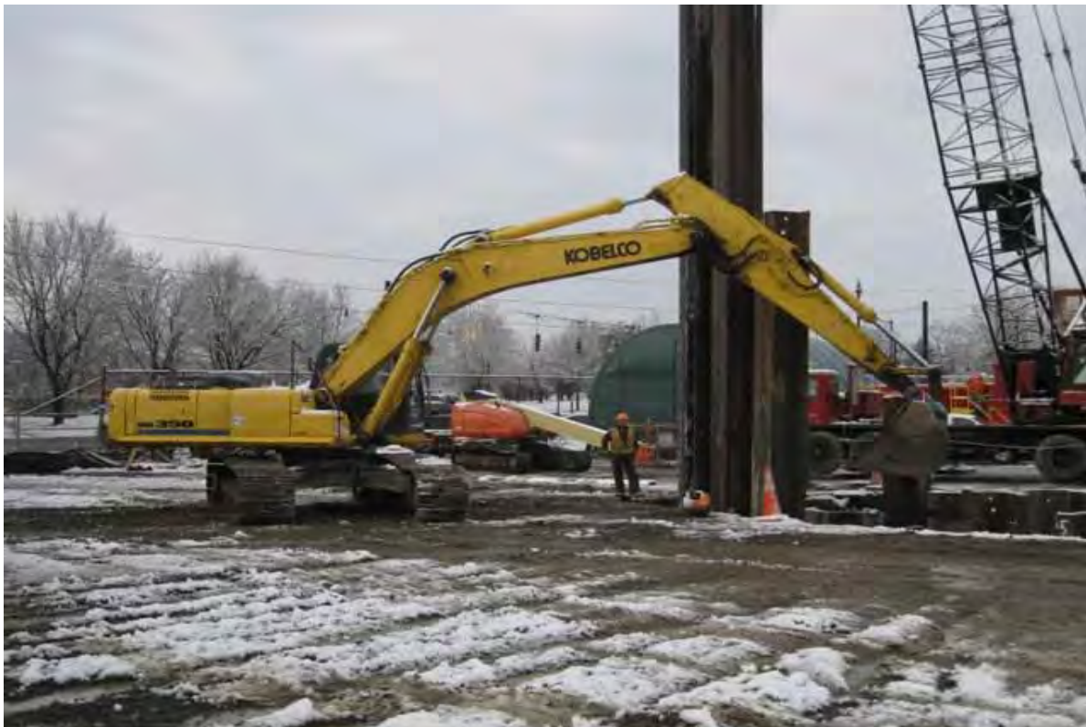
Photo #18 (2011.12.08): Facing south west. Final sheets being installed at south end of trench alignment.
