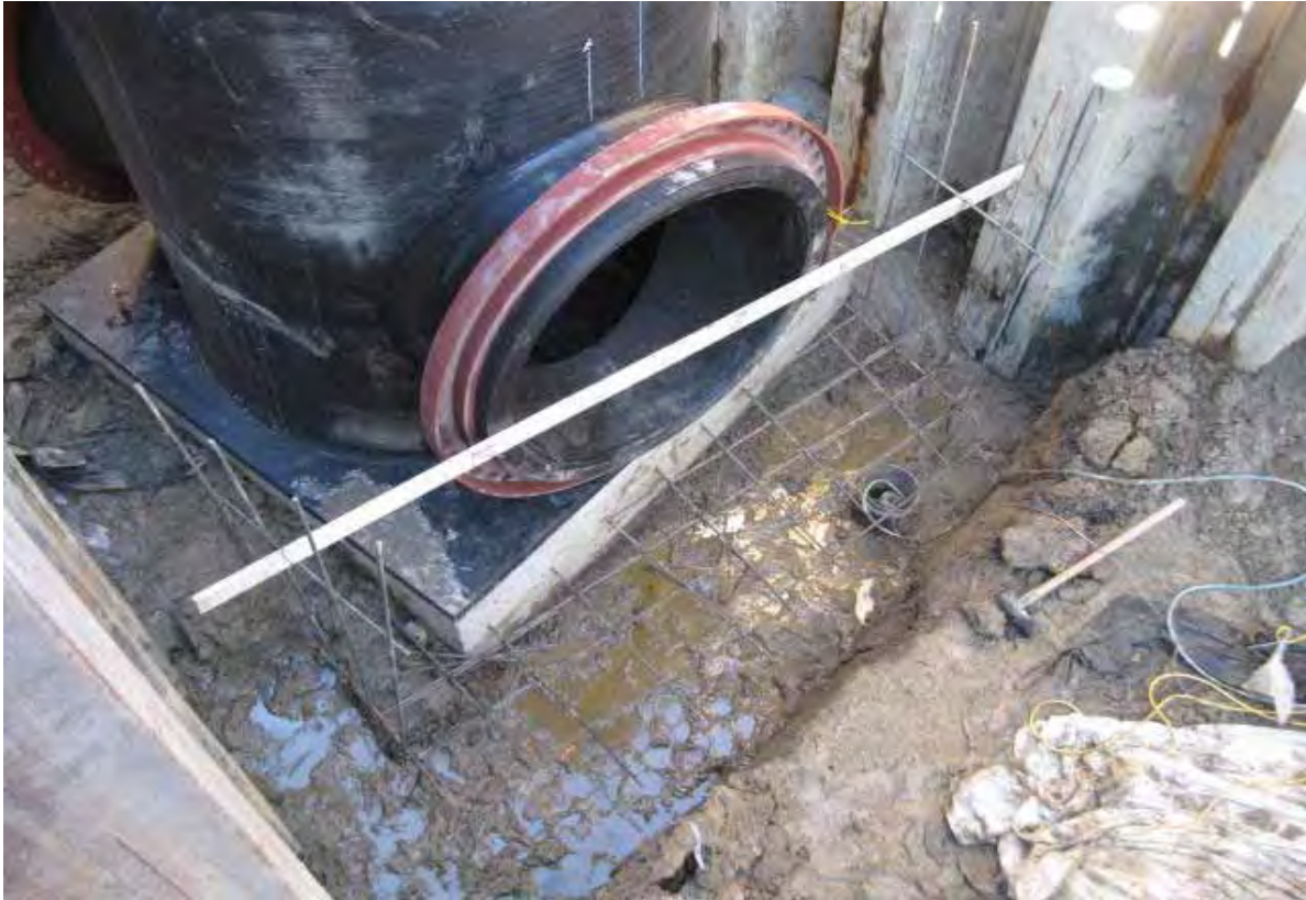
Photo #29 (2012.01.09): View of re-bar being placed for the southern collar at MH-1C.
