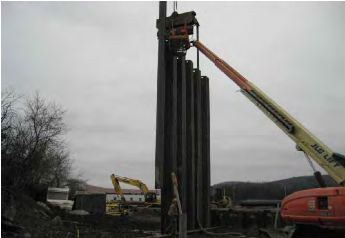
Photo #42 (2012.02.02): Facing east. View of Tioga personnel driving the northern section of the phase two sheets.
