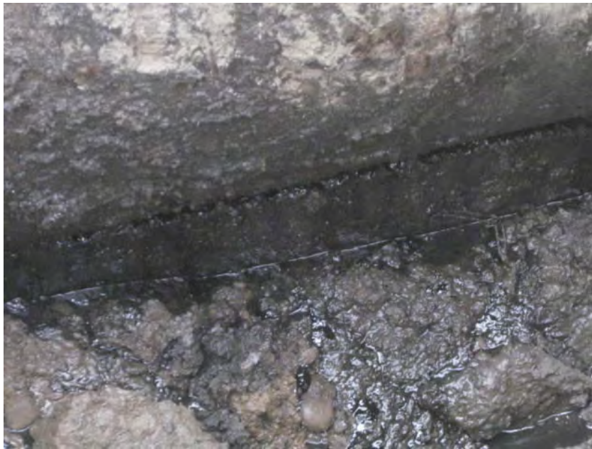
View of concrete below RCP showing water and NAPL below RCP.
