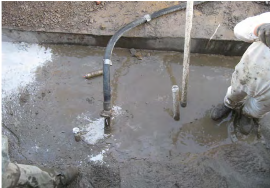
View of grouting of the slip-lined section of HDPE pipe at MH-1.
