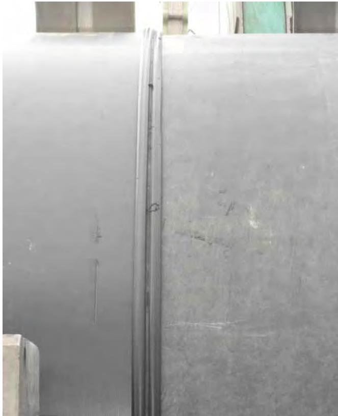
Photo #24 (2011.12.27): Facing west. A completed butt fusion of the south flange and an approximately 54-foot section of HDPE.
