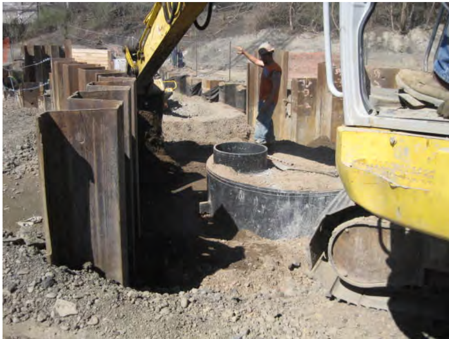
View of backfill being placed near MH-1C.
