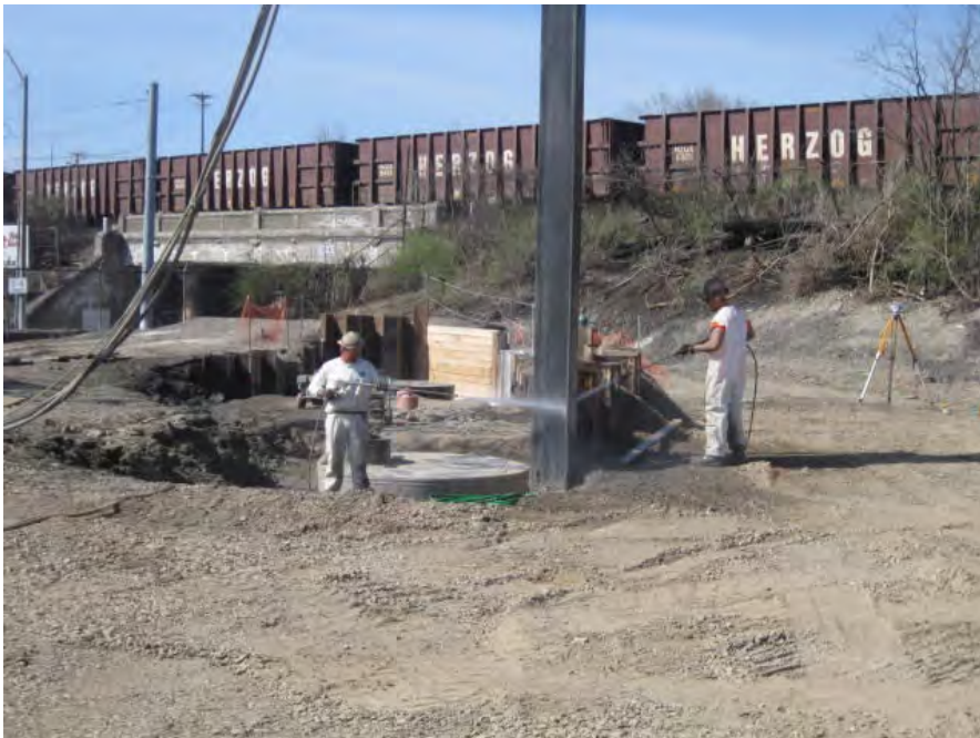
View of sheeting removal on the northern end of the site.
