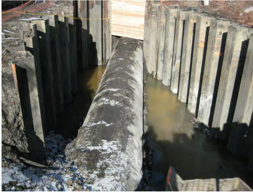
View of the north end of the Phase Two area after soil has been removed and lagging was installed.
