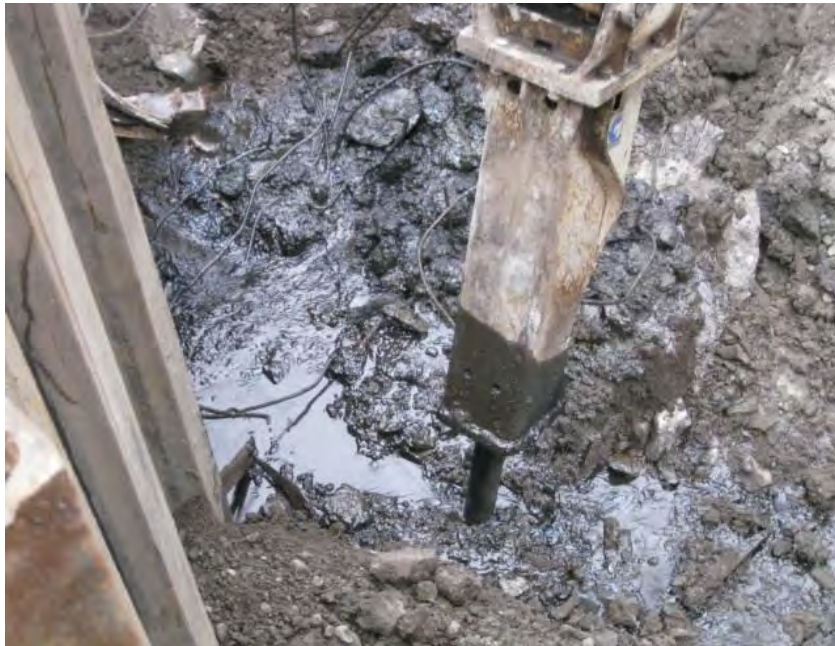
View of the removal of the concrete pipe chase near MH-1 today showing impacted material from inside the pipe chase.
