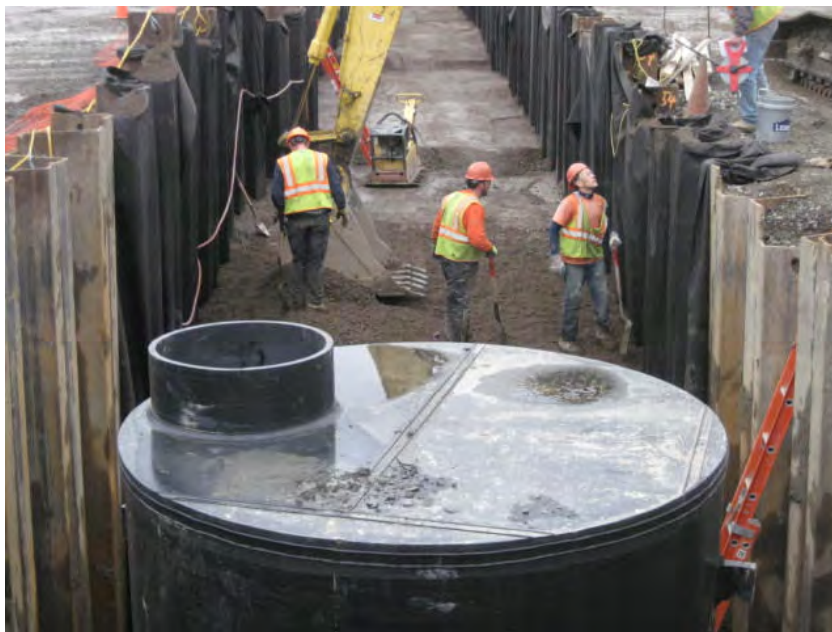
View of backfill being placed on top of the HDPE pipe.
