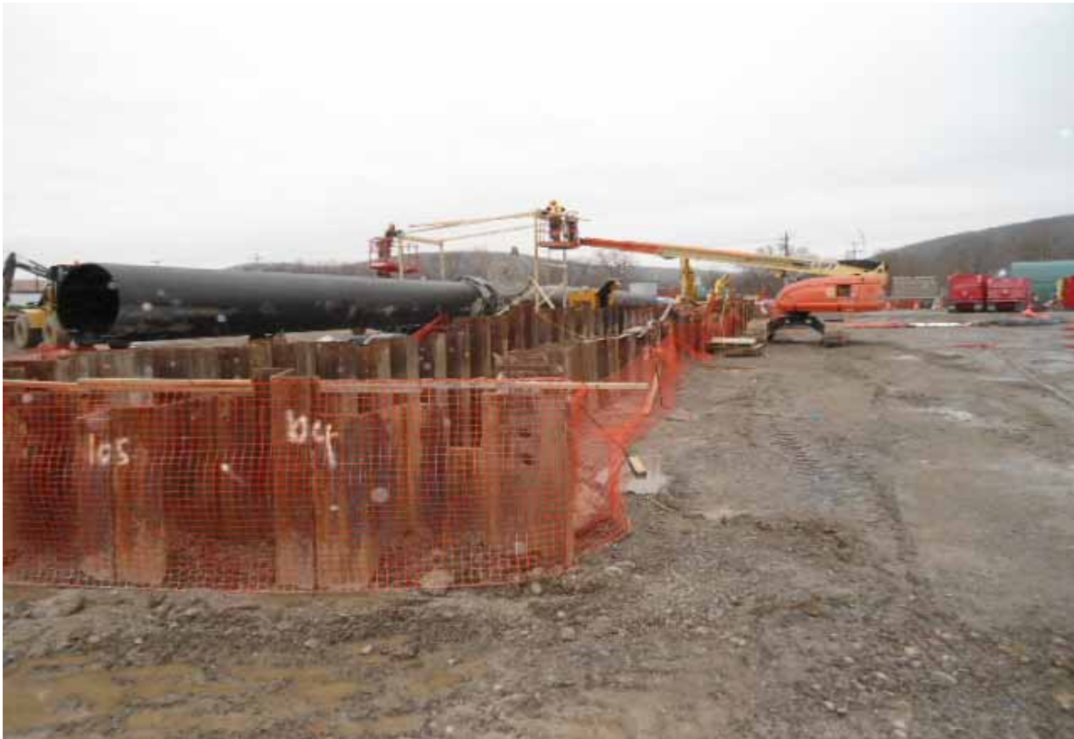
Photo #25 (2011.12.28): Facing south. Vari-Tech butt-fusing a section of HDPE and constructing a temporary structure.
