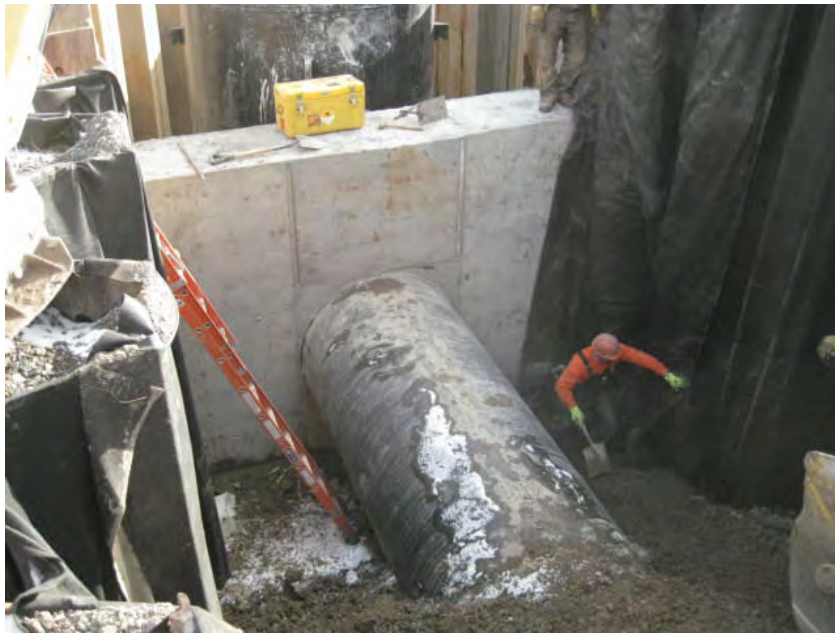
View of concrete collar at MH-1B.
