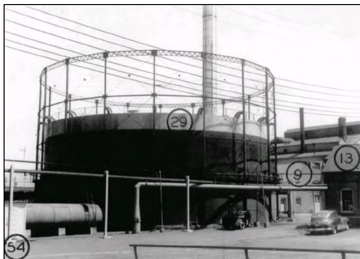
Figure 7.4 Former No. 2 gas holder.
