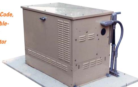
Typical stationary natural-gas fired generator
