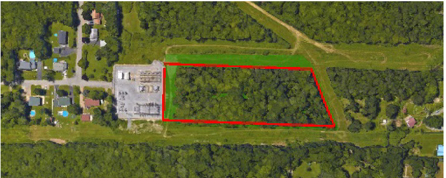
Proposed expansion at Big Tree Substation in Orchard Park.
